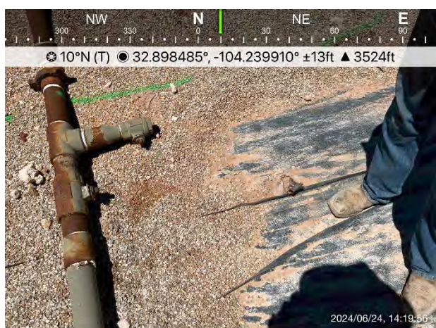
Figure 5. Hole in the liner (CS-01)
