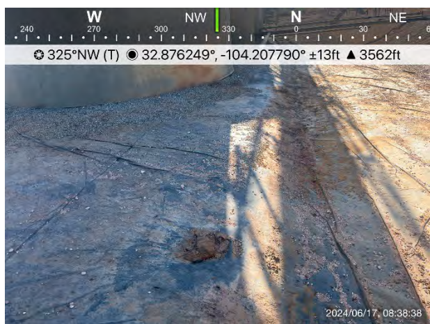
Figure 5. Hole in the liner (CS-01)
