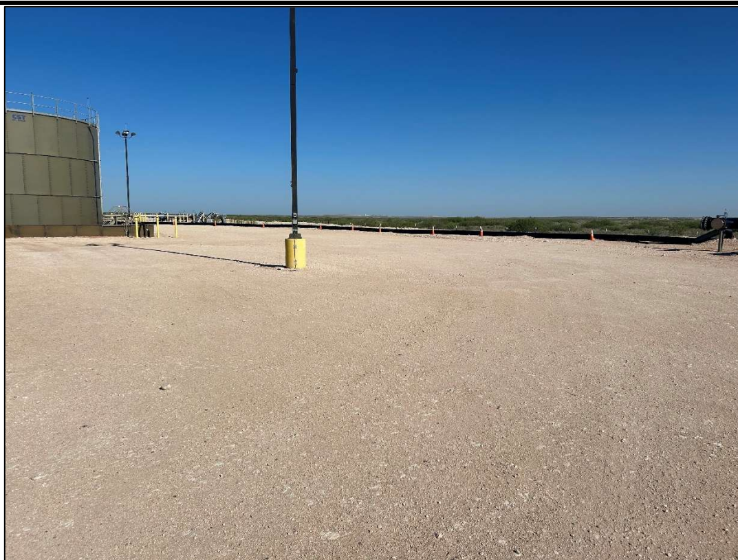
PHOTO 12: View of the remediated area facing northwest. 6/27/2024
