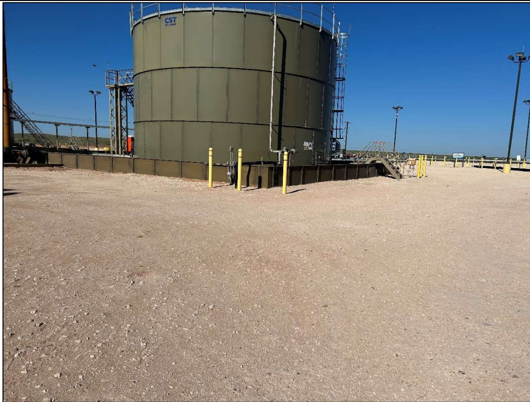
PHOTO 17: View of the remediated area facing southwest. 6/27/2024
