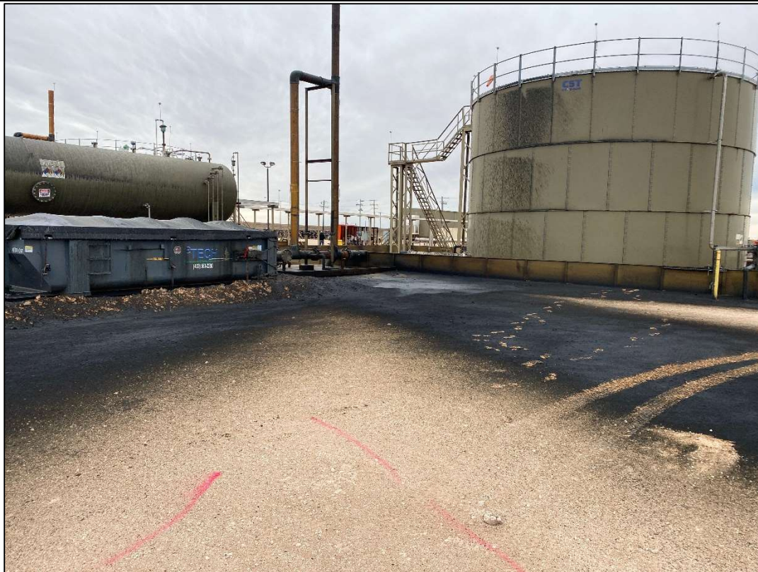
PHOTO 1: View of the impacted area facing southwest. 2/09/24
