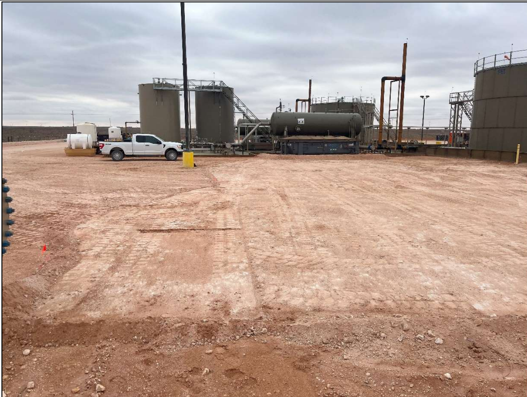
PHOTO 6: View of the excavated area facing southeast. 2/29/24
