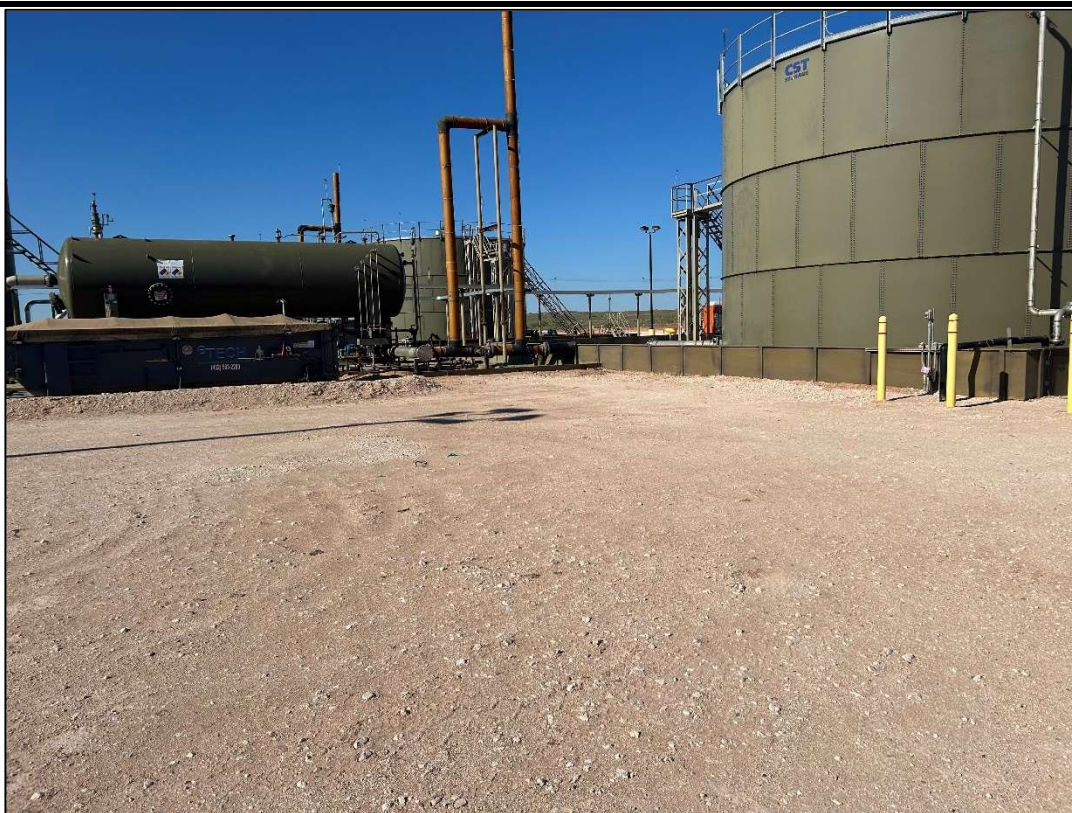
PHOTO 16: View of the remediated area facing south by southwest. 6/27/2024
