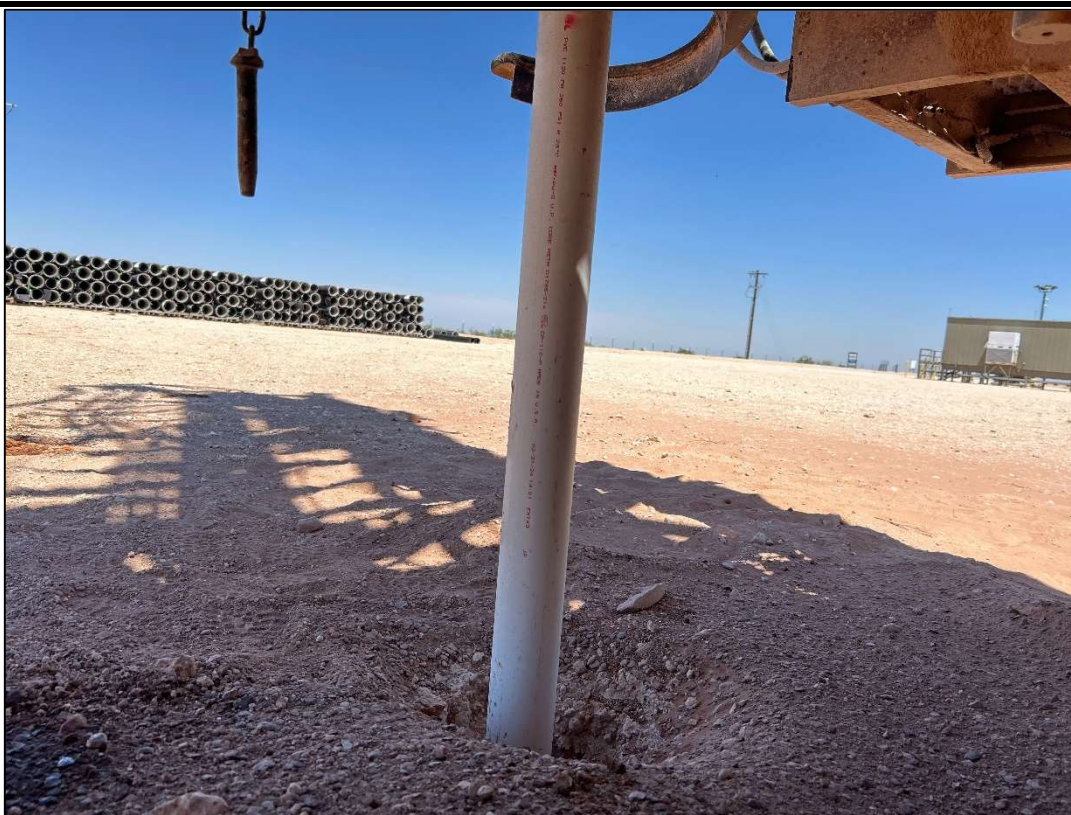
PHOTO 10: View of the temporary monitoring well facing northwest. 6/14/24
