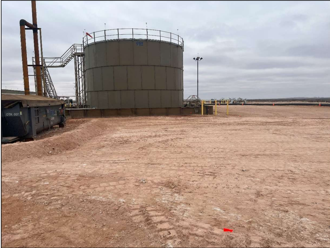
PHOTO 7: View of the south end of the excavated area facing west. 2/29/24
