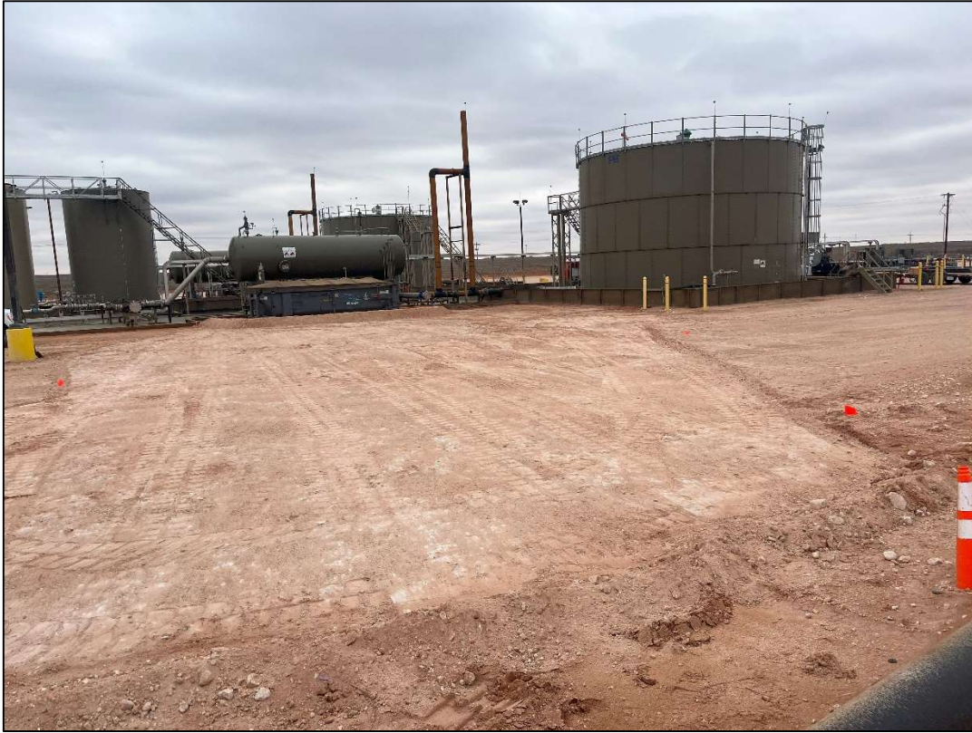
PHOTO 5: View of the excavated area facing southwest. 2/29/24
