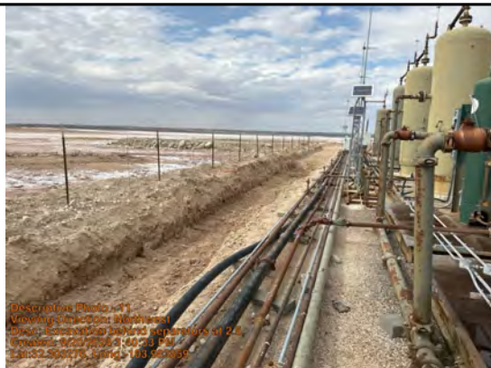
Excavation behind separators at 2.5'
