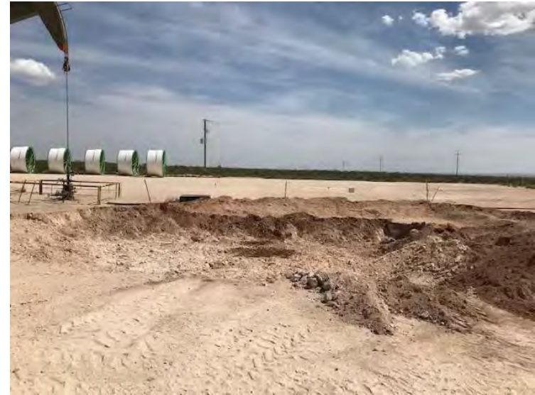
Photograph 6: View of excavation facing south (2RP-3937).
