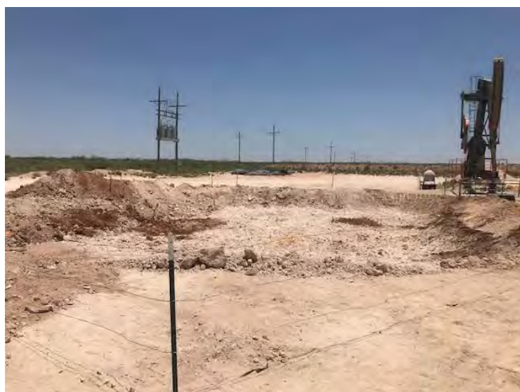
Photograph 11: View of excavation facing east (2RP-3937).
