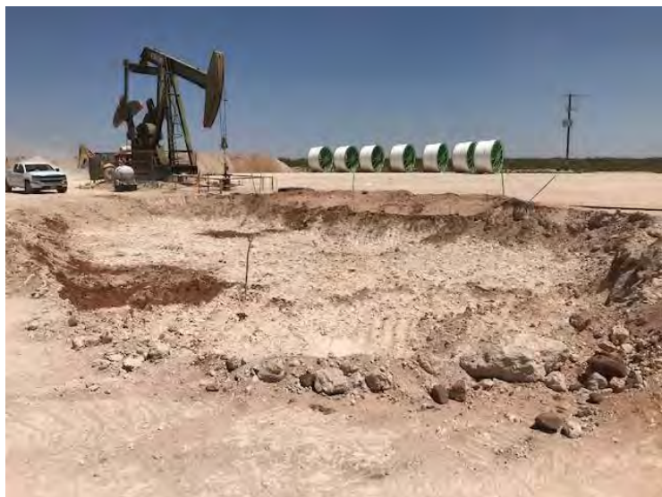
Photograph 9: View of excavation facing southeast (2RP-3937).
