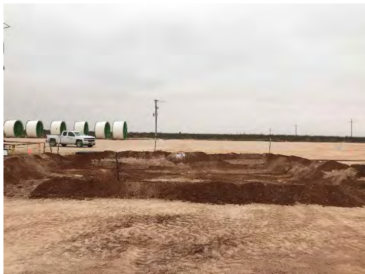
Photograph 3: View of excavation facing south (2RP-3937).
