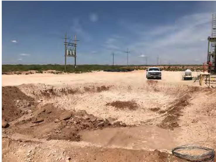
Photograph 5: View of excavation facing east (2RP-3937).
