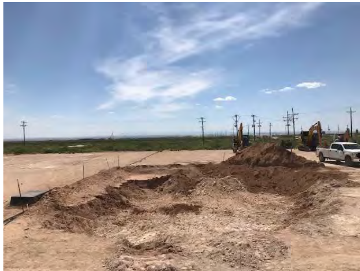
Photograph 7: View of excavation facing west (2RP-3937).
