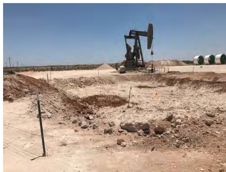
Photograph 12: View of excavation facing southeast (2RP-3937).
