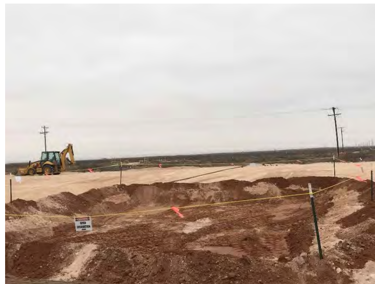
Photograph 4: View of excavation facing west (2RP-3937).
