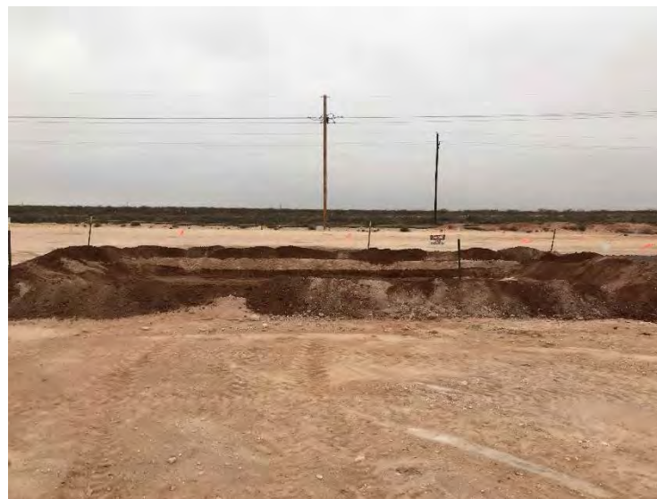
Photograph 2: View of excavation facing north (2RP-3937).
