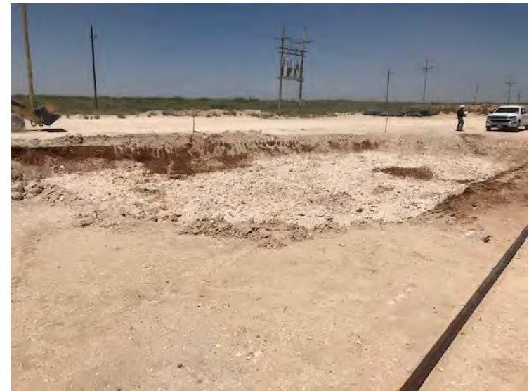
Photograph 8: View of excavation facing northeast (2RP-3937).
