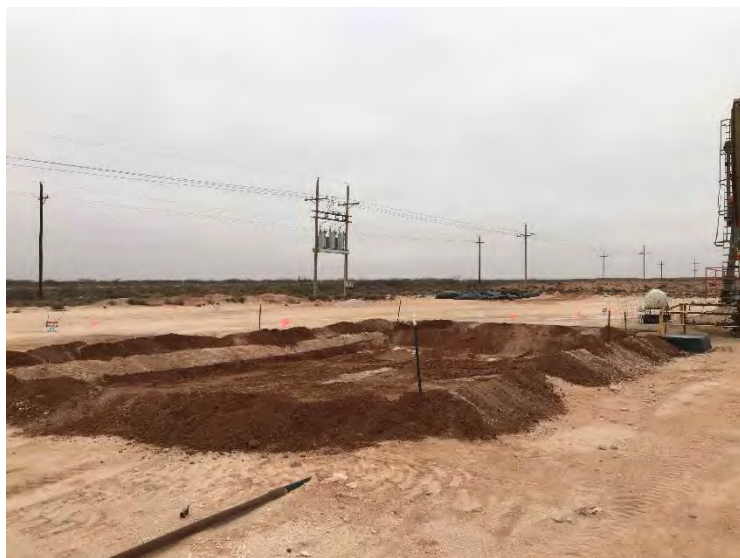
Photograph 1: View of excavation facing east (2RP-3937).
