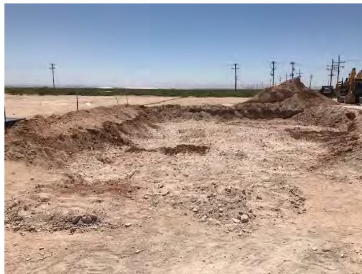
Photograph 10: View of excavation facing west (2RP-3937).
