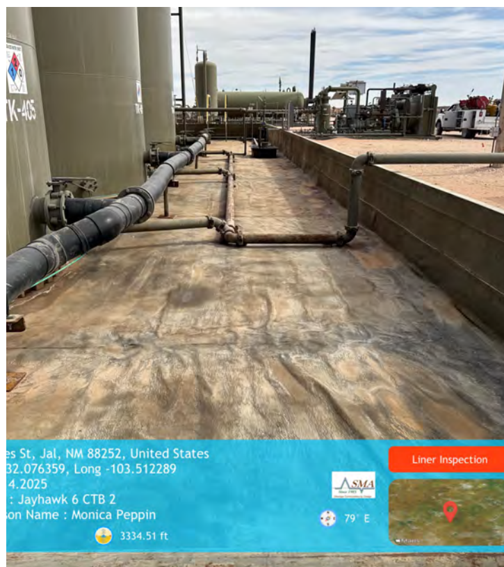
Photograph #20: Liner on north side of tanks
