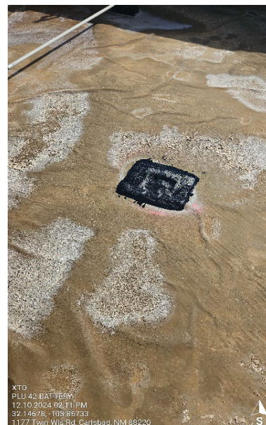
Photograph: 4 Date: 12/10/2024 Description: Patched liner tear View: South
