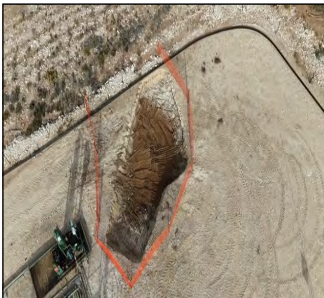
Photograph taken during excavation.
