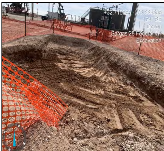
Photograph taken during excavation facing southeast.
