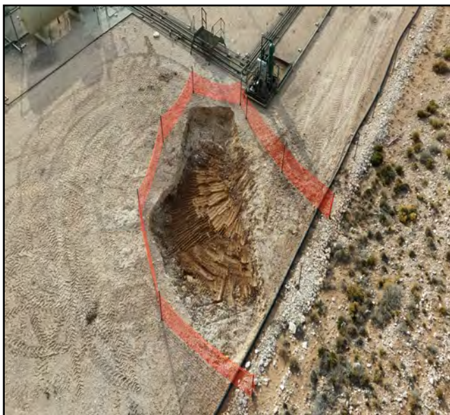
Photograph taken during excavation.
