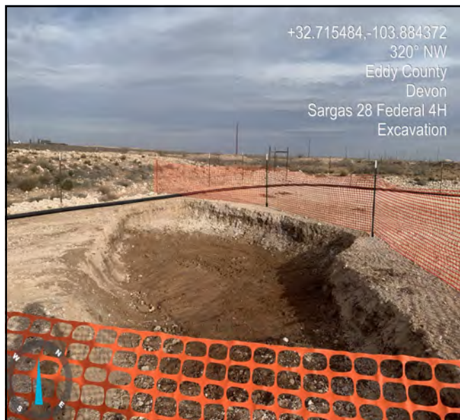
Photograph taken during excavation facing northwest.
