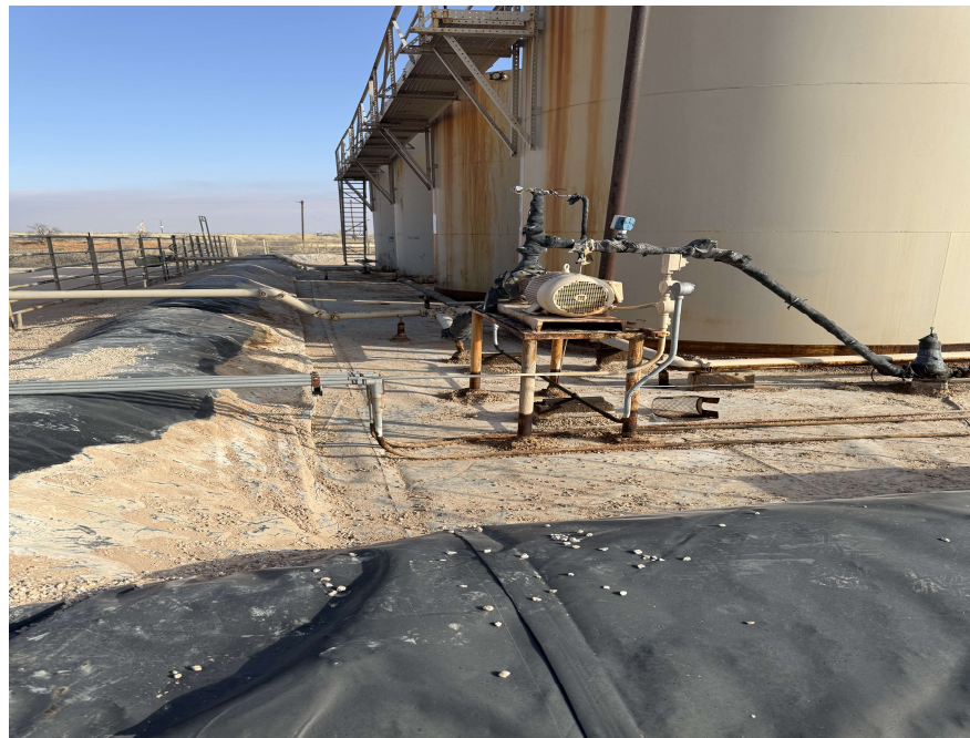
Photograph 2 (dated 2/11/2025) – View looking N at west side secondary containment with the liner exposed.
