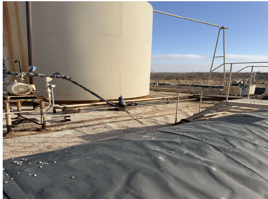
Photograph 4 (dated 2/11/2025) – View looking SE at the exposed liner within secondary containment.
