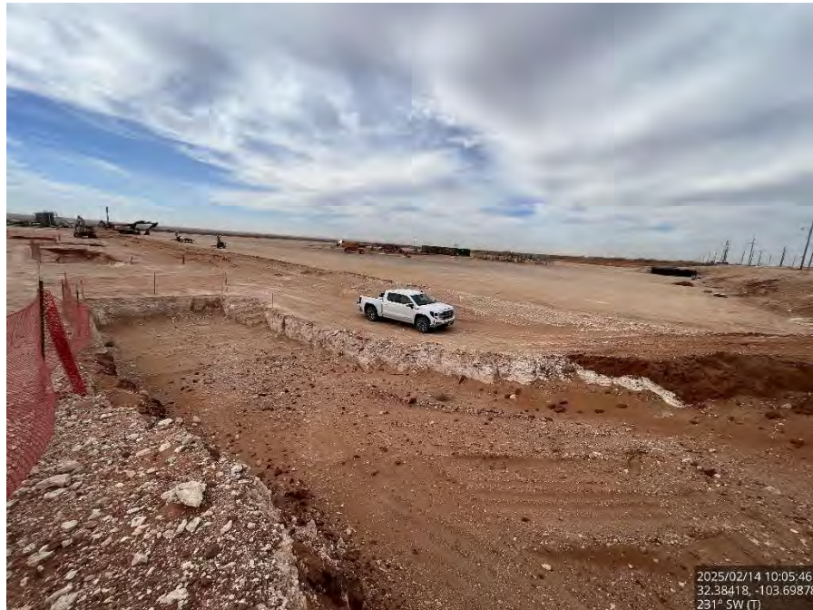
Excavated Area #4 on the pad, viewing southwest.
