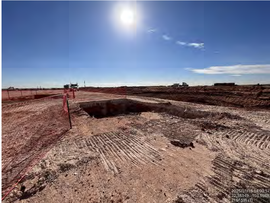
Excavated Area #2 on the pad, viewing southwest.
