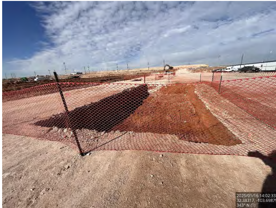
Excavated Area #1 on the pad, viewing north.
