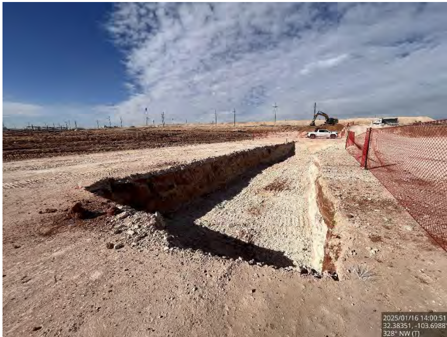
Excavated Area #3 on the pad, viewing northwest.
