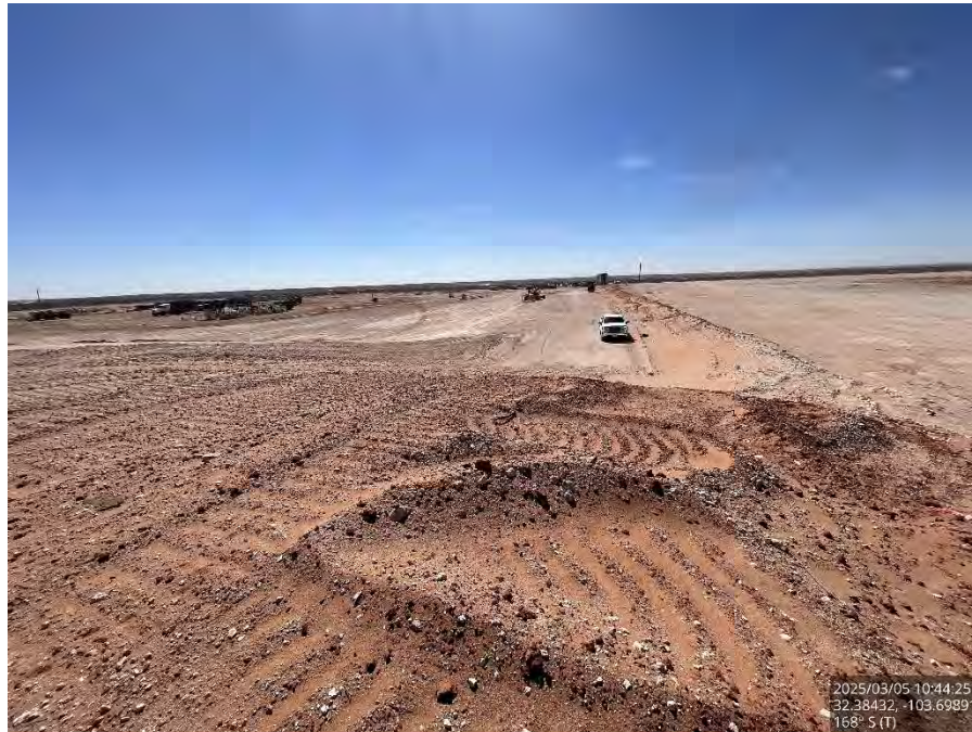
Backfilled area on the pad, viewing south.
