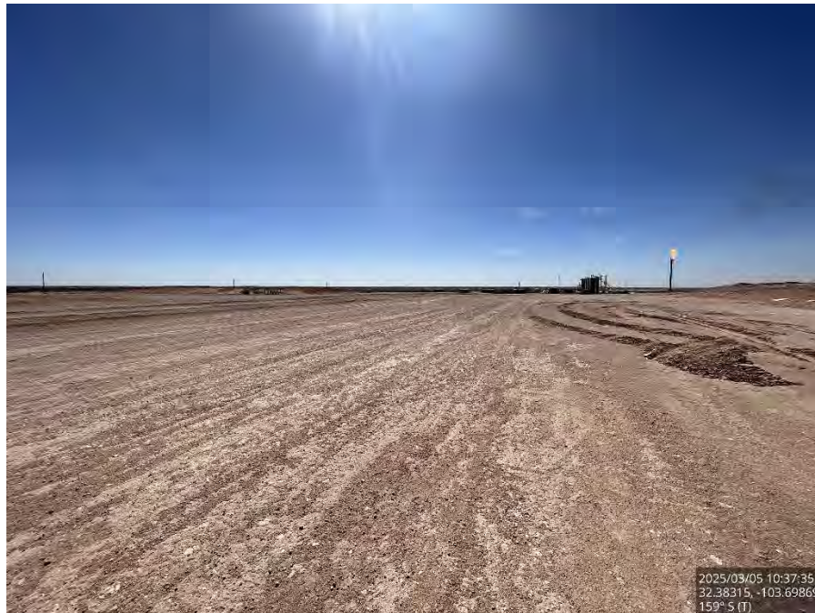
Backfilled area on the pad, viewing south.
