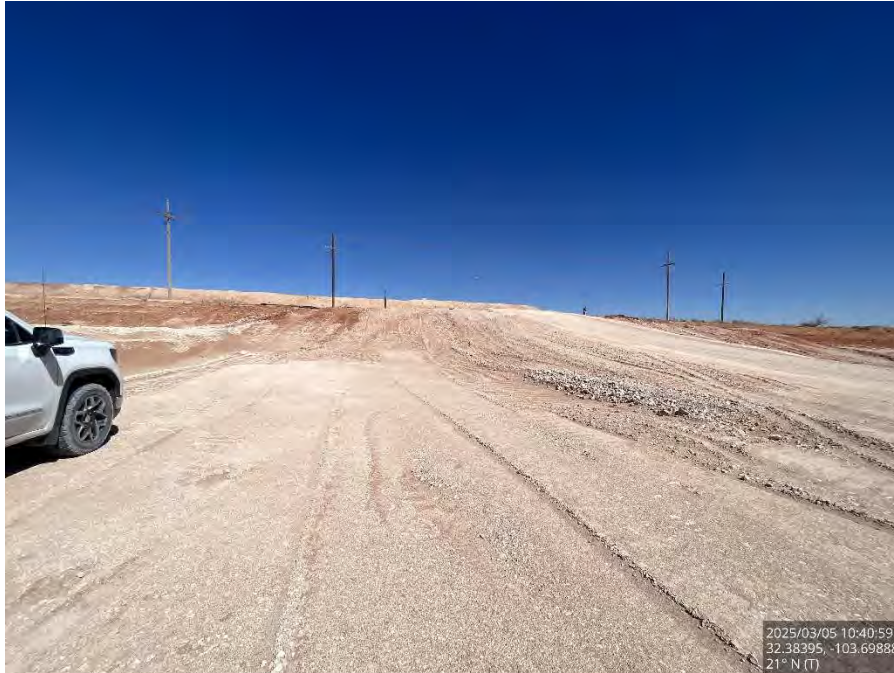
Backfilled area on the pad, viewing north.
