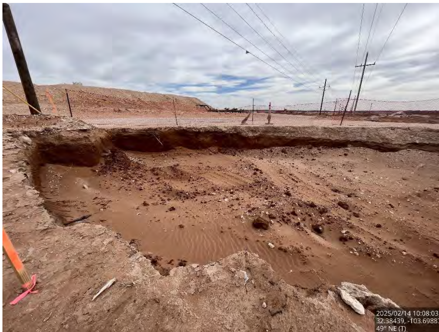
Excavated Area #4 on the pad, viewing northeast.
