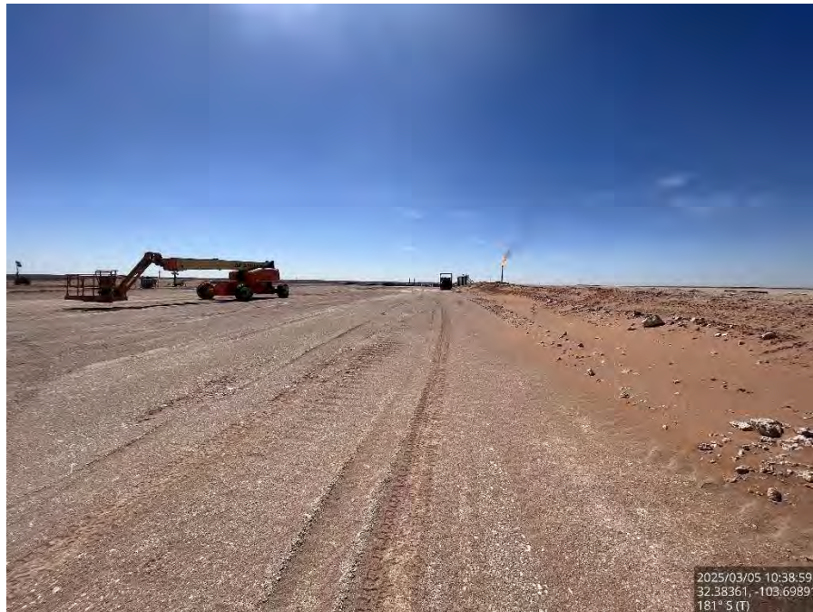
Backfilled area on the pad, viewing south.
