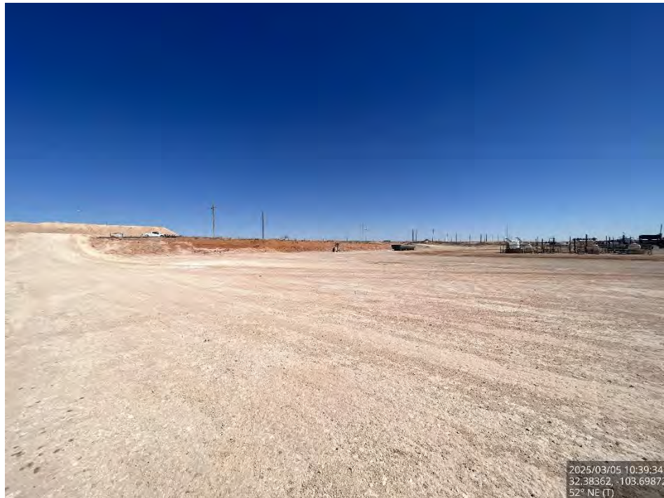
Backfilled area on the pad, viewing northeast.
