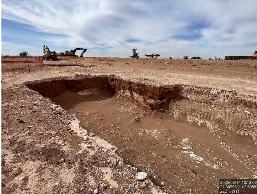
Excavated Area #3 on the pad, viewing southwest.
