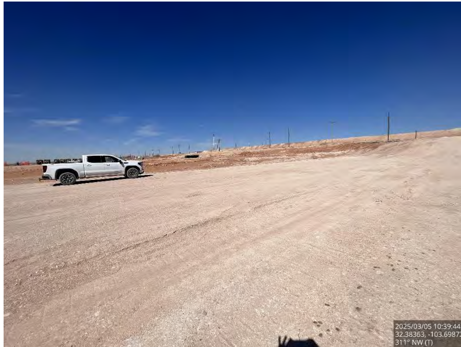
Backfilled area on the pad, viewing northwest.
