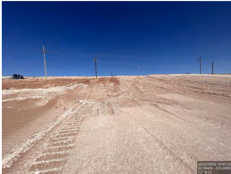
Backfilled area on the pad, viewing north.
