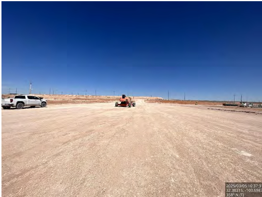
Backfilled area on the pad, viewing north.
