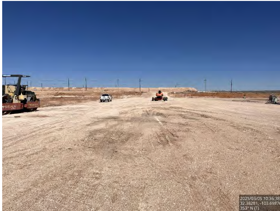
Backfilled area on the pad, viewing west.
