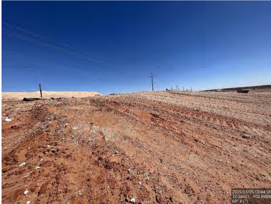
Backfilled area on the pad, viewing east.
