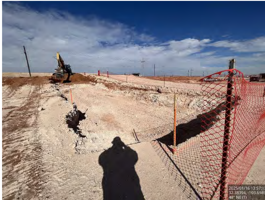
Excavated Area #4 on the pad, viewing northeast.
