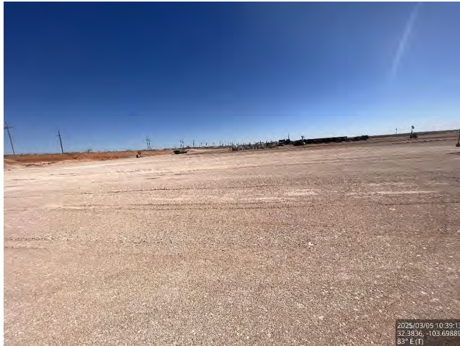
Backfilled area on the pad, viewing east.
