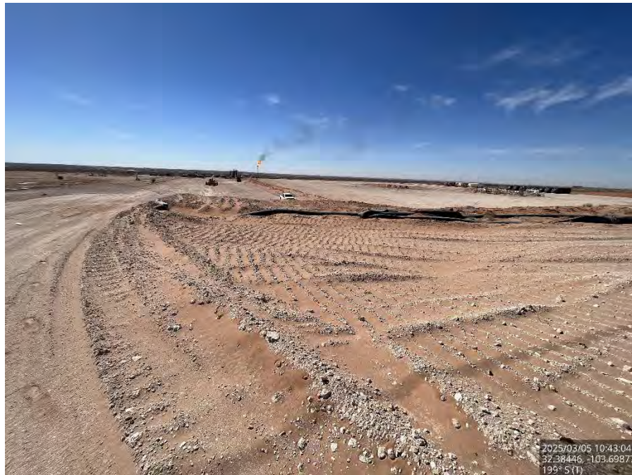
Backfilled area on the pad, viewing south.
