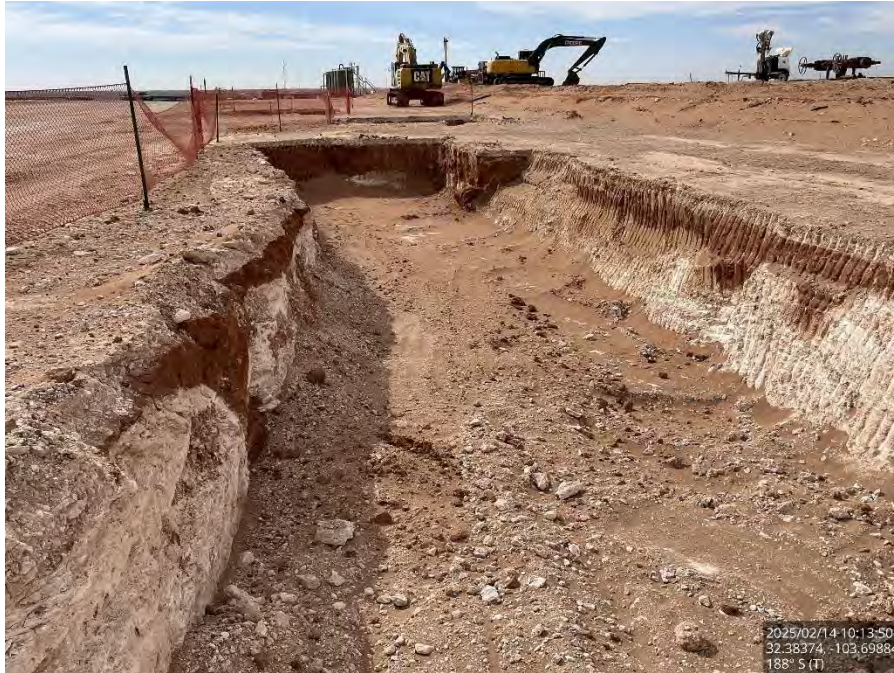
Excavated Area #3 on the pad, viewing south.
