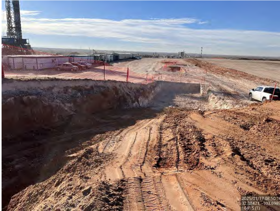
Excavated Area #4 on the pad, viewing south.
