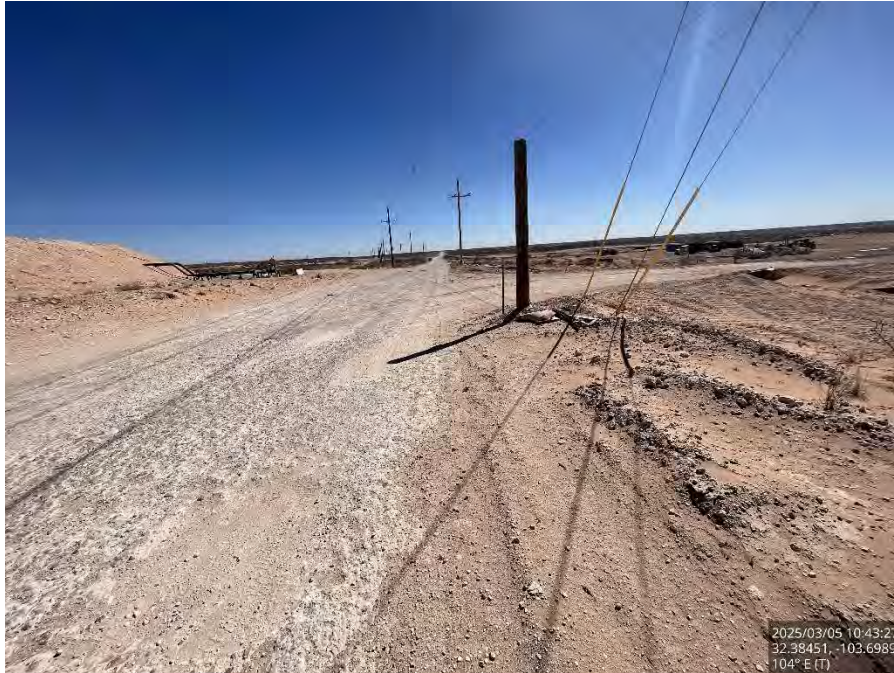
Backfilled area on the pad, viewing east.
