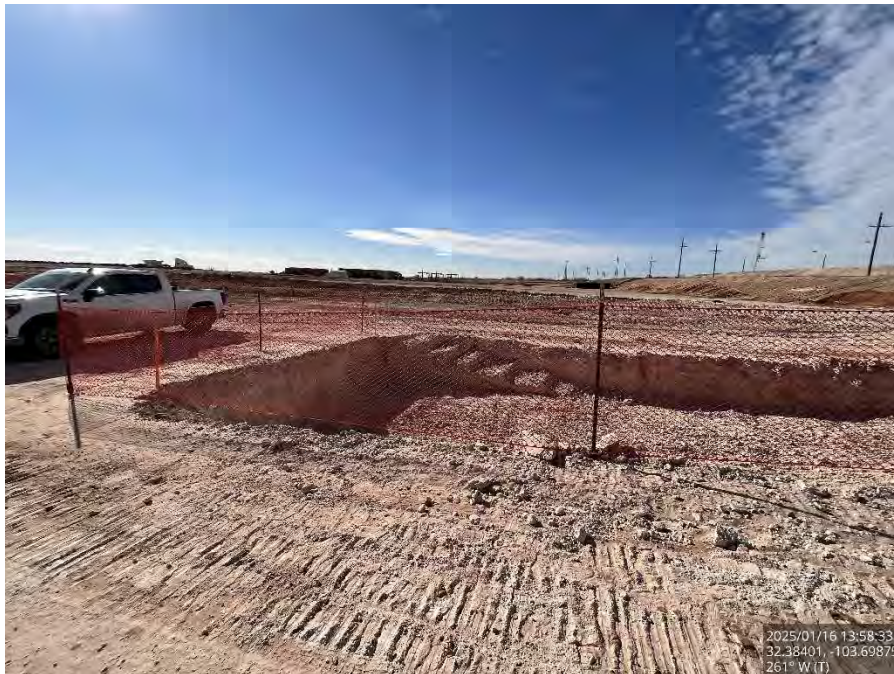
Excavated Area #3 on the pad, viewing west.
