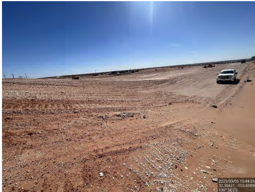
Backfilled area on the pad, viewing southeast.
