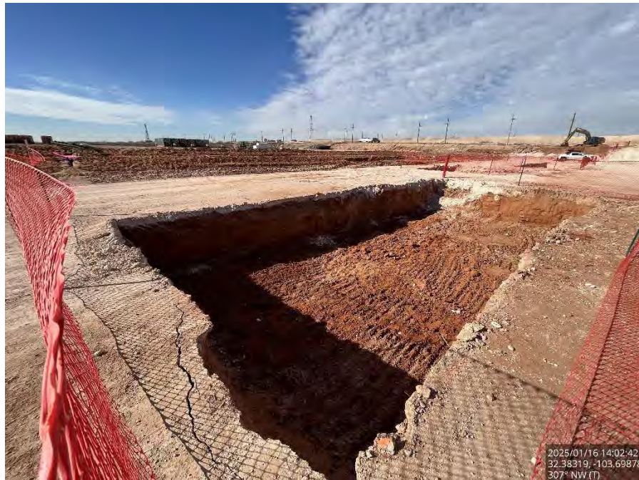
Excavated Area #1 on the pad, viewing northwest.
