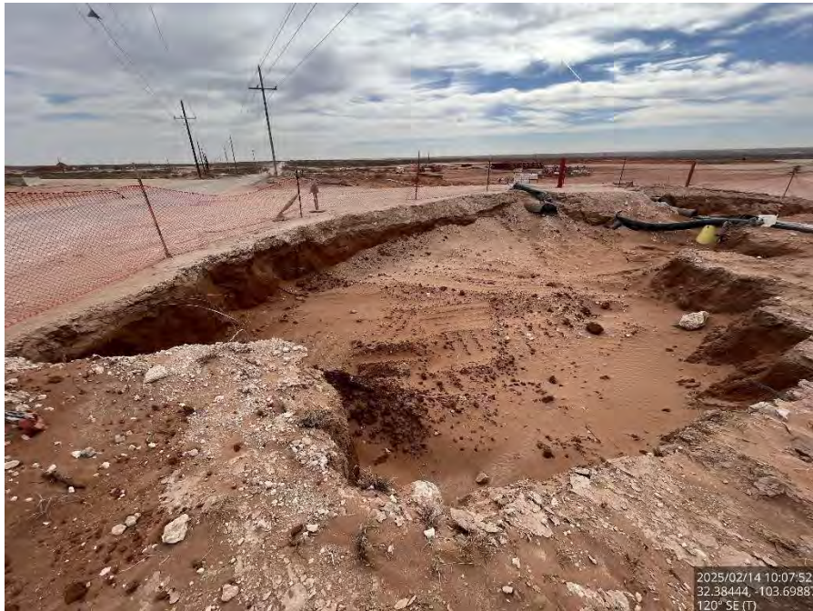
Excavated Area #4 on the pad, viewing southeast.
