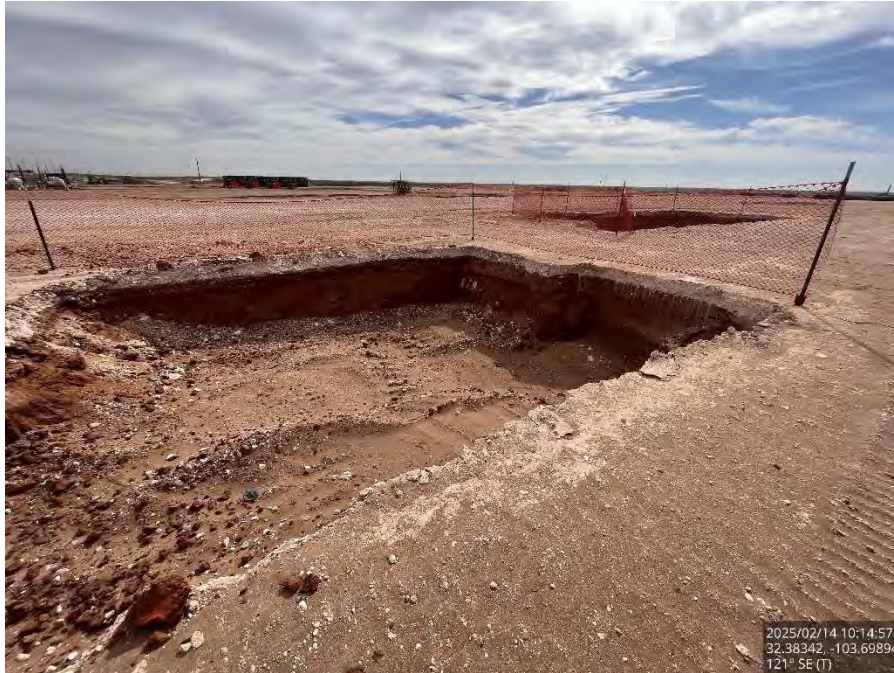
Excavated Area #2 on the pad, viewing southeast.
