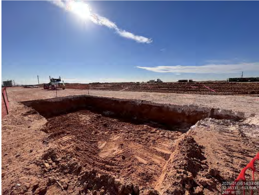
Excavated Area #1 on the pad, viewing west.
