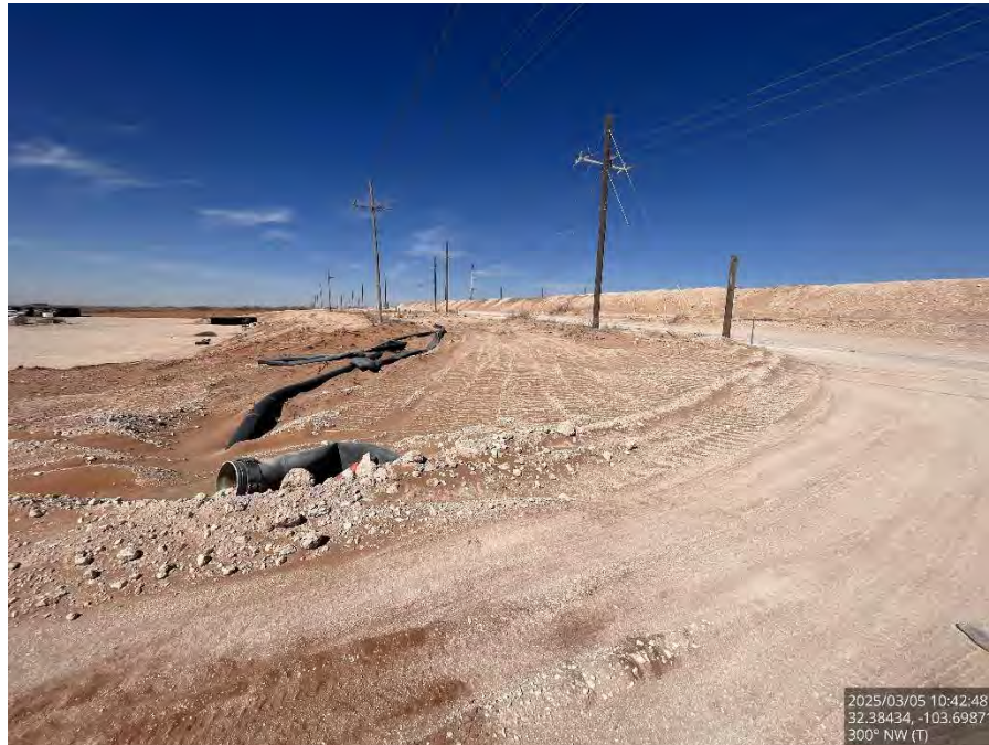
Backfilled area on the pad, viewing northwest.
