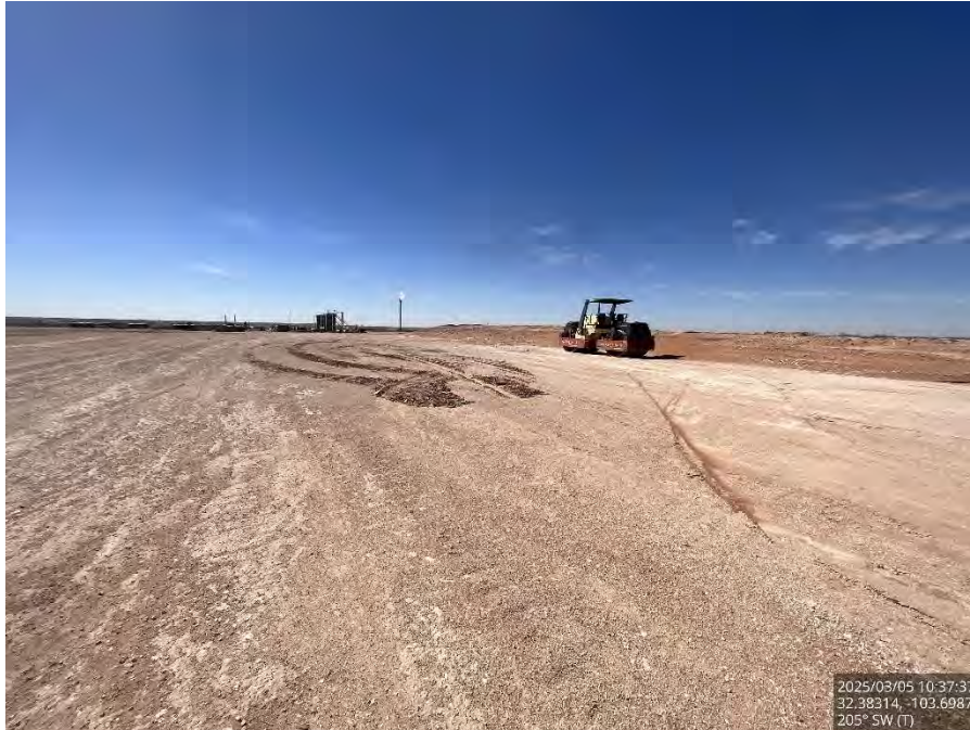
Backfilled area on the pad, viewing southwest.
