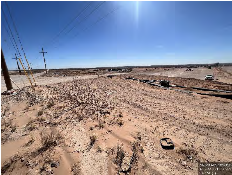
Backfilled area on the pad, viewing southeast.
