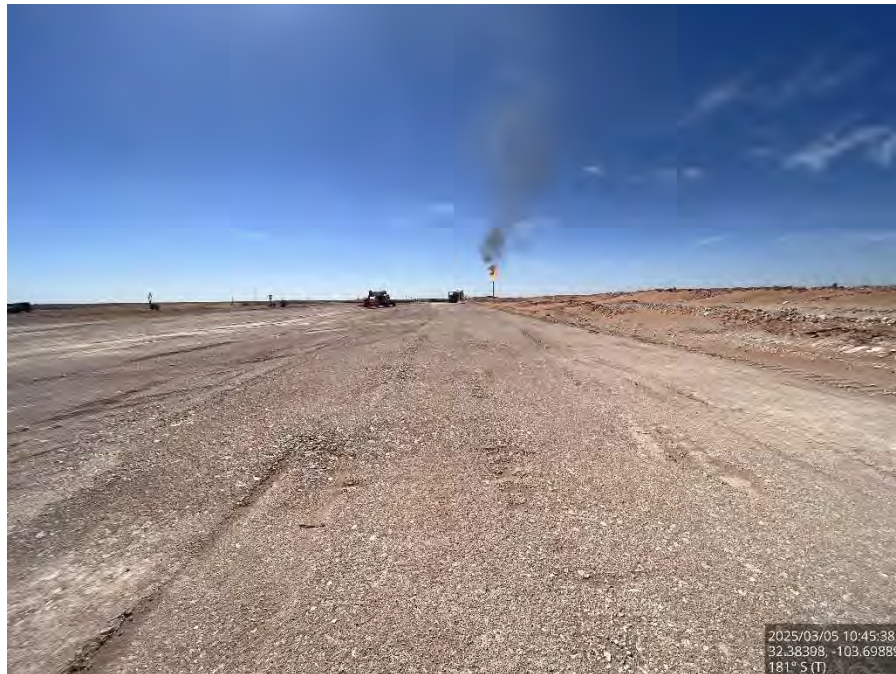
Backfilled area on the pad, viewing south.
