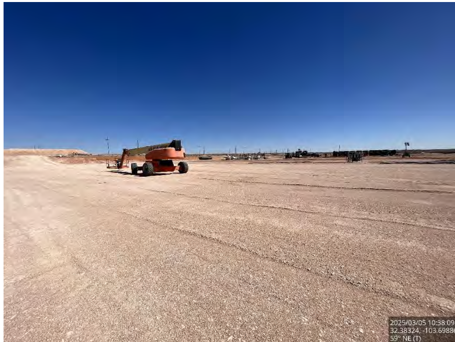
Backfilled area on the pad, viewing northeast.
