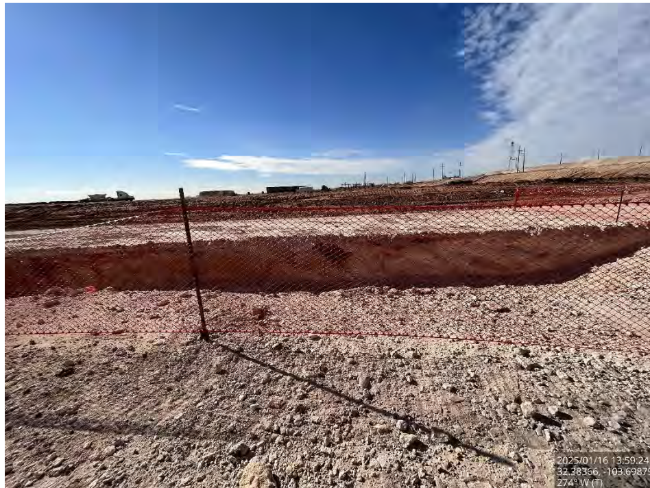
Excavated Area #3 on the pad, viewing west.
