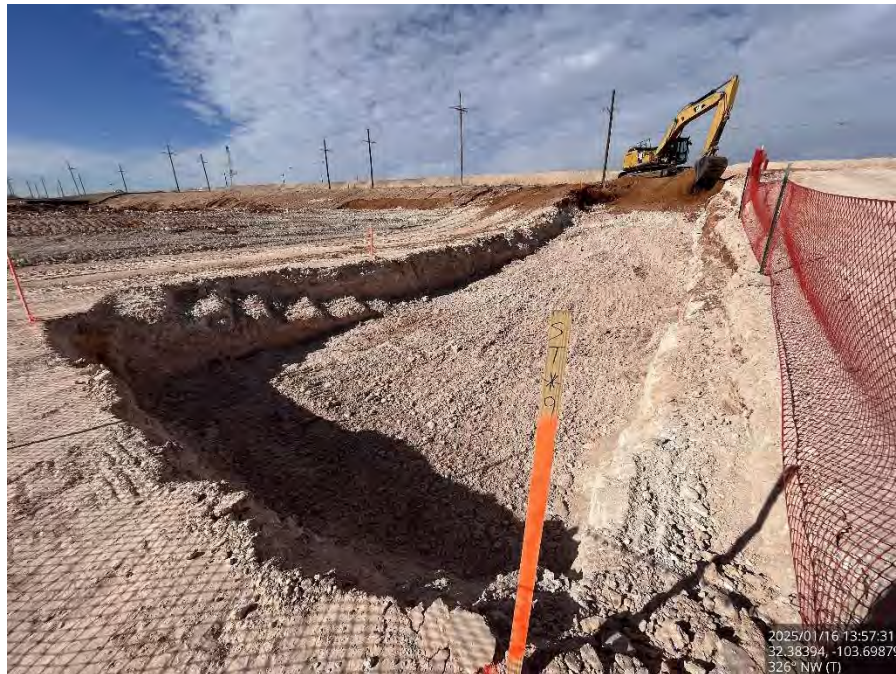
Excavated Area #4 on the pad, viewing northwest.
