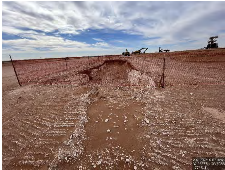
Excavated Area #3 on the pad, viewing south.
