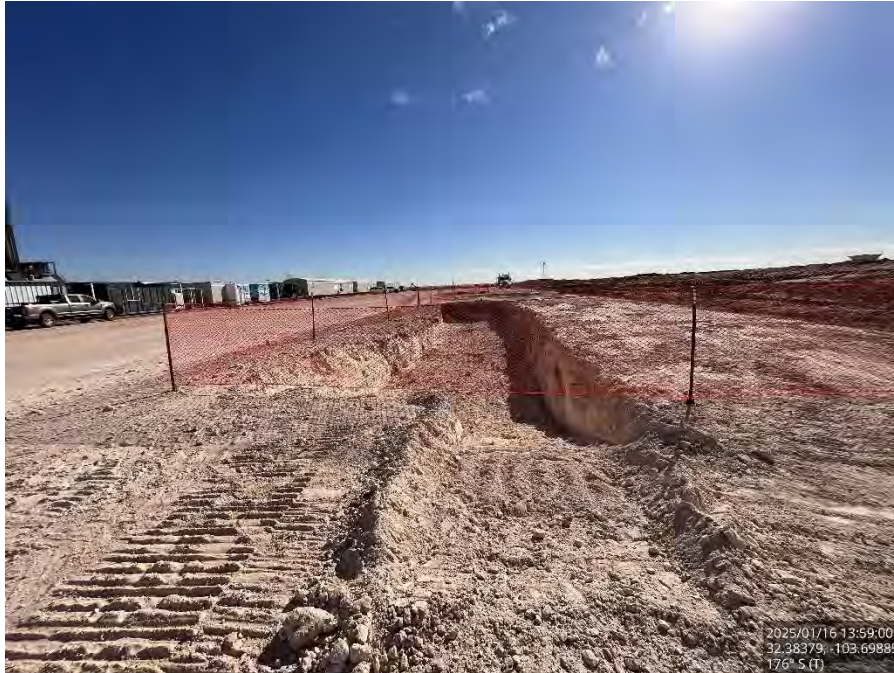
Excavated Area #3 on the pad, viewing south.
