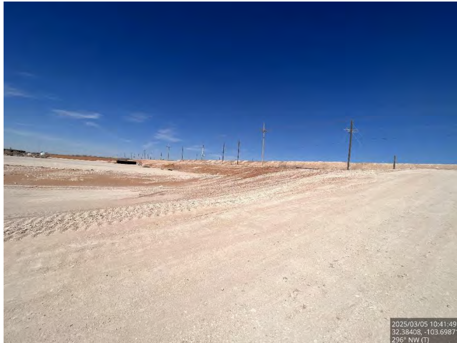
Backfilled area on the pad, viewing northwest.
