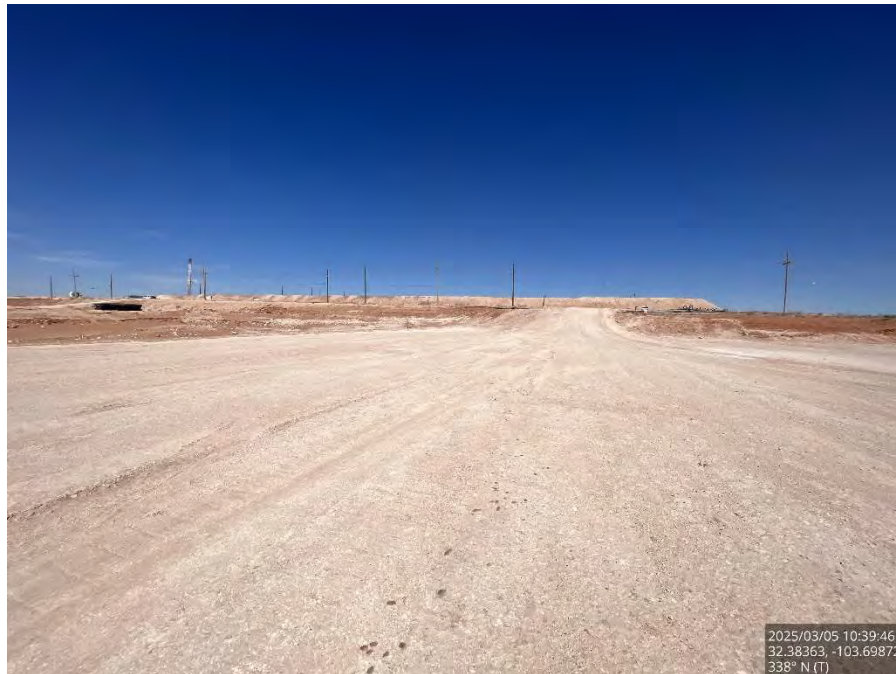
Backfilled area on the pad, viewing north.
