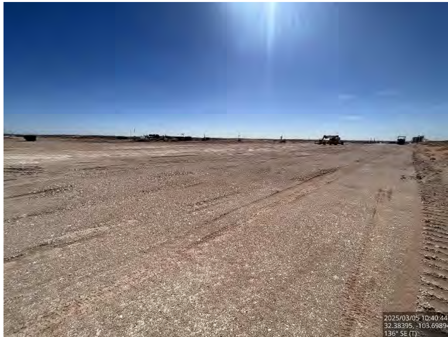
Backfilled area on the pad, viewing southeast.
