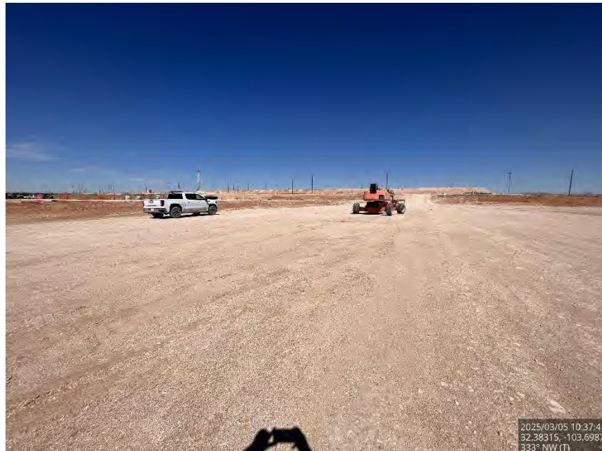
Backfilled area on the pad, viewing northwest.
