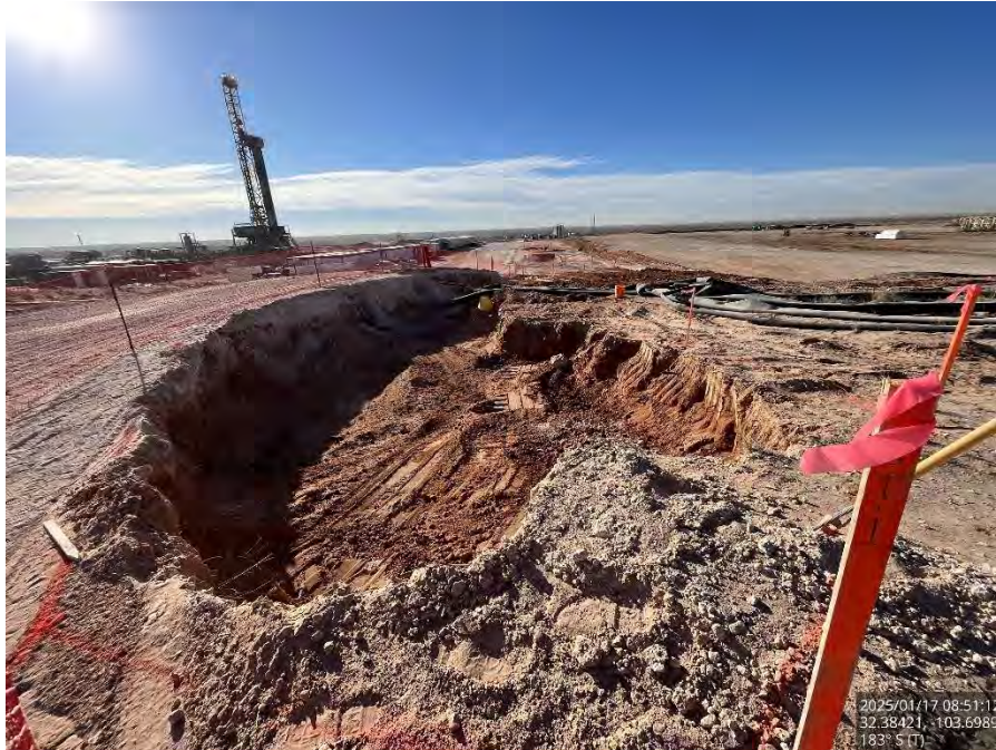
Excavated Area #4 on the pad, viewing south.
