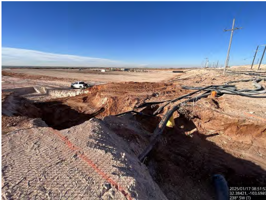
Excavated Area #4 on the pad, viewing southwest.
