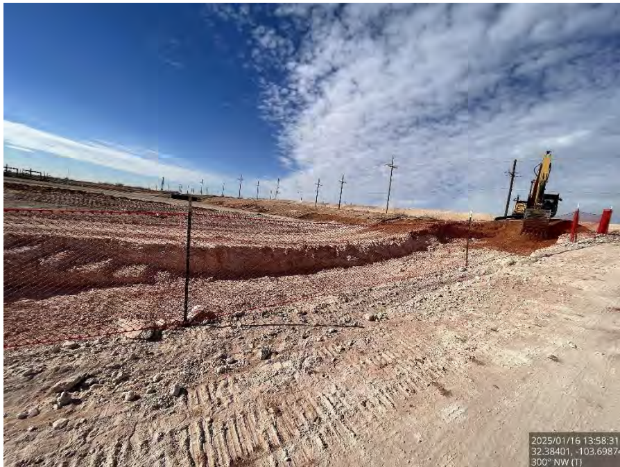
Excavated Area #4 on the pad, viewing northwest.
