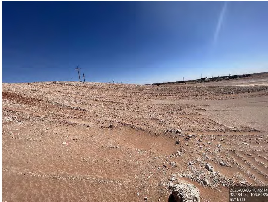
Backfilled area on the pad, viewing east.
