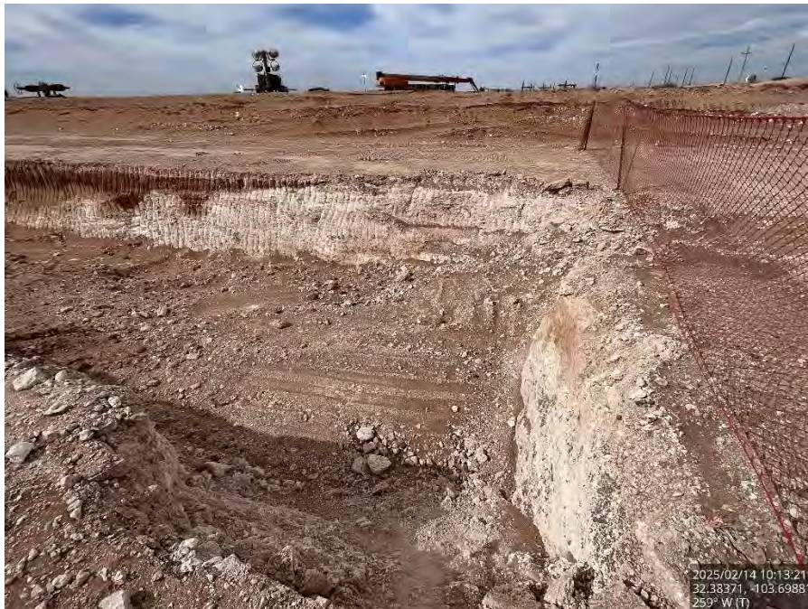
Excavated Area #3 on the pad, viewing west.
