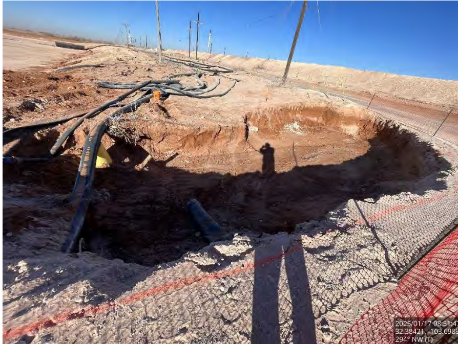
Excavated Area #4 on the pad, viewing west.
