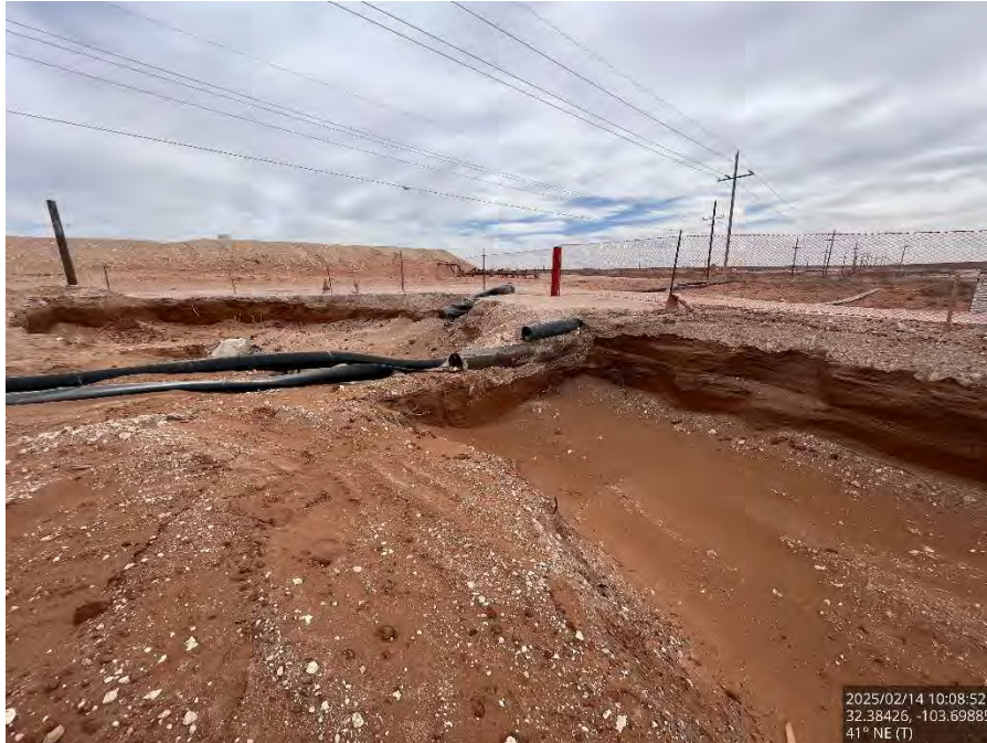
Excavated Area #4 on the pad, viewing northeast.
