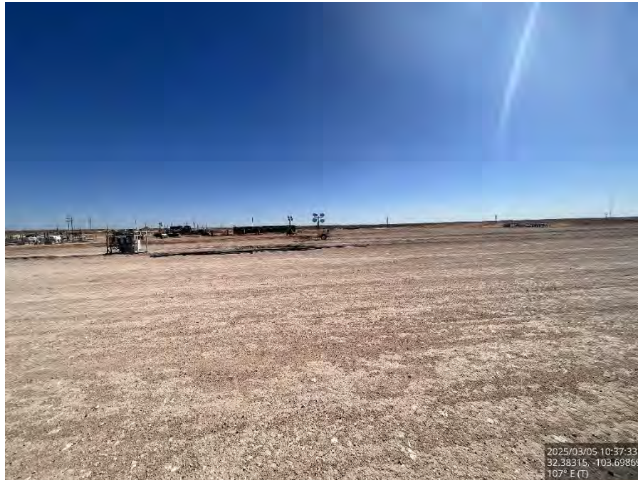
Backfilled area on the pad, viewing east.
