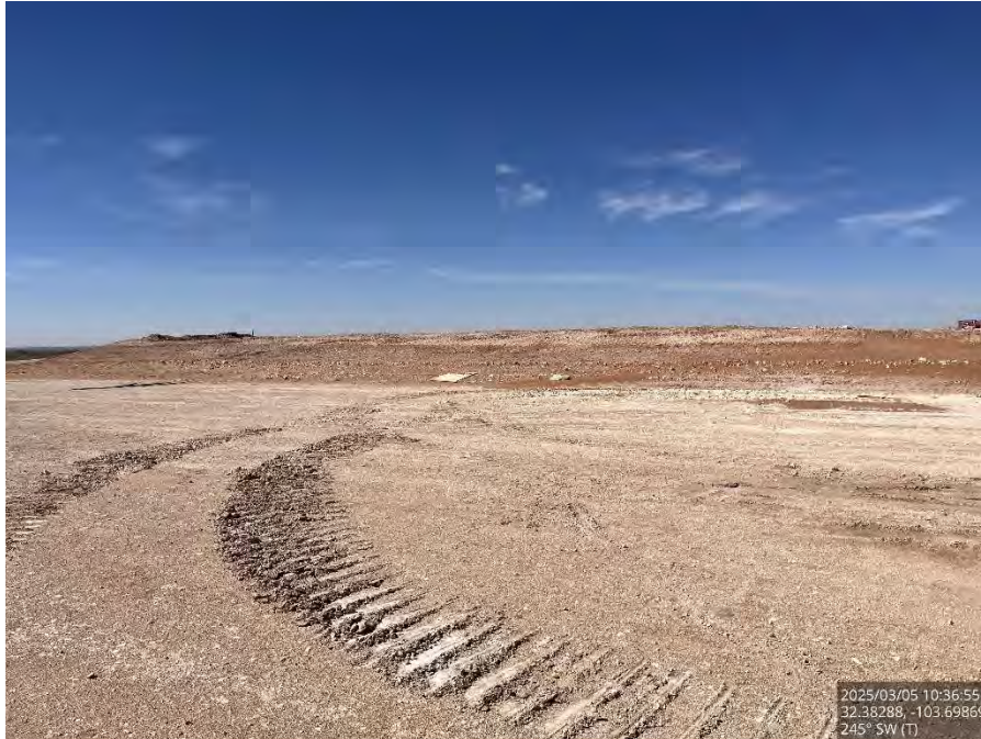
Backfilled area on the pad, viewing southwest.
