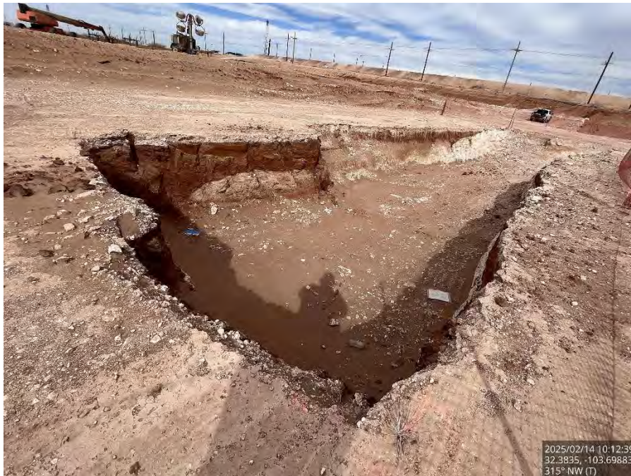
Excavated Area #3 on the pad, viewing northwest.
