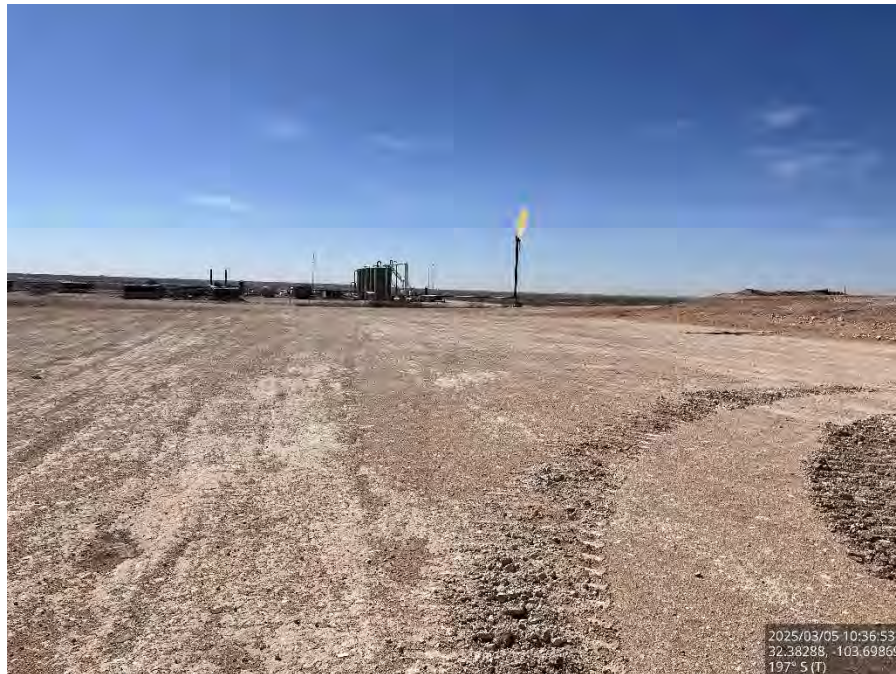
Backfilled area on the pad, viewing south.
