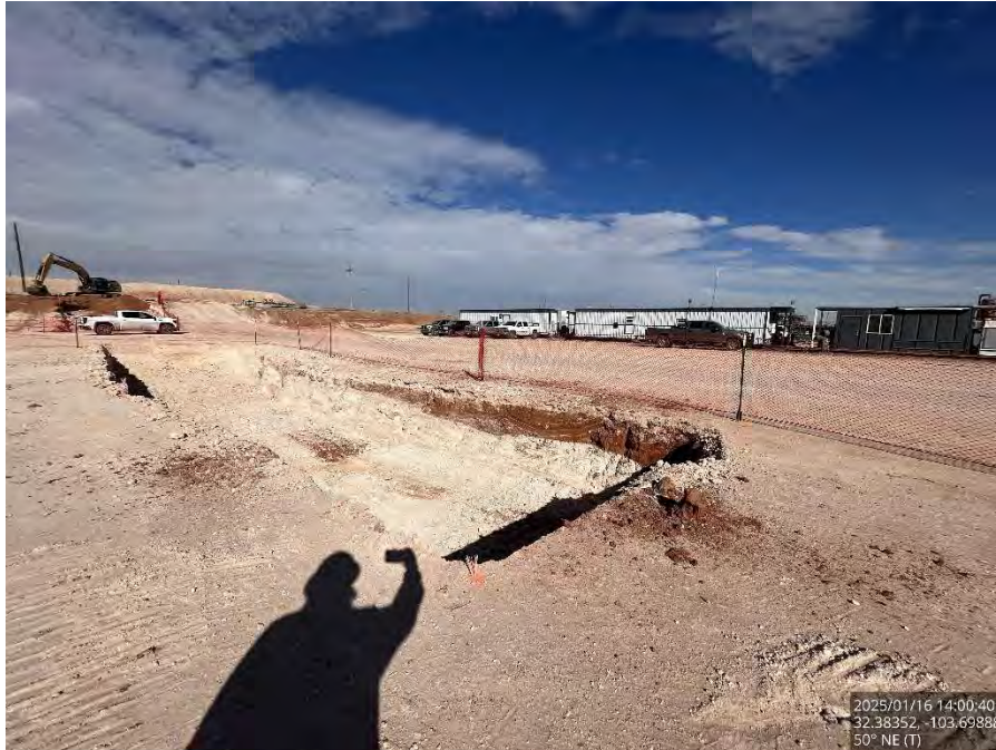
Excavated Area #3 on the pad, viewing northeast.
