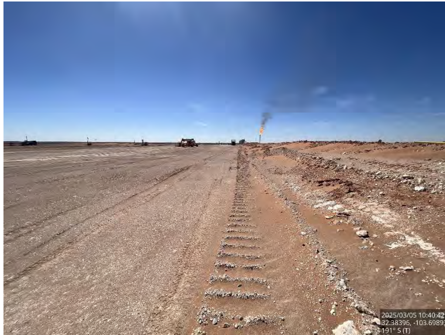
Backfilled area on the pad, viewing south.
