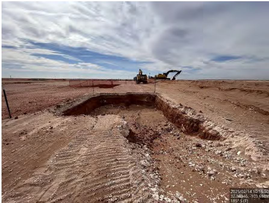
Excavated Area #2 on the pad, viewing south.
