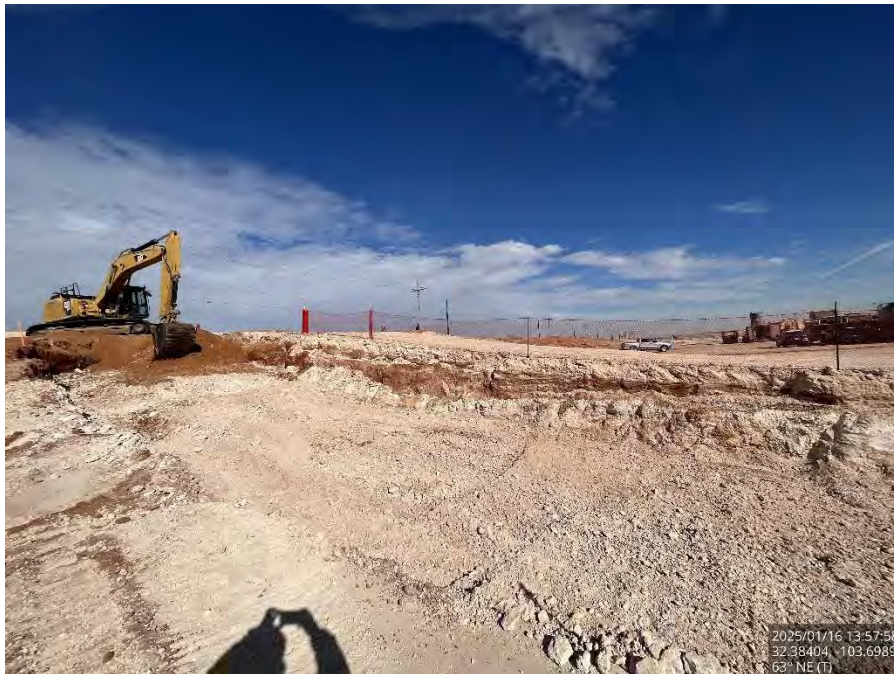
Excavated Area #4 on the pad, viewing northeast.
