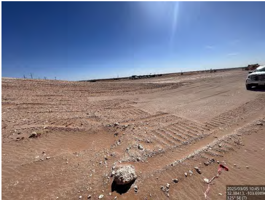
Backfilled area on the pad, viewing southeast.
