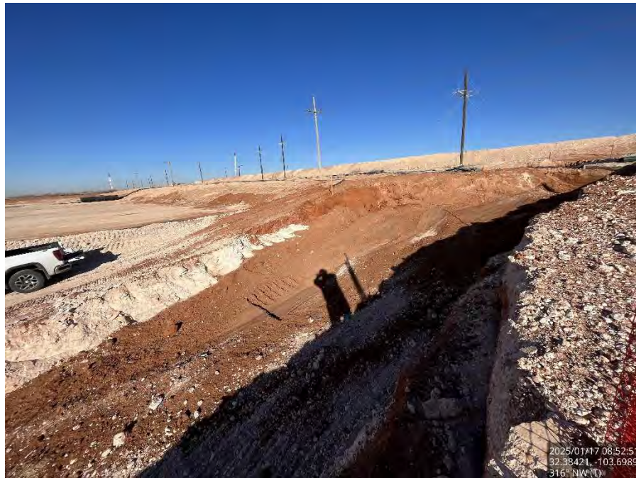
Excavated Area #4 on the pad, viewing northwest.
