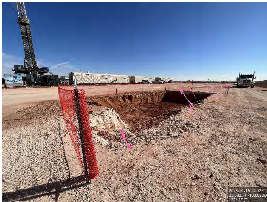
Excavated Area #1 on the pad, viewing southeast.
