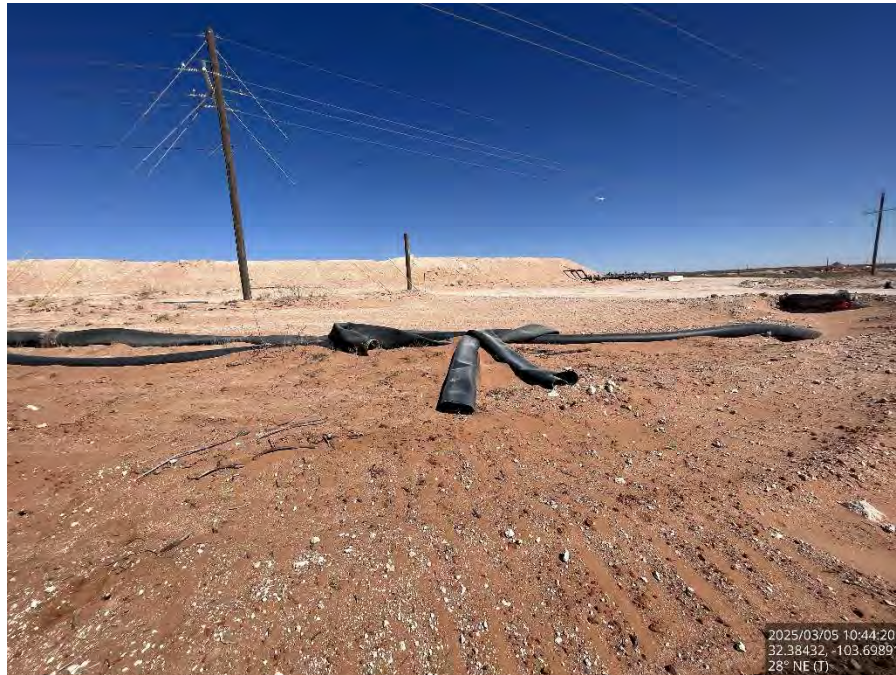
Backfilled area on the pad, viewing northeast.
