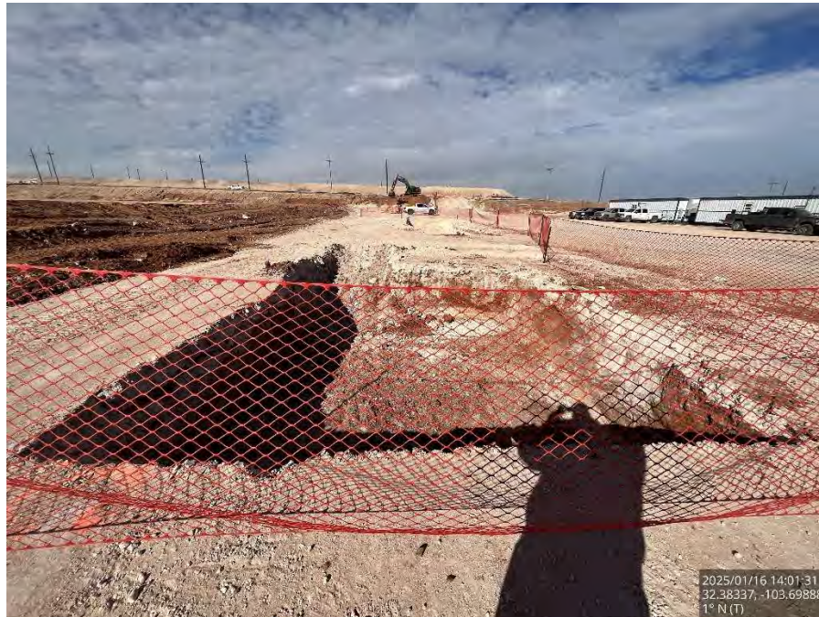
Excavated Area #2 on the pad, viewing north.
