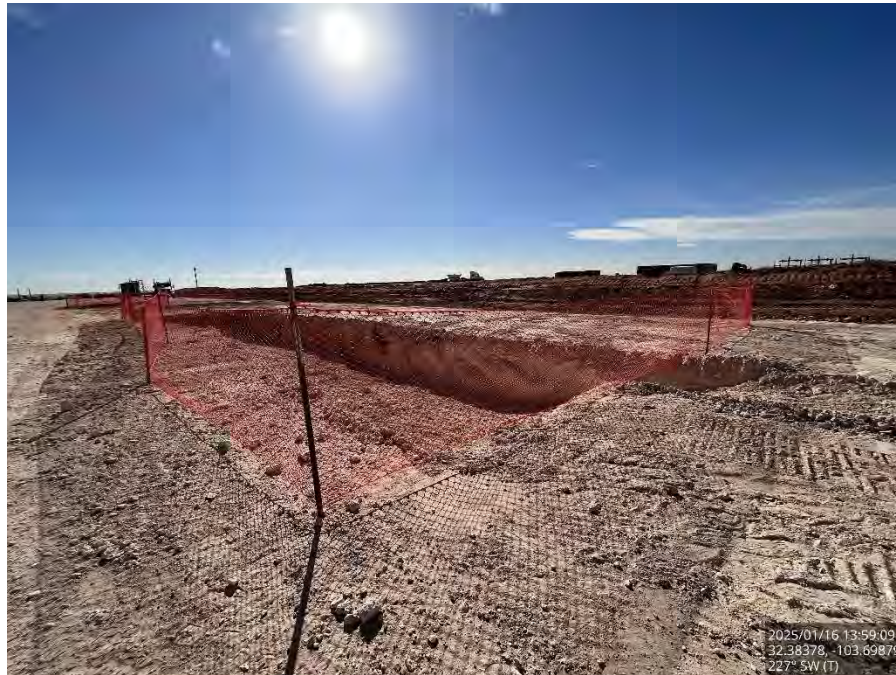
Excavated Area #3 on the pad, viewing southwest.
