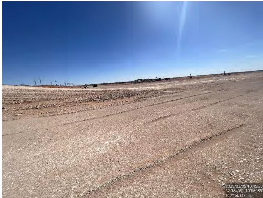
Backfilled area on the pad, viewing southeast.
