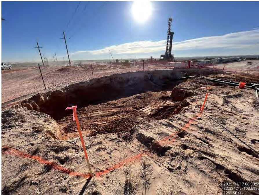
Excavated Area #4 on the pad, viewing southeast.
