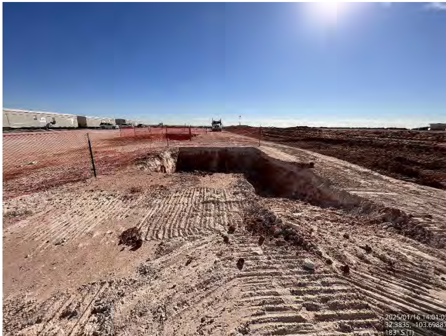
Excavated Area #2 on the pad, viewing south.
