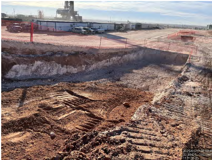
Excavated Area #4 on the pad, viewing southeast.
