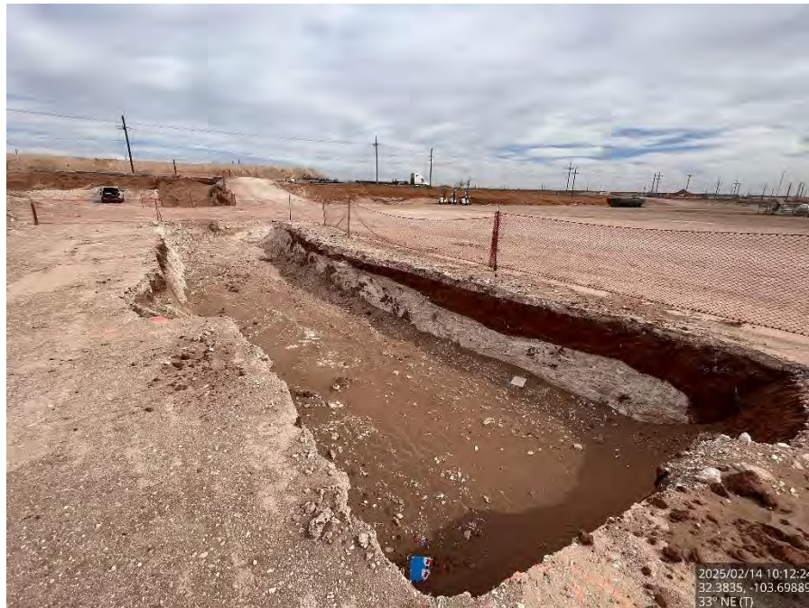
Excavated Area #3 on the pad, viewing northeast.
