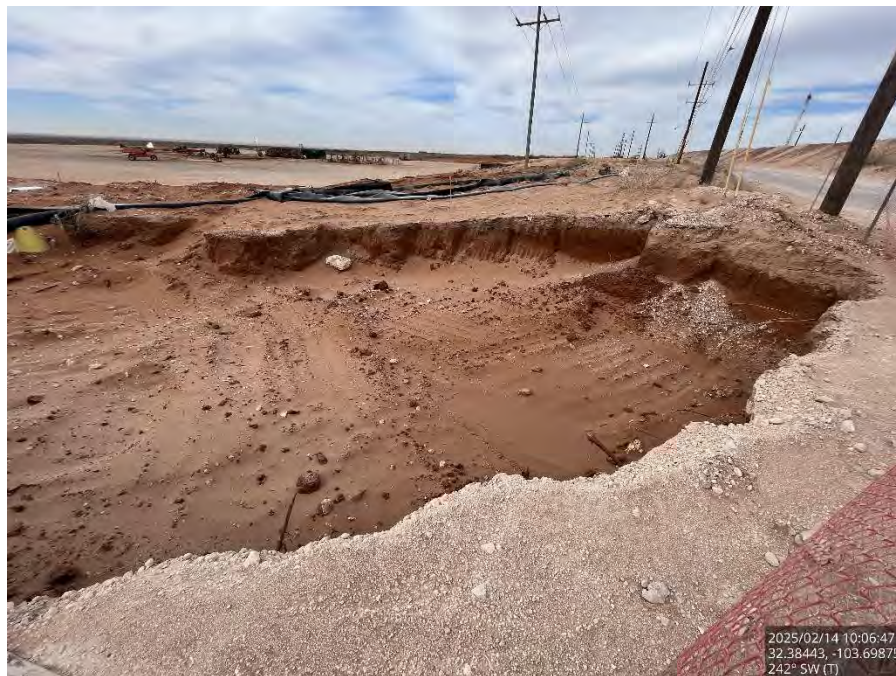
Excavated Area #4 on the pad, viewing southwest.
