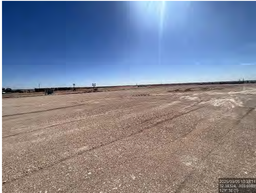
Backfilled area on the pad, viewing southeast.
