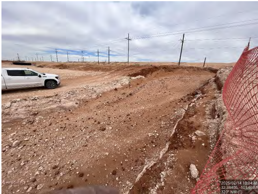
Excavated Area #4 on the pad, viewing northwest.
