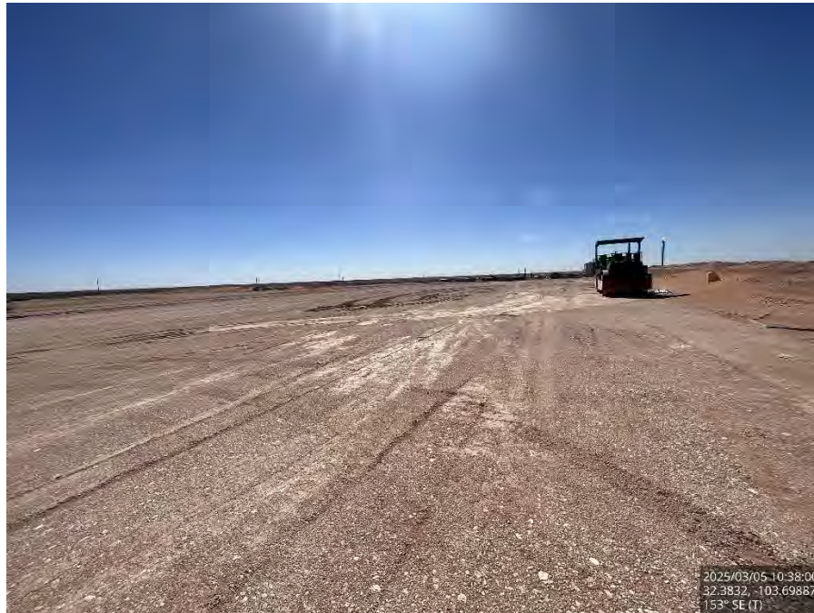
Backfilled area on the pad, viewing southeast.
