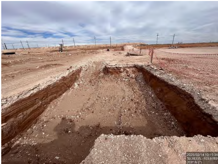
Excavated Area #2 on the pad, viewing north.
