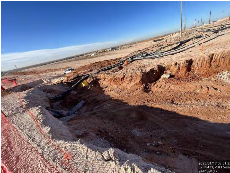
Excavated Area #4 on the pad, viewing southwest.
