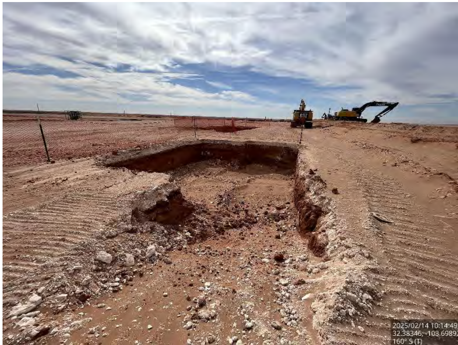
Excavated Area #2 on the pad, viewing south.
