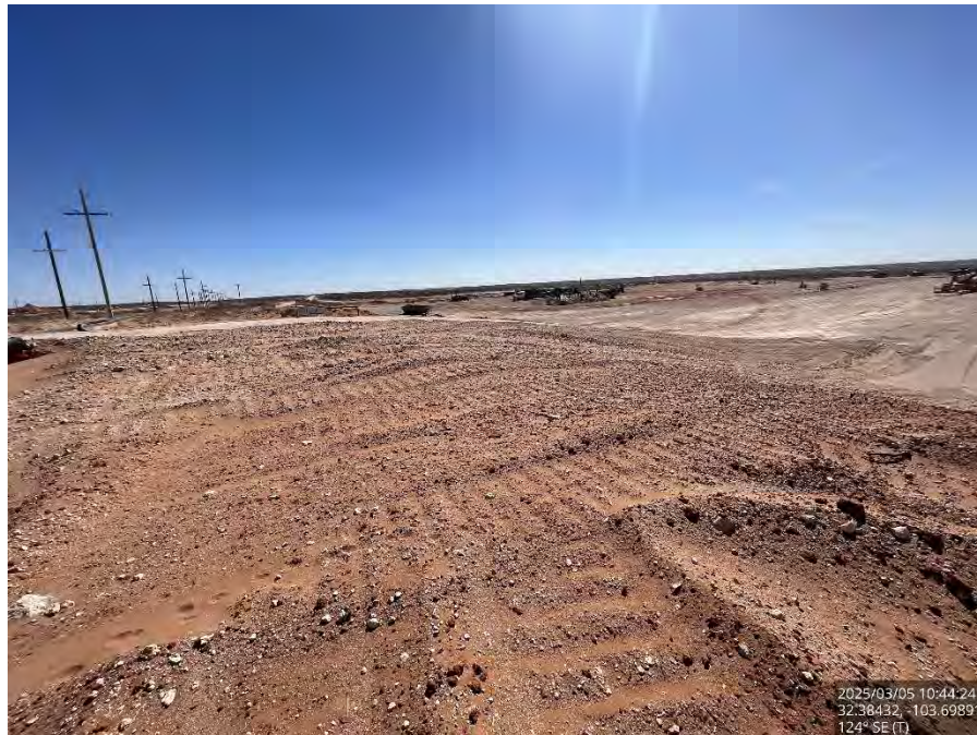
Backfilled area on the pad, viewing southeast.
