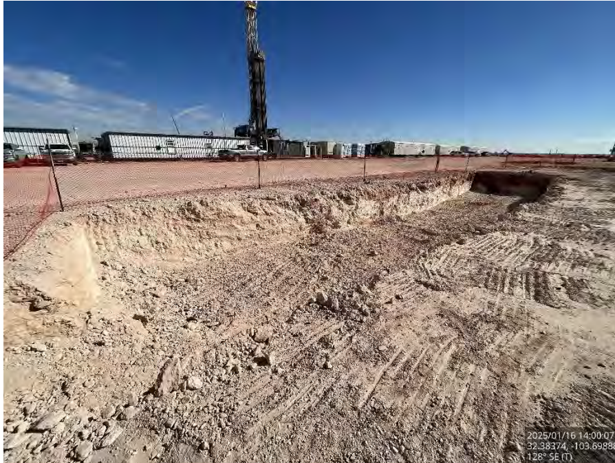
Excavated Area #3 on the pad, viewing southeast.
