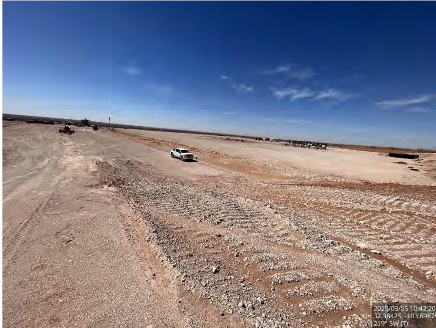
Backfilled area on the pad, viewing southwest.
