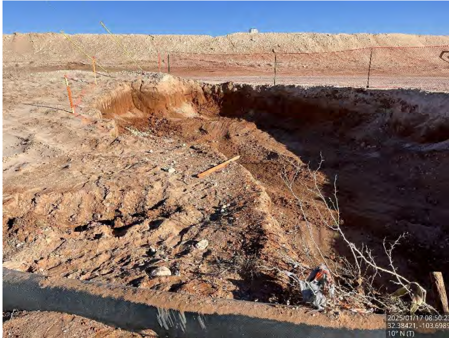
Excavated Area #4 on the pad, viewing north.
