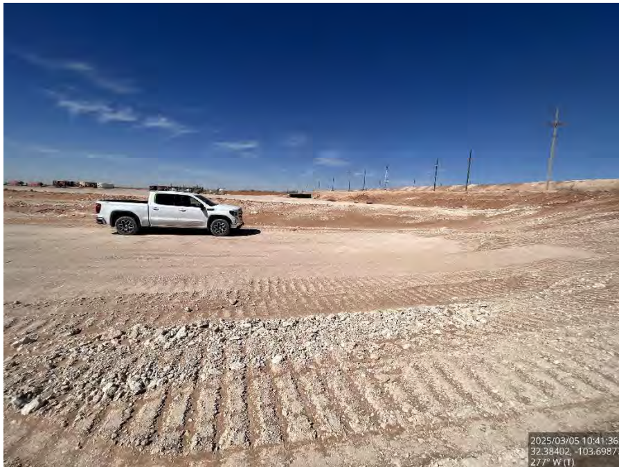
Backfilled area on the pad, viewing west.
