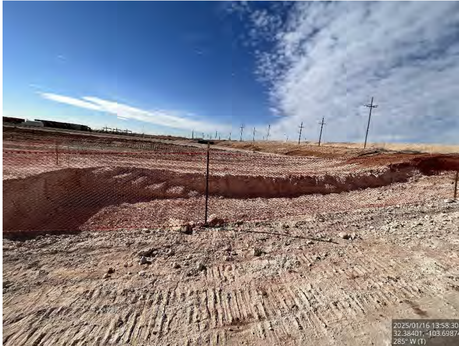
Excavated Area #4 on the pad, viewing west.
