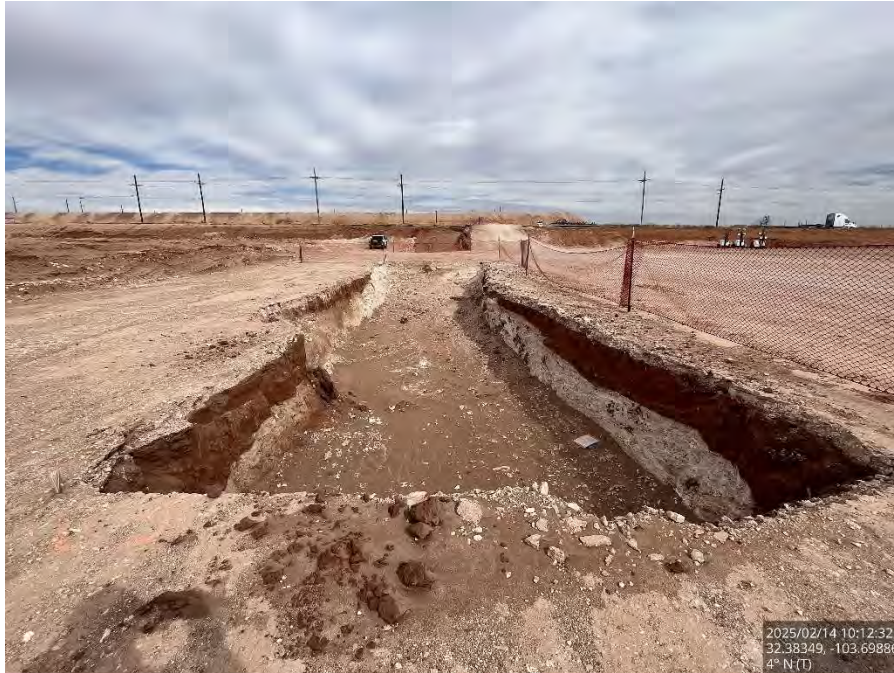
Excavated Area #3 on the pad, viewing north.
