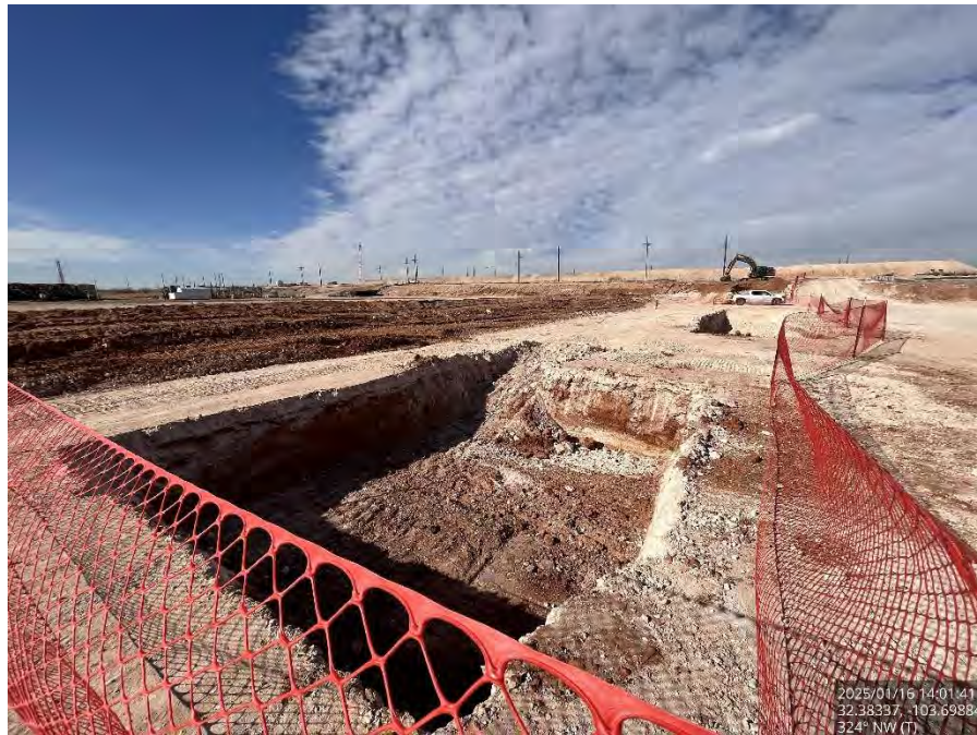
Excavated Area #2 on the pad, viewing northwest.
