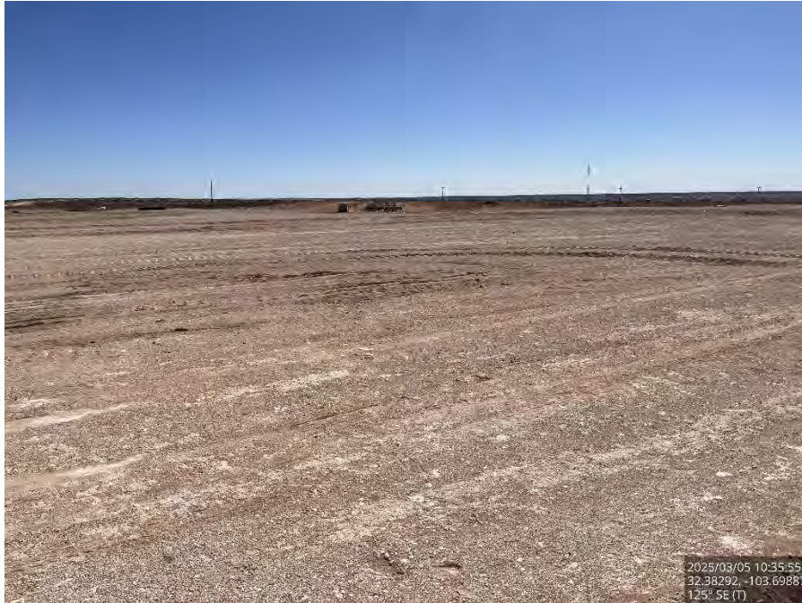
Backfilled Area on the pad, viewing southeast.
