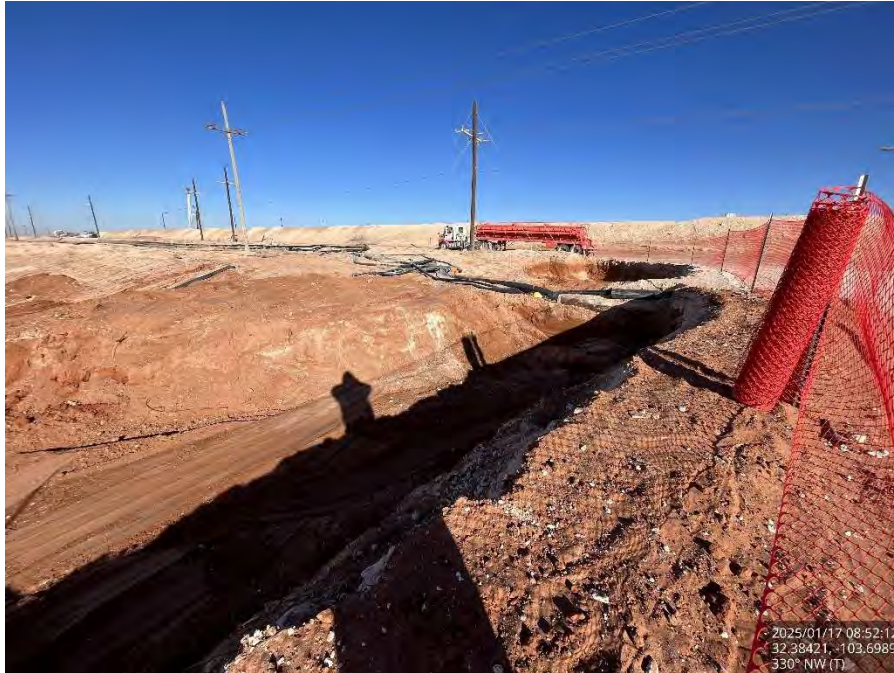
Excavated Area #4 on the pad, viewing northwest.
