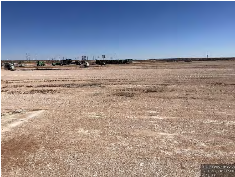
Backfilled area on the pad, viewing east.
