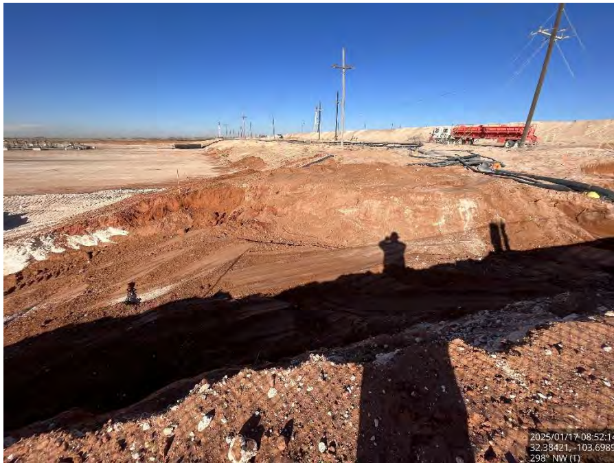
Excavated Area #4 on the pad, viewing northwest.
