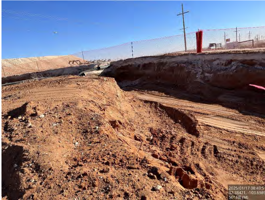
Excavated Area #4 on the pad, viewing northeast.
