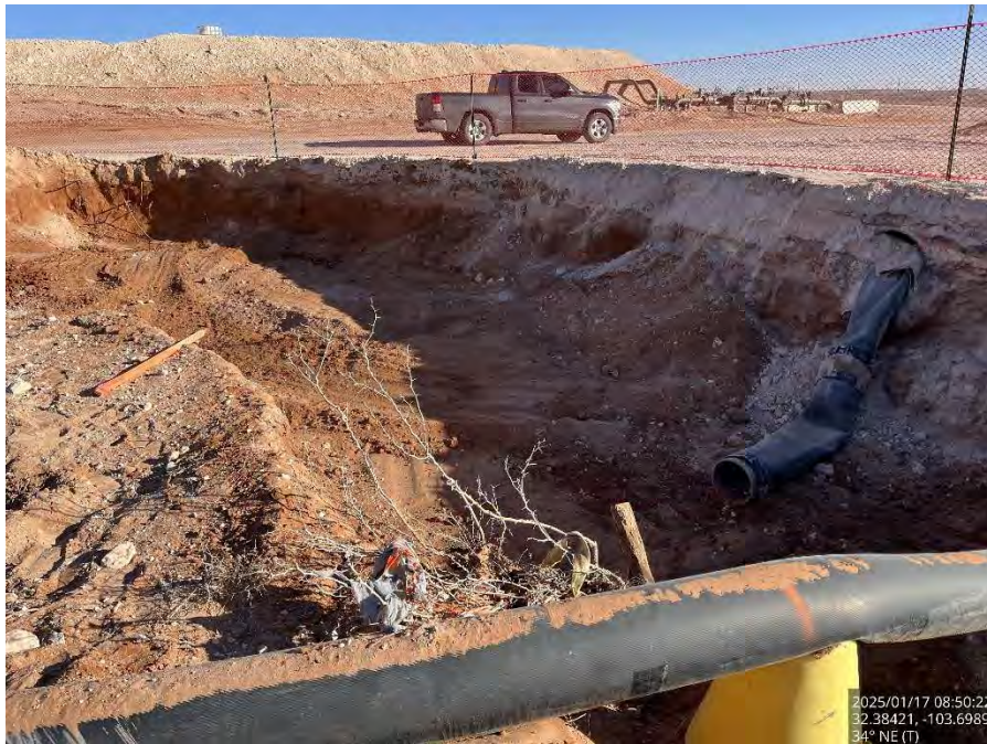
Excavated Area #4 on the pad, viewing northeast.
