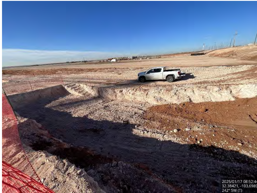
Excavated Area #4 on the pad, viewing southwest.
