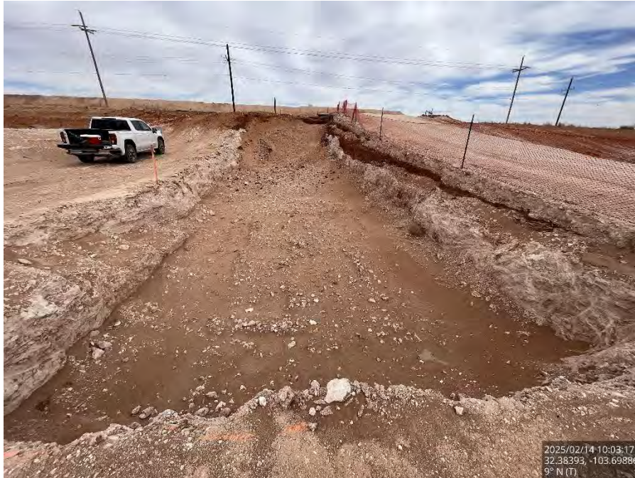
Excavated Area #4 on the pad, viewing north.
