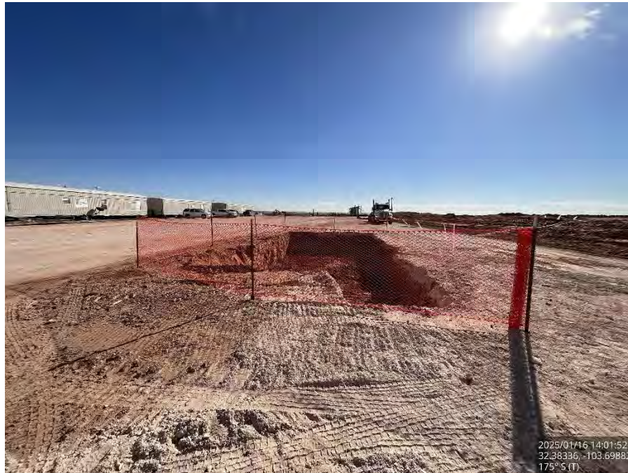
Excavated Area #1 on the pad, viewing south.
