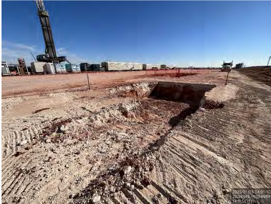
Excavated Area #2 on the pad, viewing southeast.
