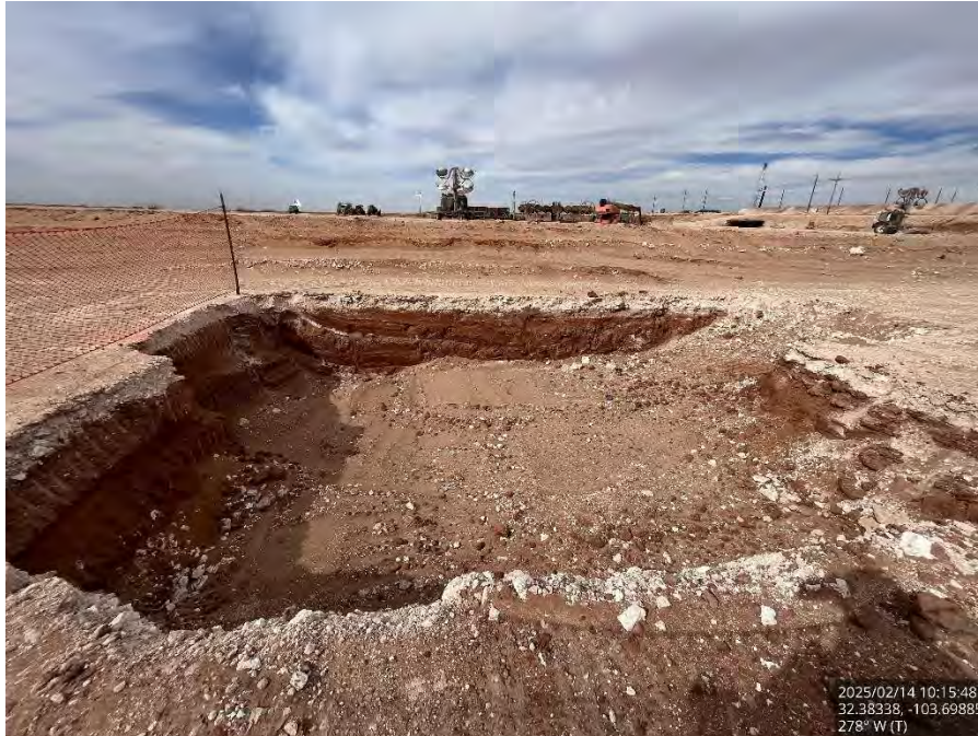
Excavated Area #2 on the pad, viewing west.
