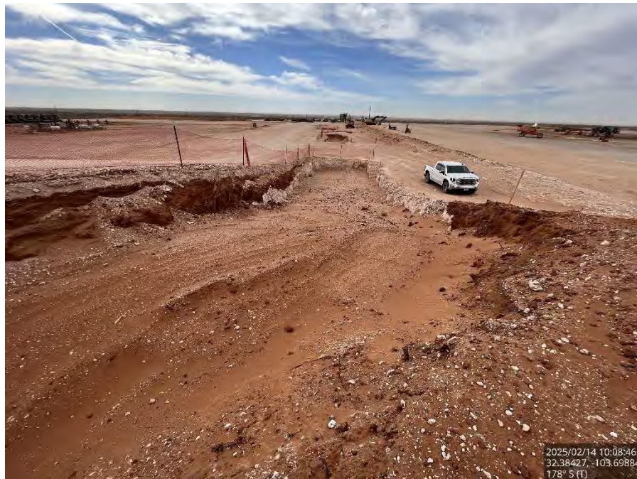
Excavated Area #4 on the pad, viewing south.
