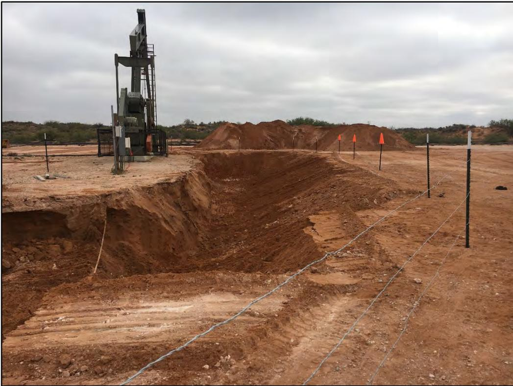
Photo 9. Excavation secured using 3-wire fencing.
