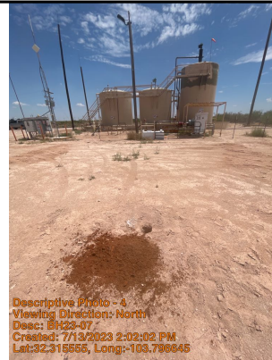
Viewing Direction: South
