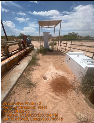
Viewing Direction: West
