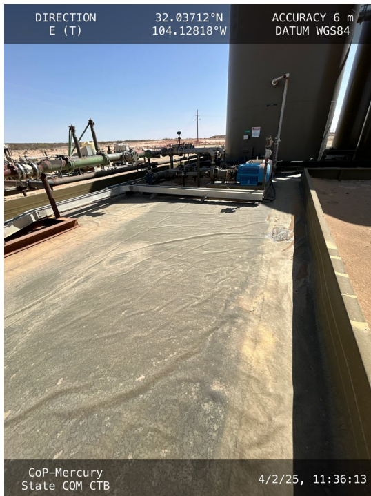
Photo 5 View of central portion of secondary containment.
