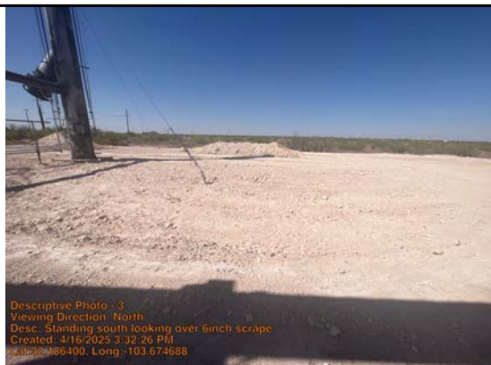
Standing south looking over 6inch scrape
