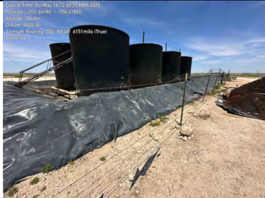
Outer walls of lined containment (east wall)
