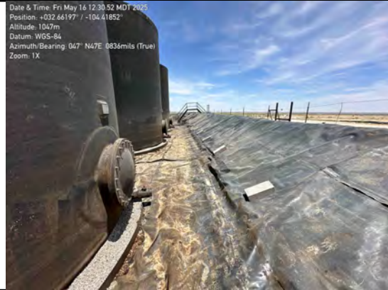
Inside walls of lined containment
