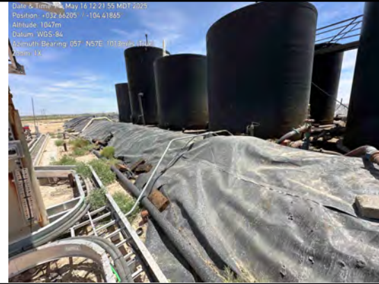
Outer walls of lined containment (west wall)
