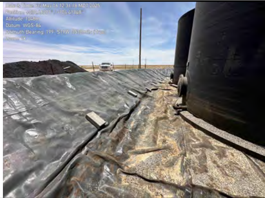
Inside walls of lined containment
