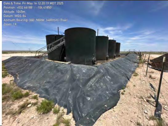
Outer walls of lined containment (south wall)
