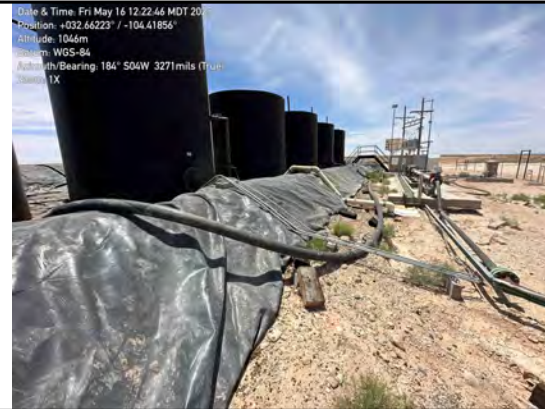
Outer walls of lined containment (west wall)
