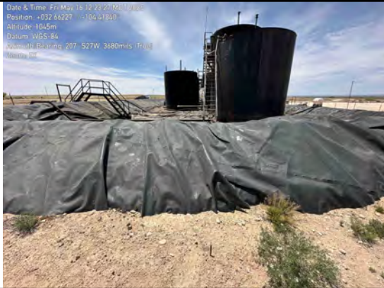
Outer walls of lined containment (north wall)
