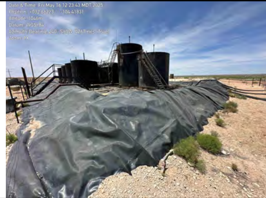
Outer walls of lined containment (north wall)
