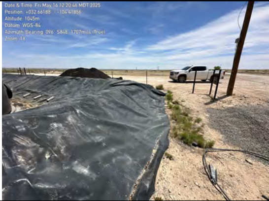
Outer walls of lined containment (south wall)
