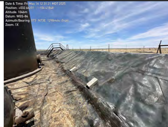
Inside walls of lined containment
