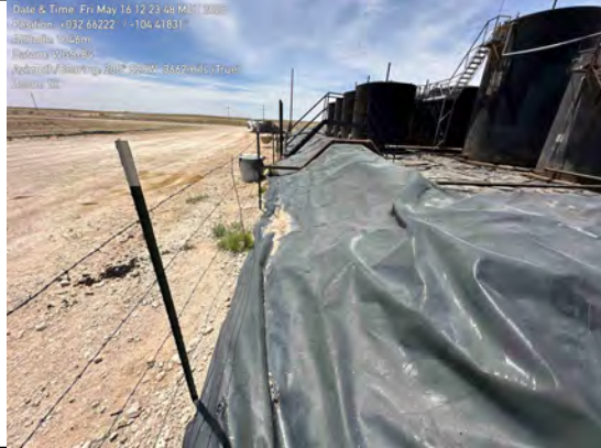
Outer walls of lined containment (east wall)
