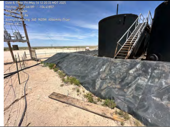
Outer walls of lined containment (south wall)
