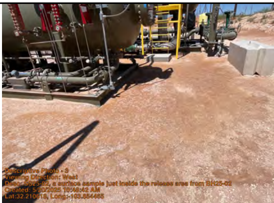
Viewing Direction: West
