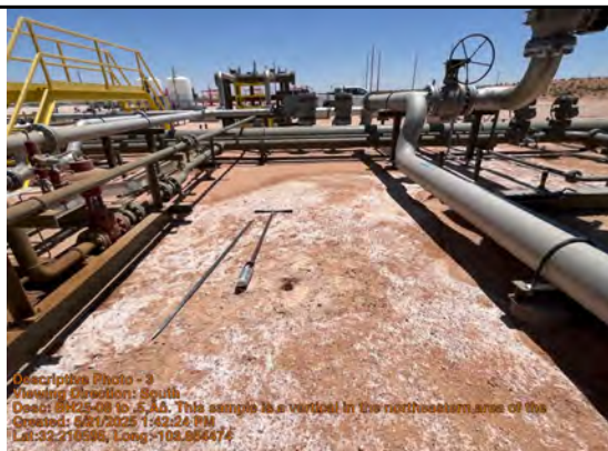
Viewing Direction: South
