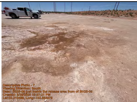
Viewing Direction: South
