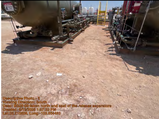
Viewing Direction: South
