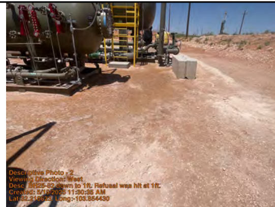
Viewing Direction: West
