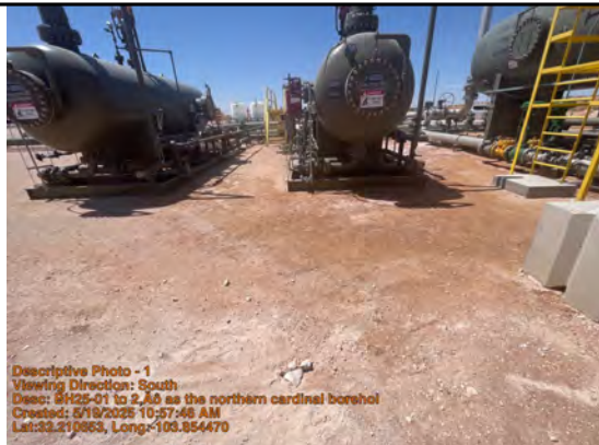
Viewing Direction: South
