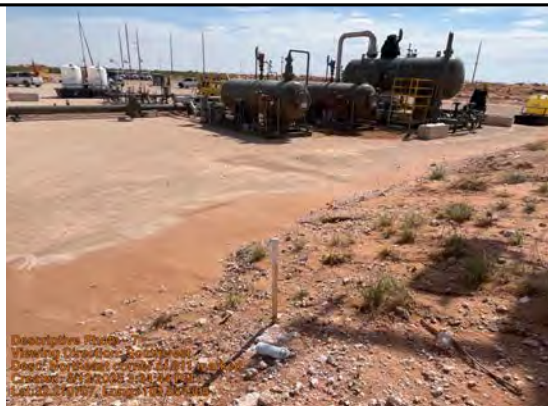
Northeast corner of 811 marked
