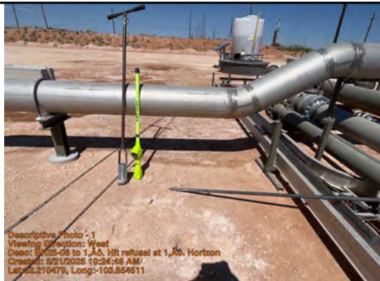
Viewing Direction: West
