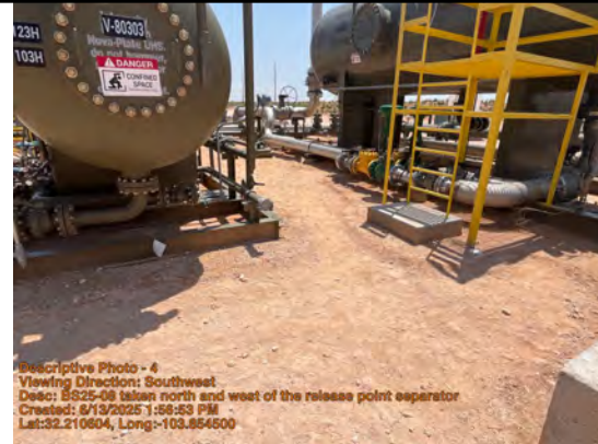
BS25-08 taken north and west of the release point separator
