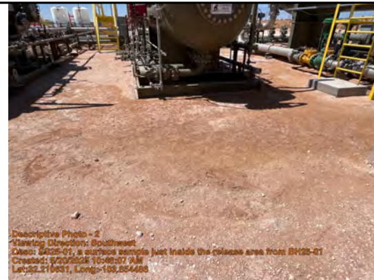
Viewing Direction: South
