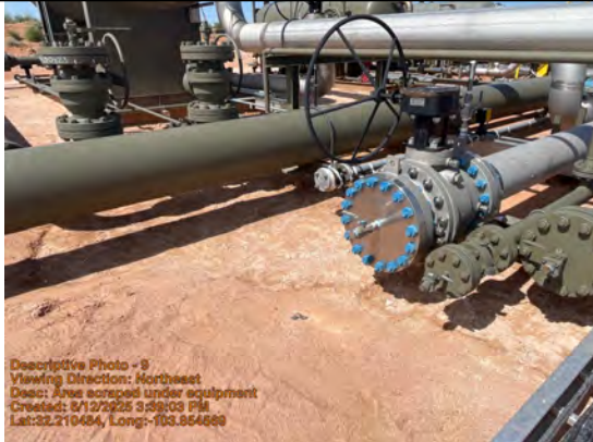
Area scraped under equipment
