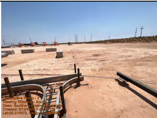
Viewing Direction: South
