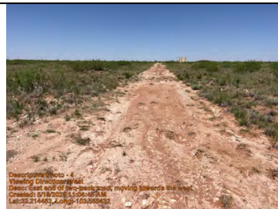
East half of ripped two-track road, moving towards the west
