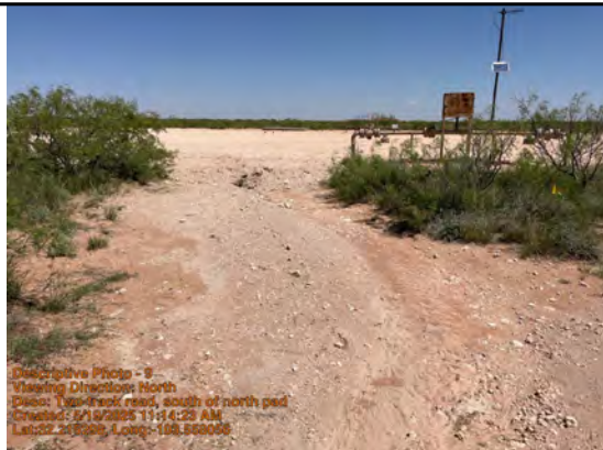
Ripped two-track road, south of north pad
