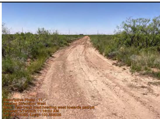
Ripped two-track road heading west towards pad/pit
