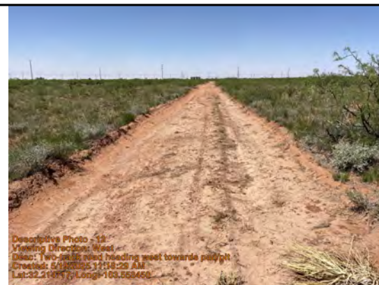
Ripped two-track road heading west towards pad/pit
