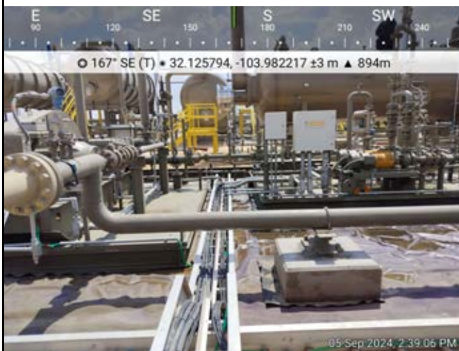
Photograph: 2 Description: Liner Inspection View: Southeast
