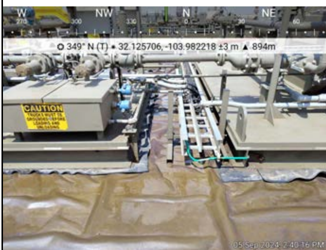
Photograph: 4 Description: Liner Inspection View: Northwest
