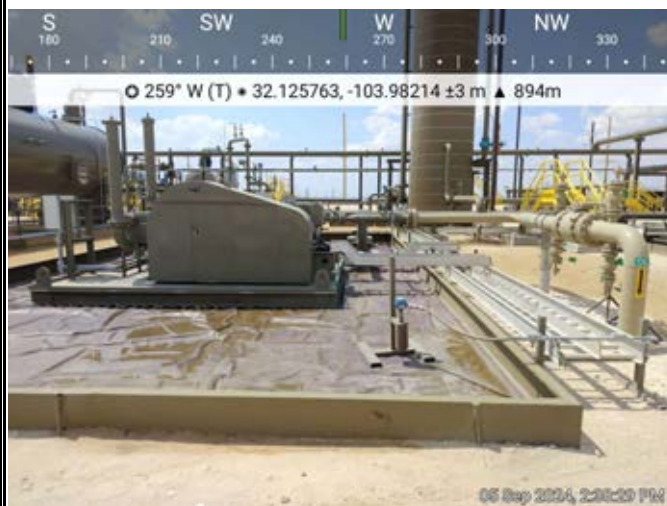
Photograph: 1 Description: Liner Inspection View: Southwest
