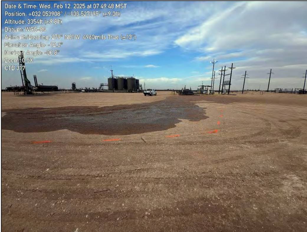
PHOTO 1: Northwestern view of release extent during excavation preparation. 2/12/2025
