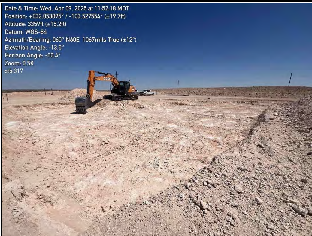
PHOTO 4: Northeastern view during excavation activities. 4/9/2025
