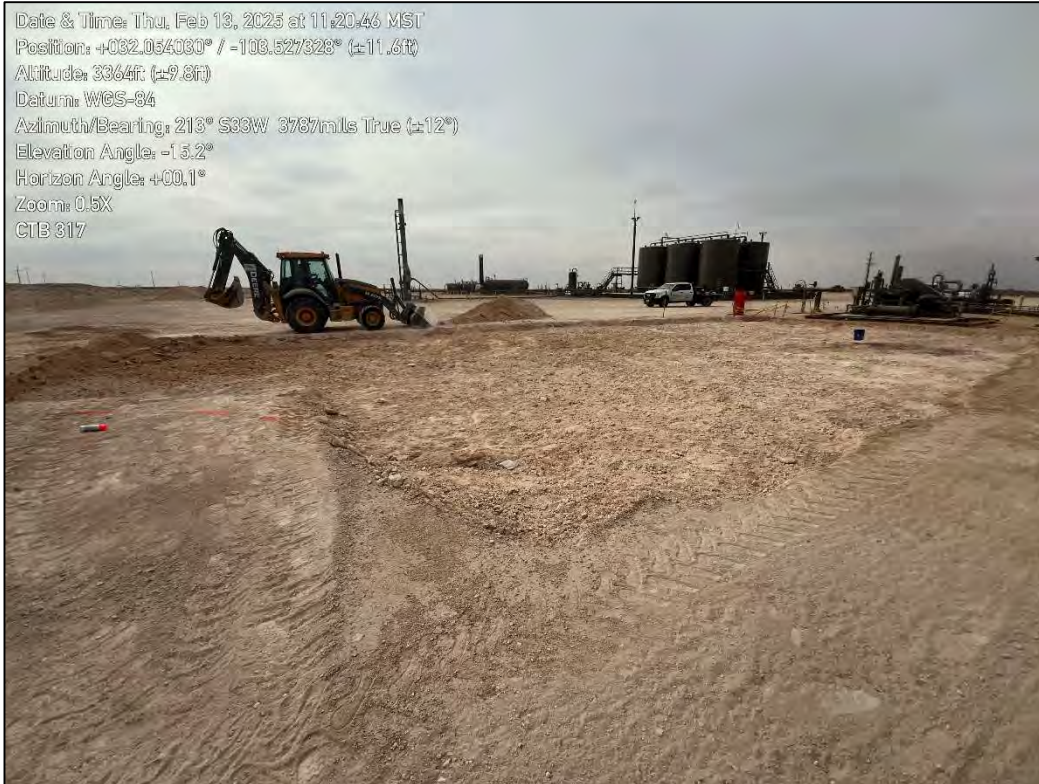
PHOTO 3: Southwestern view during excavation activities. 2/13/2025
