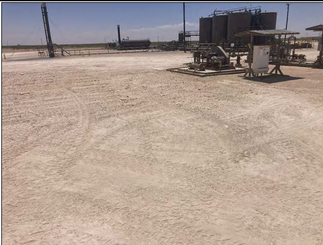
PHOTO 7: Southwestern view following restoration activities. 4/29/2025
