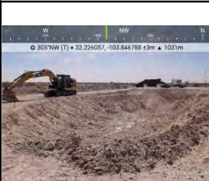
Photograph: 1 Date: 3/12/2025 Description: Deferral excavation extent 15' deep View: Northwest
