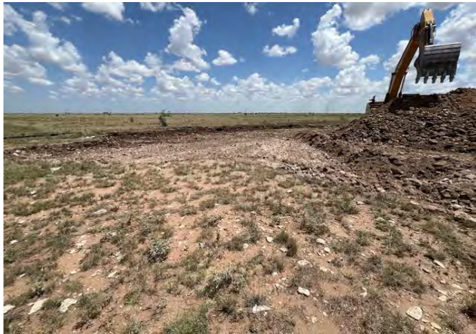
View to SE of excavation (6/19/25).
