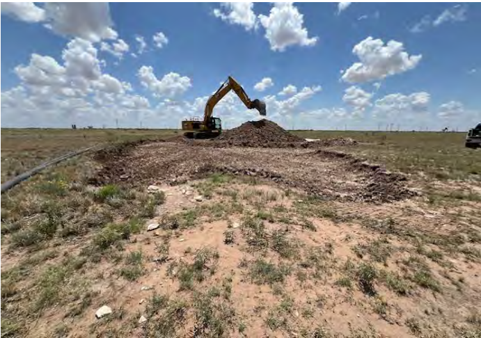
View to E of excavation (6/19/25).
