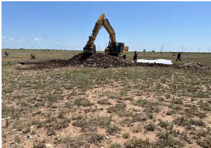
View to E of excavating and laying plastic (6/19/25).
