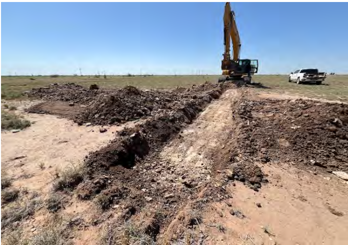
View to SE of N to S trench (6/19/25).
