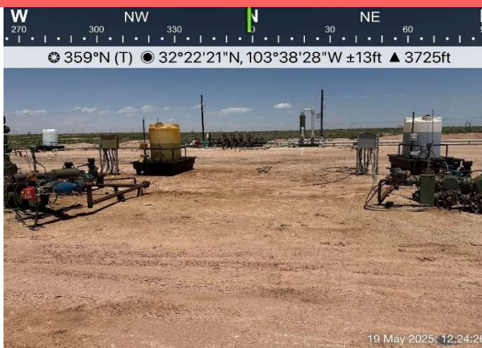
View of Area of Concern
