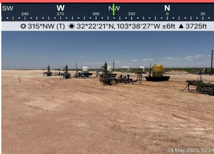
View of Area of Concern
