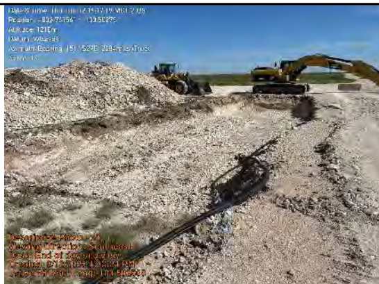
End of day site view
