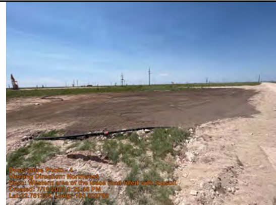
Western area of the lease road filled with topsoil
