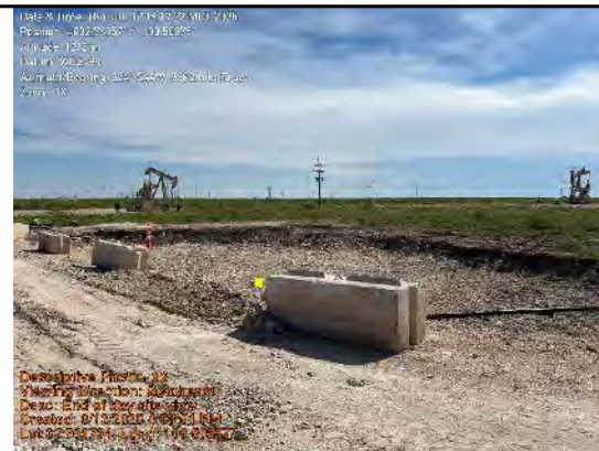
End of day site view
