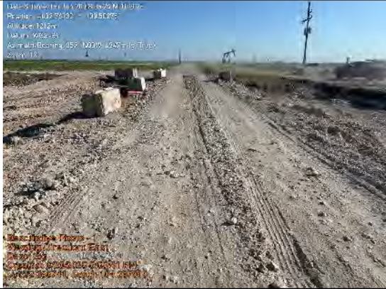
Photo of the road before excavation begins.
