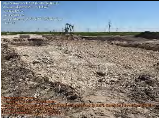
Photo showing the road has been removed to 3.5ft. Samples have been acquired and will be field screened.
