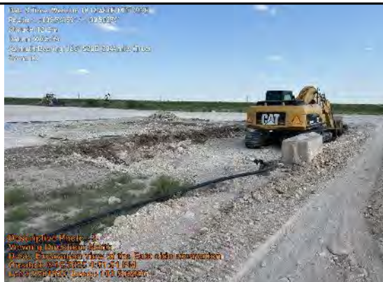
Excavation view of the East side excavation
