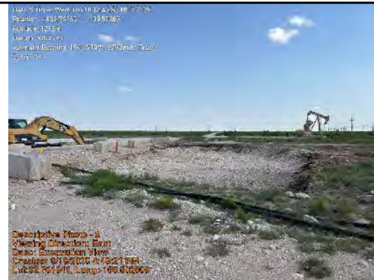
Excavation View of the West side excavation
