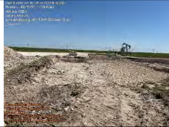
Photo showing the road has been removed to 3.5ft
