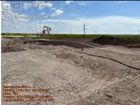
End of day site view
