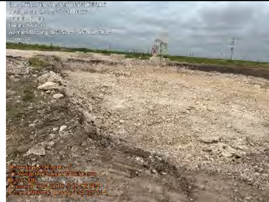
Site view of excavation
