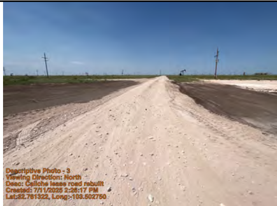
Caliche lease road rebuilt
