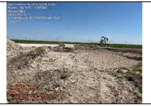
Photo showing the road has been removed to 3.5ft
