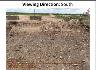
Inside excavation facing south. Collected excavation wall sample WS25-09 from 0 to 4 feet bgs.
