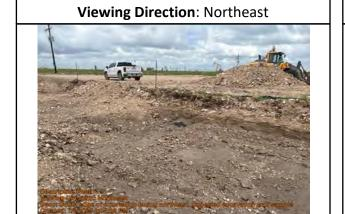
South edge of excavation facing northeast. Collected excavation wall sample WS25-08 from 3 to 5 feet bgs.
