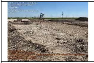
Photo showing the road has been removed to 3.5ft. Samples have been acquired and will be field screened.
