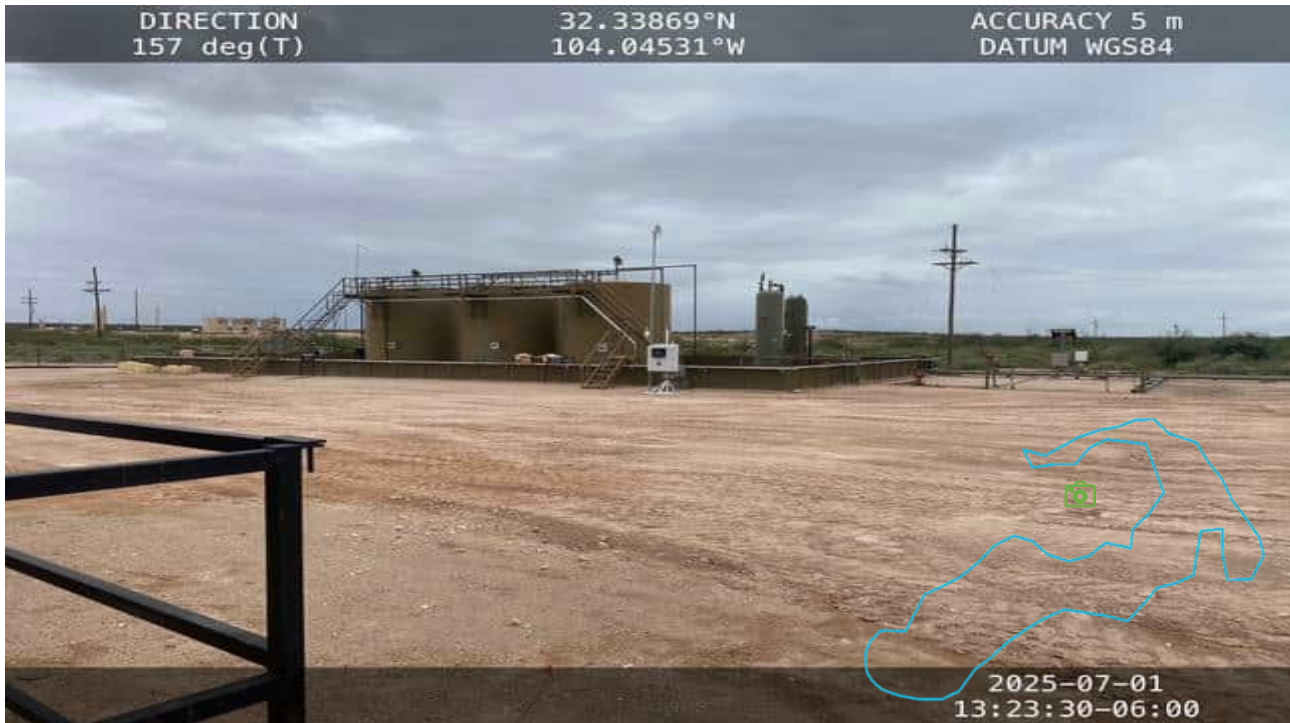
Photo 11 View of backfilled excavation area from center of pad looking S
