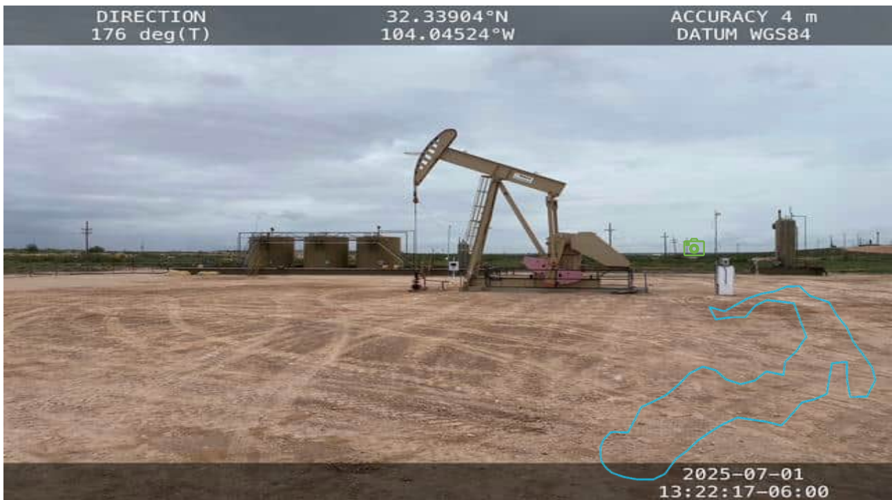
Photo 14 View of backfilled excavation area from NW corner of Pumpjack looking SE
