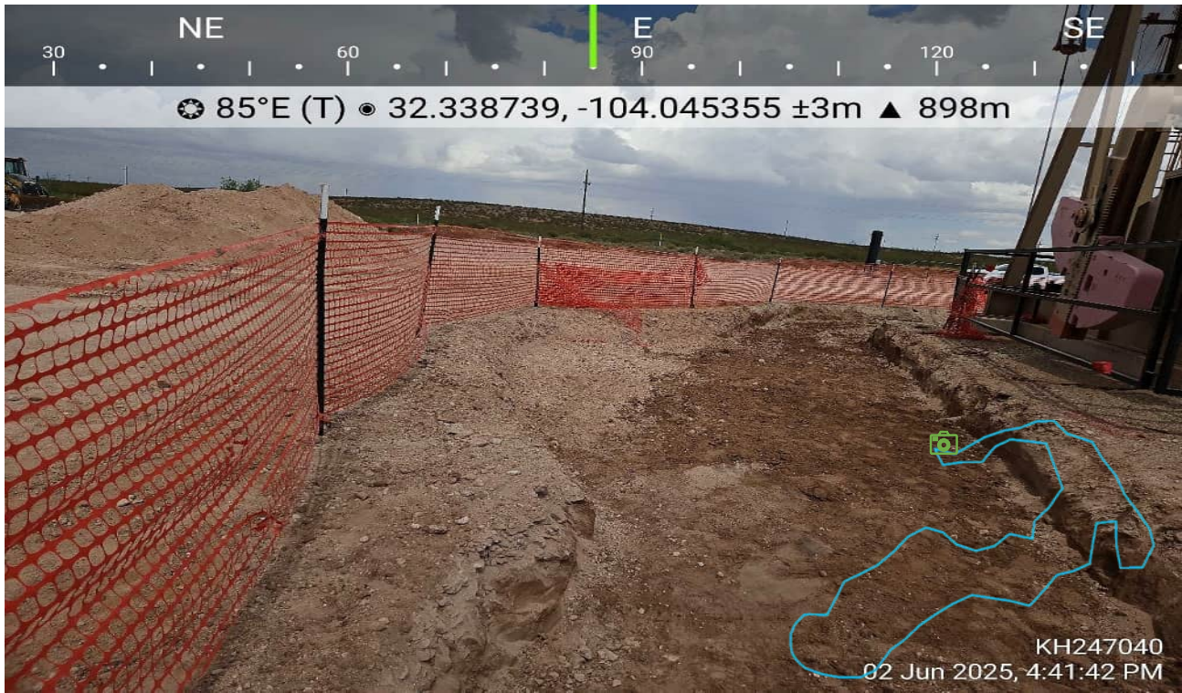
Photo 13 View of excavated area from NW corner of Pumpjack looking E
