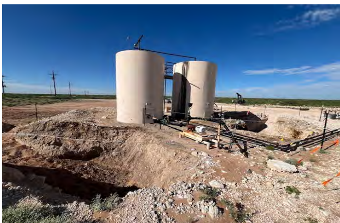
View to SW of TB excavations (8/7/25).
