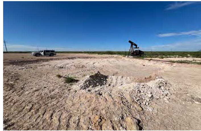
View to SW of well pad excavation (8/7/25).
