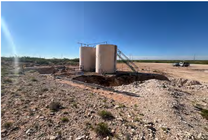
View to SE of TB excavations (8/7/25).
