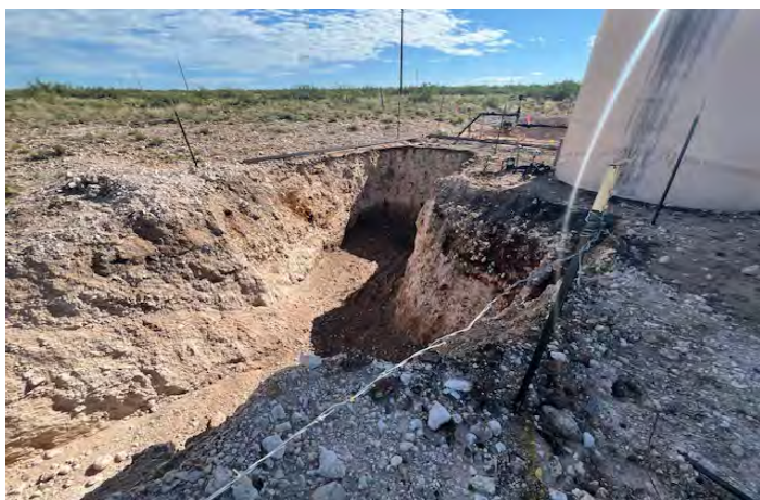
View to NW of W TB excavation (8/7/25).
