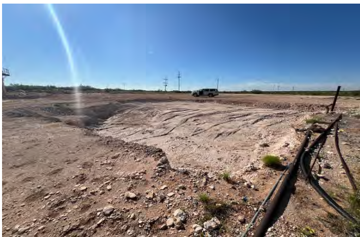
View to S of well pad excavation (8/7/25).
