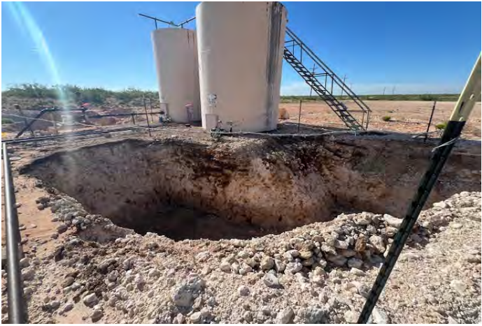
View to SE of W TB excavation (8/7/25).
