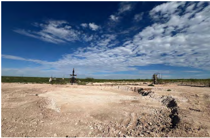
View to W of well pad excavation (8/7/25).
