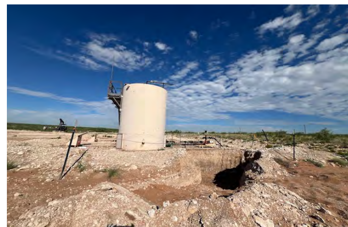
View to W of E TB excavation (8/7/25).
