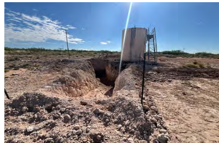
View to E of W TB excavation (8/7/25).
