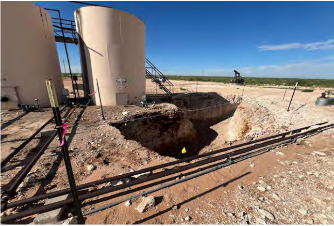
View to SW of E TB excavation (8/7/25).
