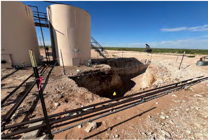
View to SW of E TB excavation (8/7/25).
