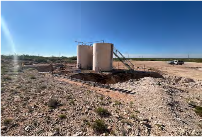
View to SE of TB excavations (8/7/25).
