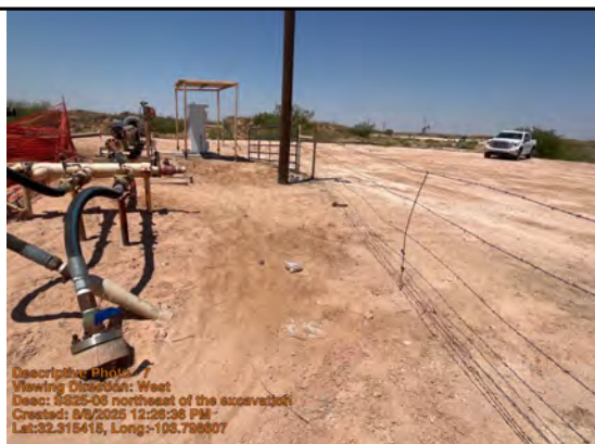
SS25-06 northeast of the excavation
