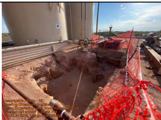
Excavation area from the southwest
