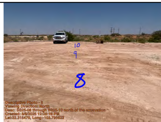
SS25-08 through SS25-10 north of the excavation
