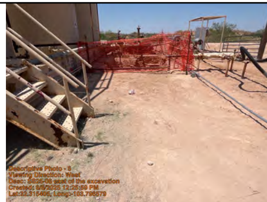
SS25-06 east of the excavation
