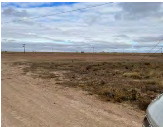
View to west of backfilled excavation (11/14/22).
