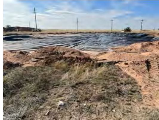
View to northeast of installed liner (11/3/22).
