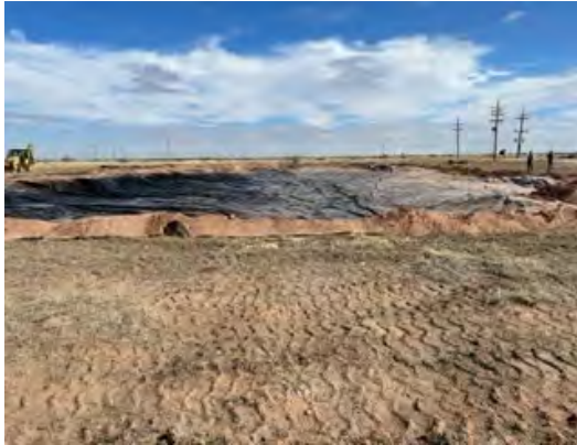
View to north of installed liner (11/3/22).
