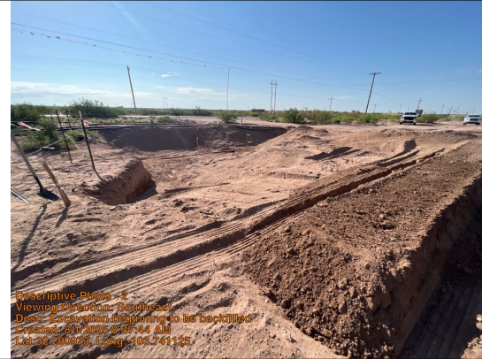
Excavation beginning to be backfilled
