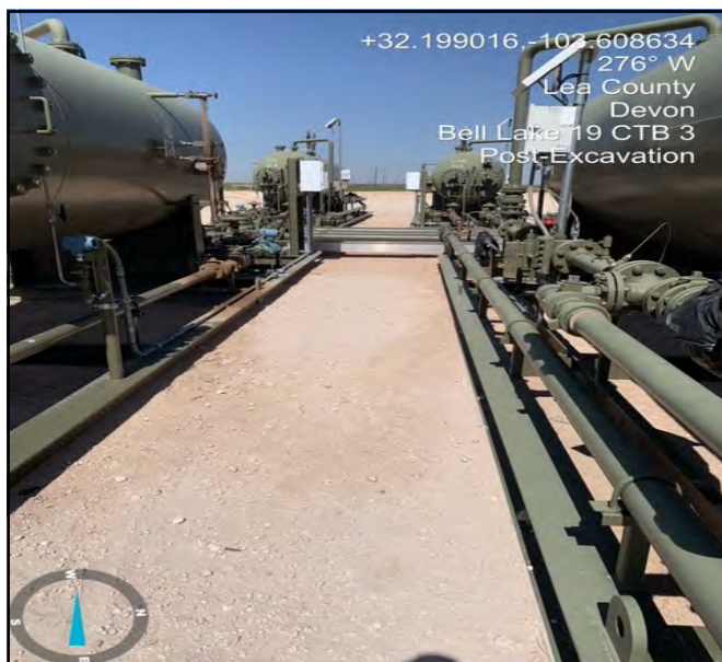
Photograph illustrating the area after backfilling with clean material facing West.
