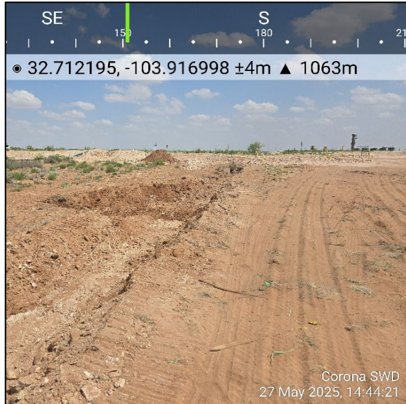
Photograph: 1 Date: 5/27/2025 Description: Excavation Activities View: Southeast
