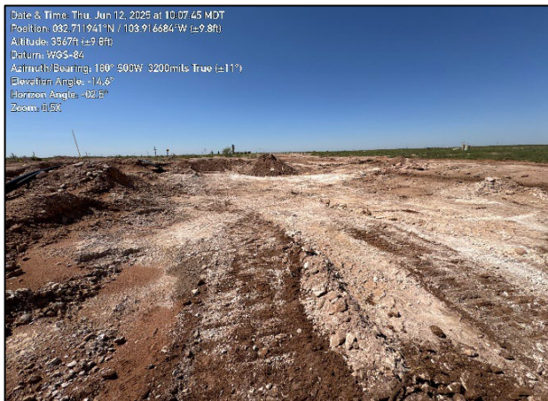
Photograph: 7 Date: 6/12/2025 Description: Excavation Area of FS01-FS14, FS18, FS20, FS21 View: Southwest
