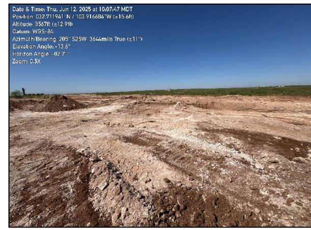
Photograph: 8 Date: 6/12/2025 Description: Excavation Area of FS01-FS09, FS11, FS18 View: Southwest
