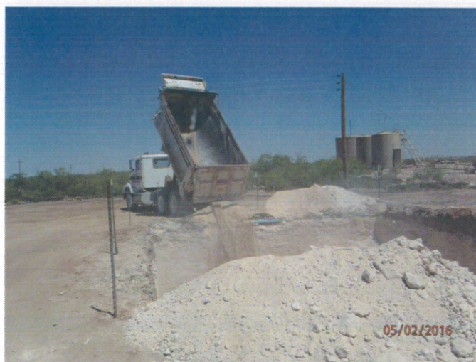
Backfilling the excavation with imported caliche, facing East 5/2/2016
