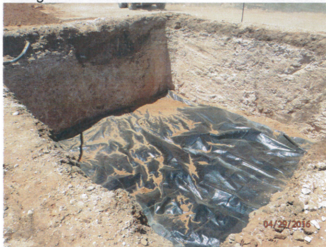
20-mil, reinforced liner installed at 11.5 ft bgs, Facing northwest 4/29/2016
