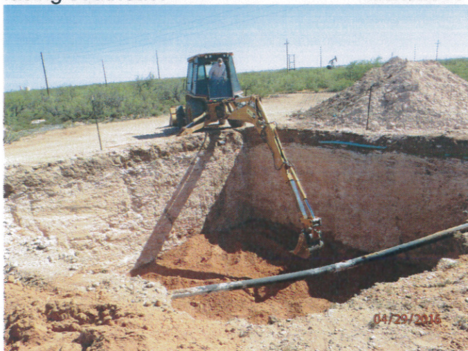
Padding the bottom of the excavation with imported blow sand, facing northeast 4/29/2016
