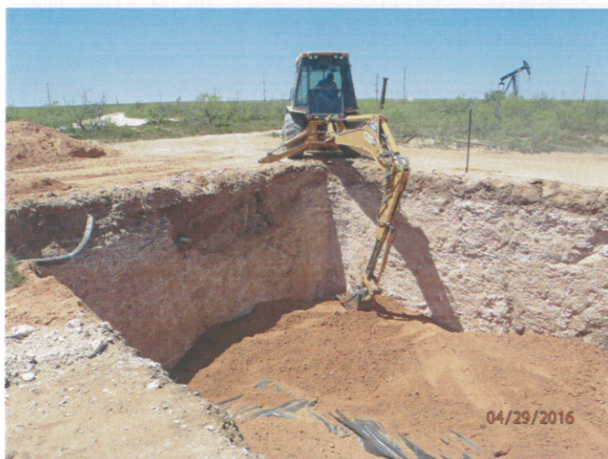
Padding the top of the liner with imported blow sand, facing northwest 4/29/2016
