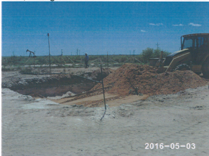
Backfilling the excavation with imported soil, facing southwest 5/3/2016
