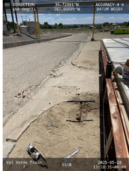
Photograph 10 Date: 05/28/2025 Description: SS10 View: South
