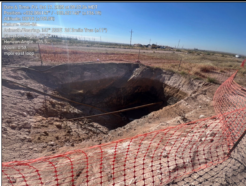
PHOTO 8: Northeastern view of site assessment activities. 10/17/2025
