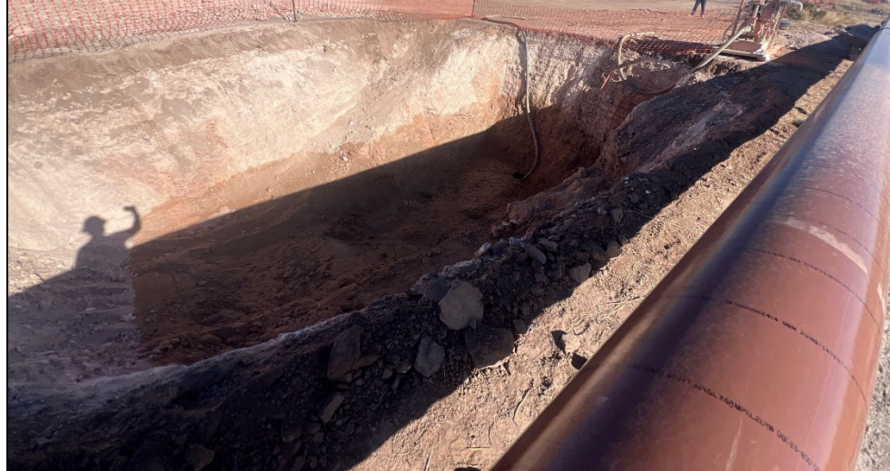
PHOTO 6: Northeastern view of site assessment activities. 10/17/2025
