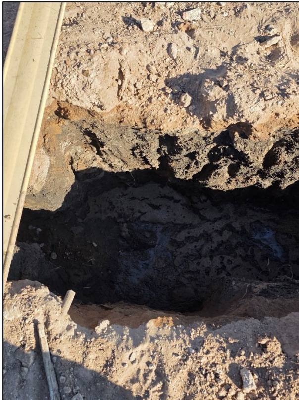
PHOTO 2: Southeastern view during initial site assessment by Contractor (Primoris). 10/14/2025
