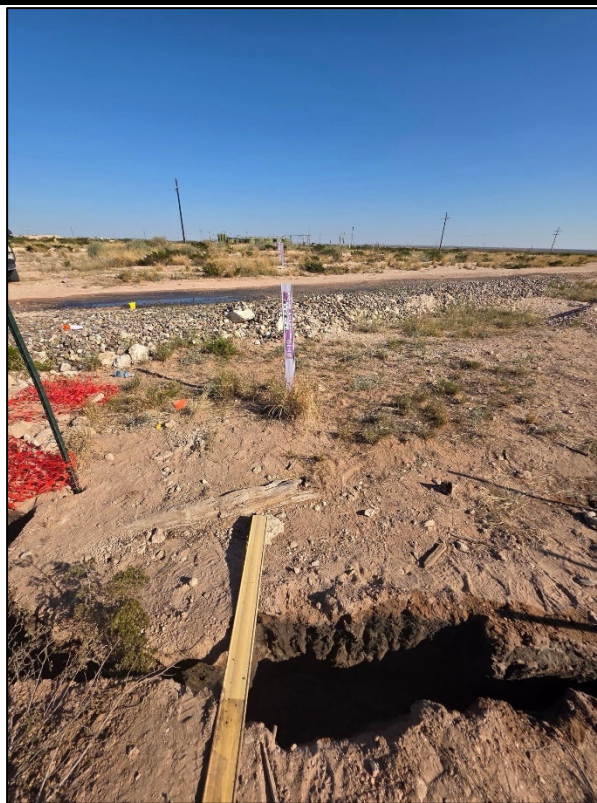
PHOTO 3: Southeastern view during initial site assessment by Contractor (Primoris). 10/14/2025
