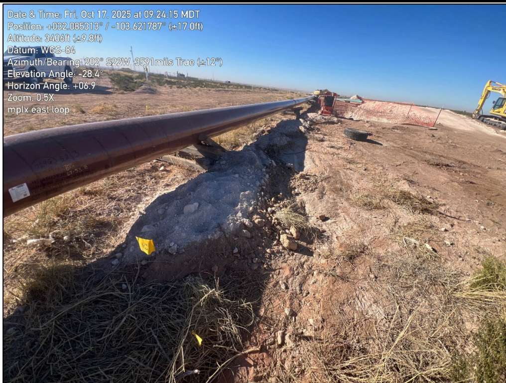
PHOTO 4: Northeastern view of site assessment activities. 10/17/2025
