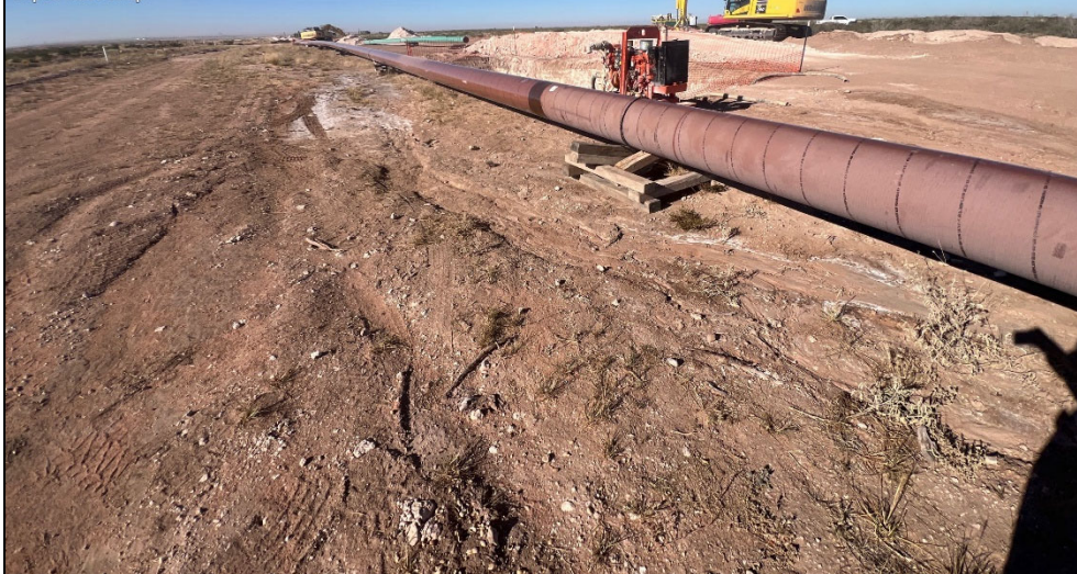
PHOTO 5: Northeastern view of site assessment activities. 10/17/2025
