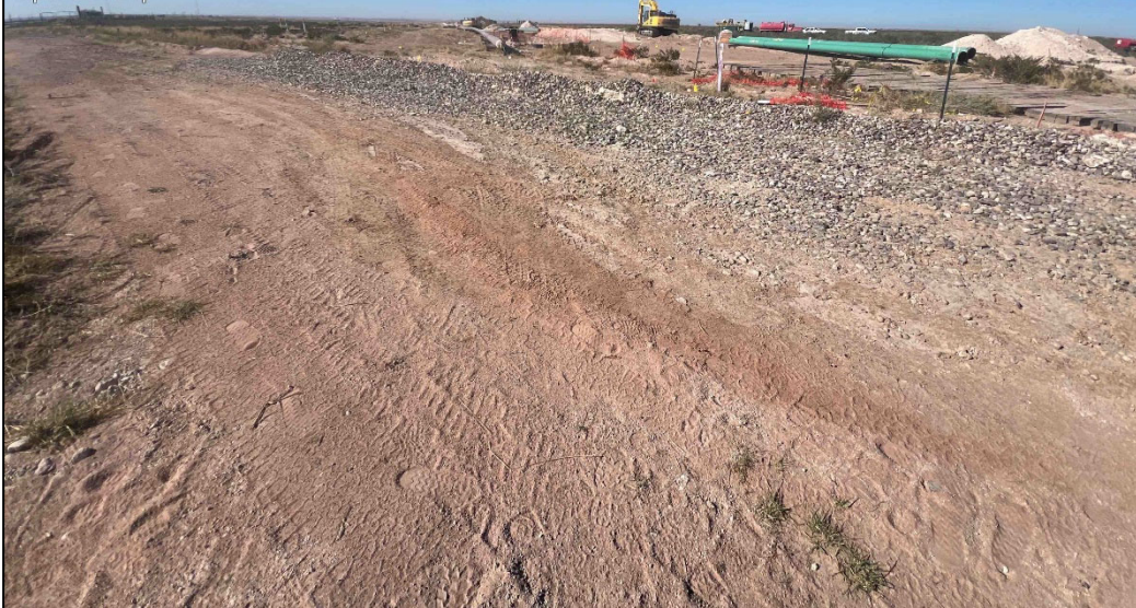
PHOTO 9: Northeastern view of site assessment activities. 10/17/2025
