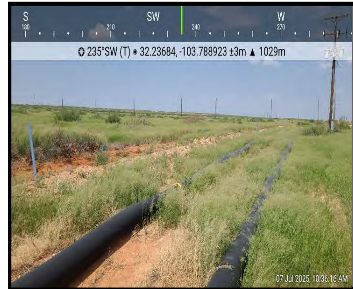
View of Area of Concern
