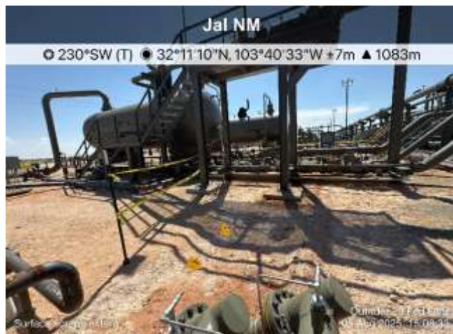
Photograph: 3 Date: 8/05/2025 Description: Surface scrape activities; near CS01 View: Southwest
