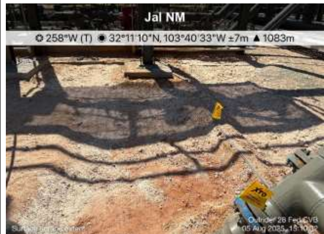
Photograph: 4 Date: 8/05/2025 Description: Surface scrape activities; near CS01 View: West
