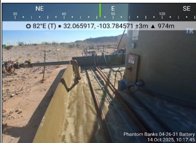
Photograph: 9 Date: 10/14/2025 Description: Liner inspection activities View: East
