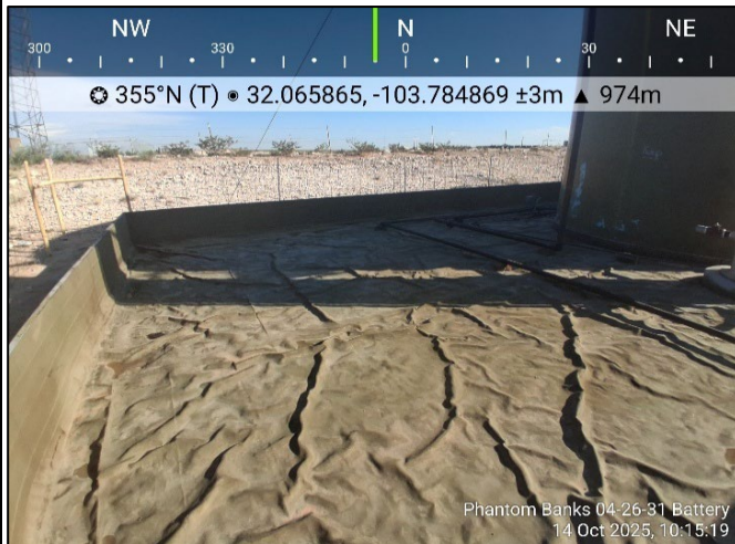
Photograph: 7 Date: 10/14/2025 Description: Liner inspection activities View: North
