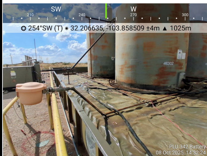
Photograph: 11 Date: 10/8/2025 Description: Non-invasive liner restoration coating View: West
