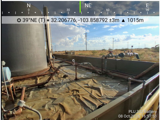
Photograph: 10 Date: 10/8/2025 Description: Non-invasive liner restoration coating View: Northeast
