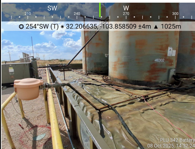
Photograph: 11 Date: 10/8/2025 Description: Non-invasive liner restoration coating View: West
