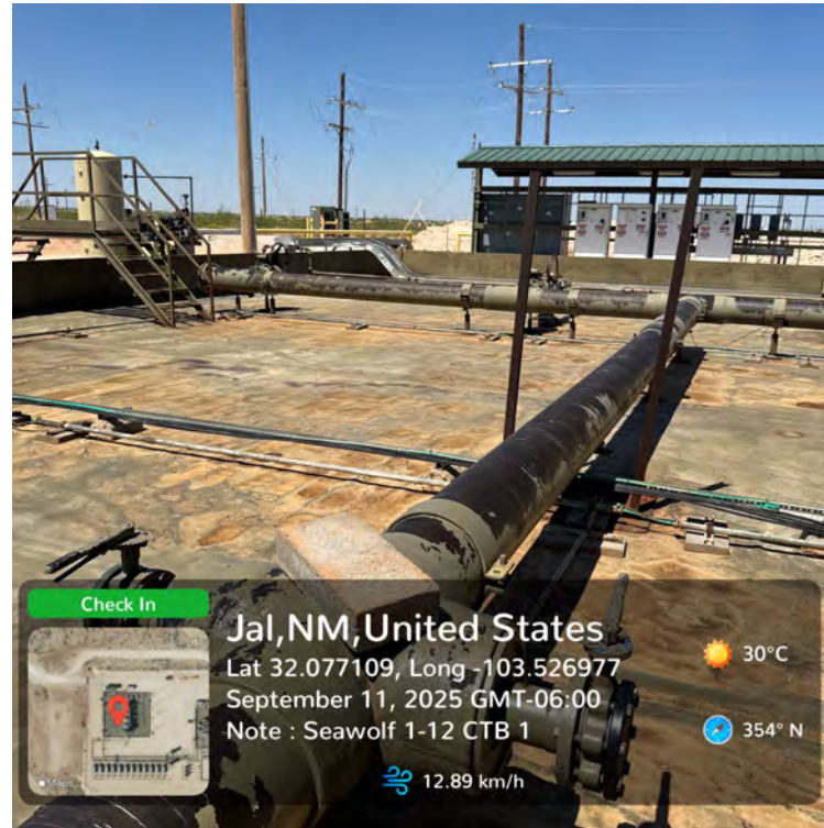
Northeast corner of liner facing north.
