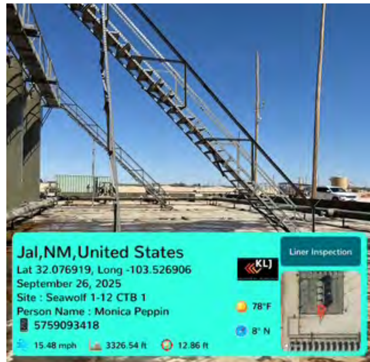
West view of liner from south end facing north.
