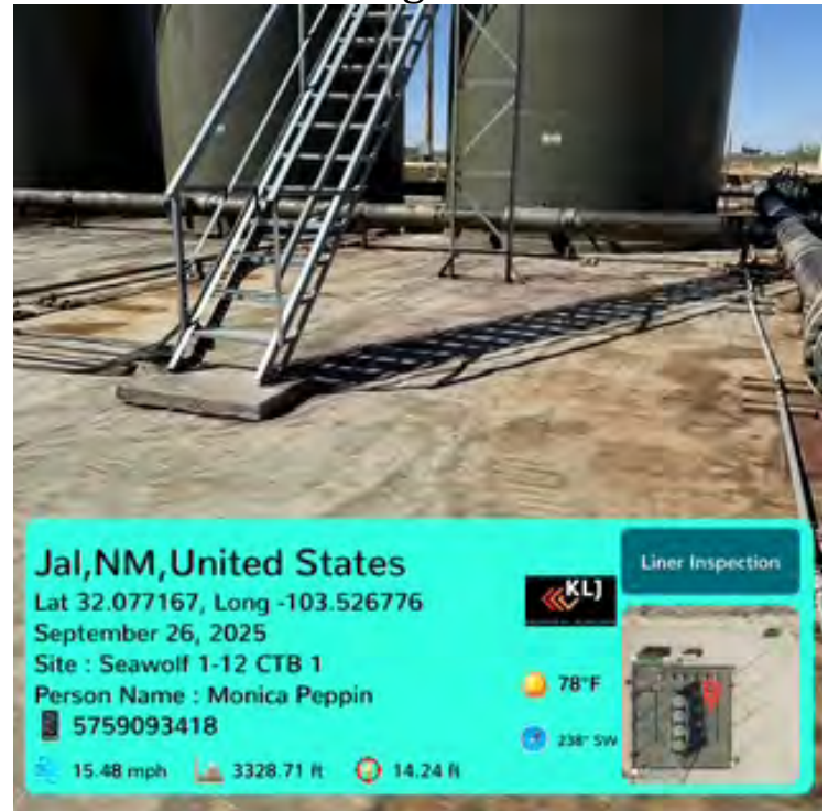
South wall view of liner facing west.
