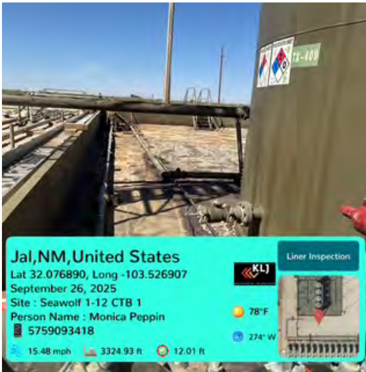
Liner on west side of containment facing northeast towards tanks.
