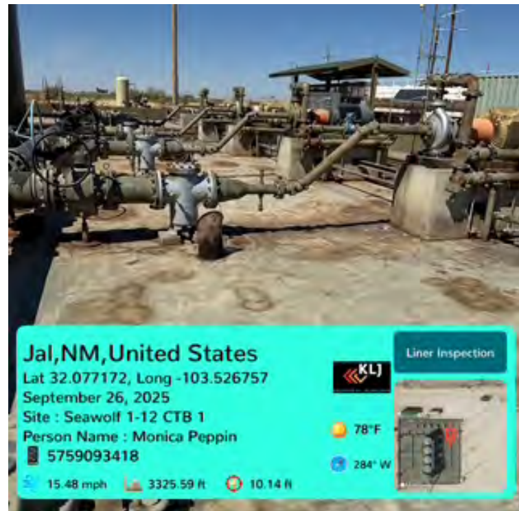
East view from west side towards tanks.
