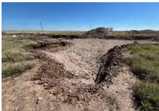
View to E of mid portion of excavation.
