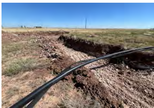
View to N of mid portion of excavation.
