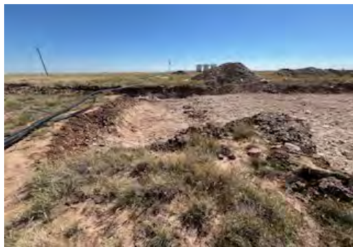
View to E of N end of excavation.
