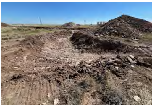
View to N of S end of excavation.
