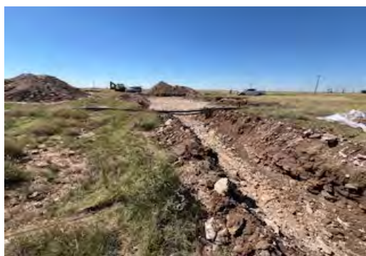
View to S of excavation from N end.
