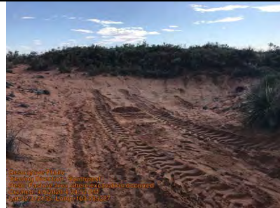
Pasture area where excavation occurred
