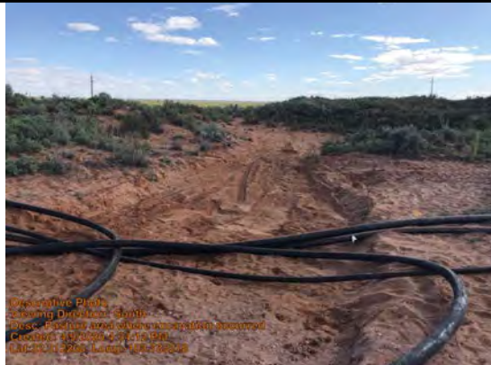
Pasture area where excavation occurred
