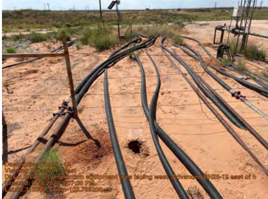
Viewing Direction: West
