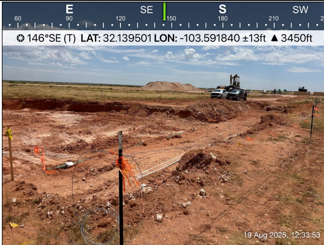
PHOTO 19: Southeastern view of excavation extent. 8/19/2025
