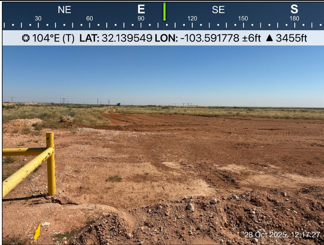
PHOTO 23: Southeastern view following restoration activities. 10/28/2025
