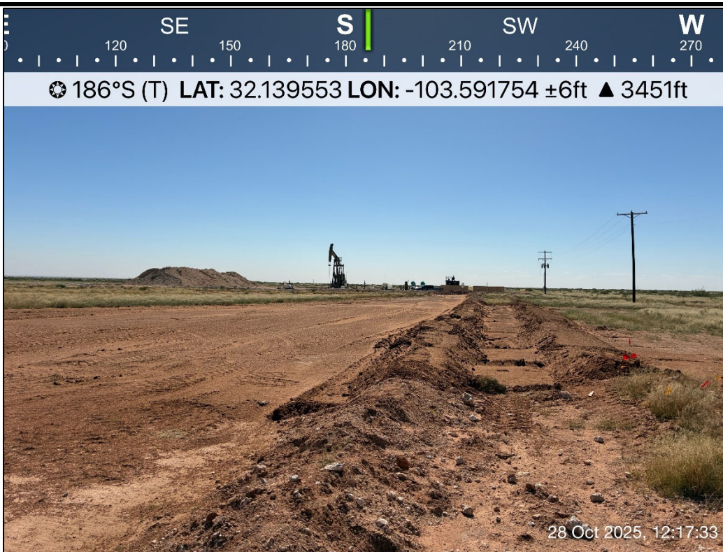
PHOTO 26: Southern view following restoration activities. 10/28/2025
