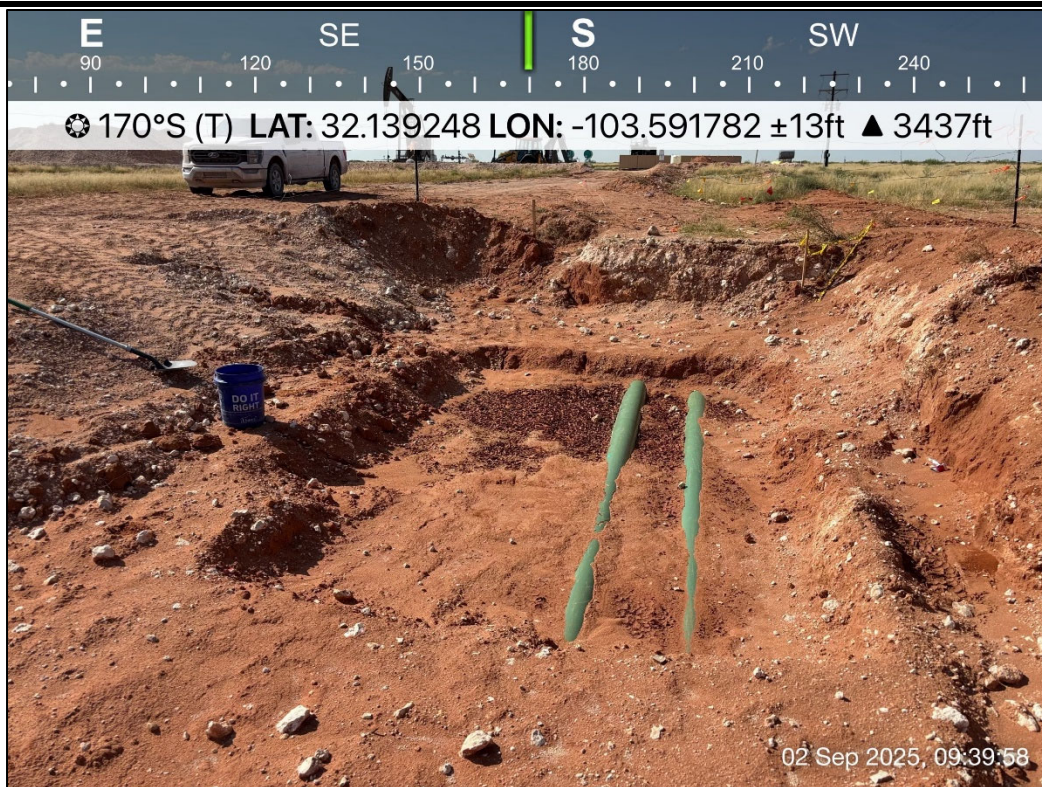
PHOTO 20: Southeastern view of excavation extent. 9/2/2025
