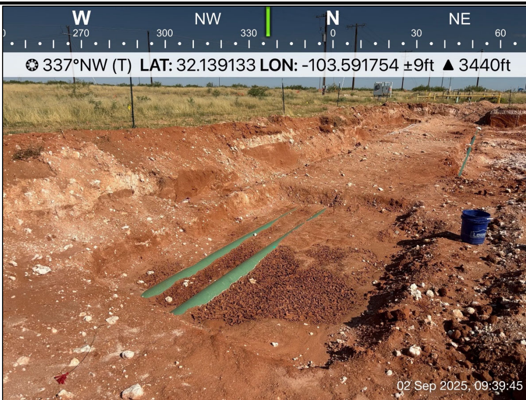
PHOTO 22: Northwestern view of excavation extent. 9/2/2025
