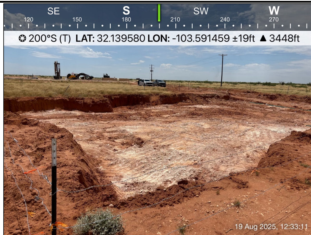
PHOTO 18: Southwestern view of excavation extent. 8/19/2025
