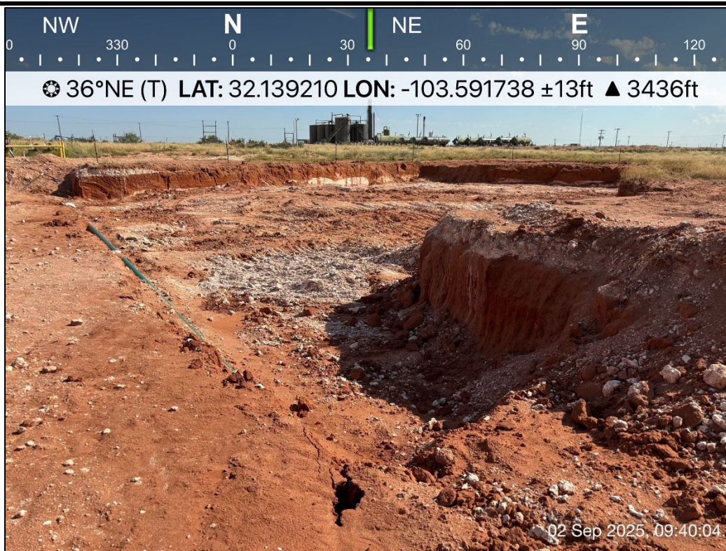
PHOTO 21: Northeastern view of excavation extent. 9/2/2025
