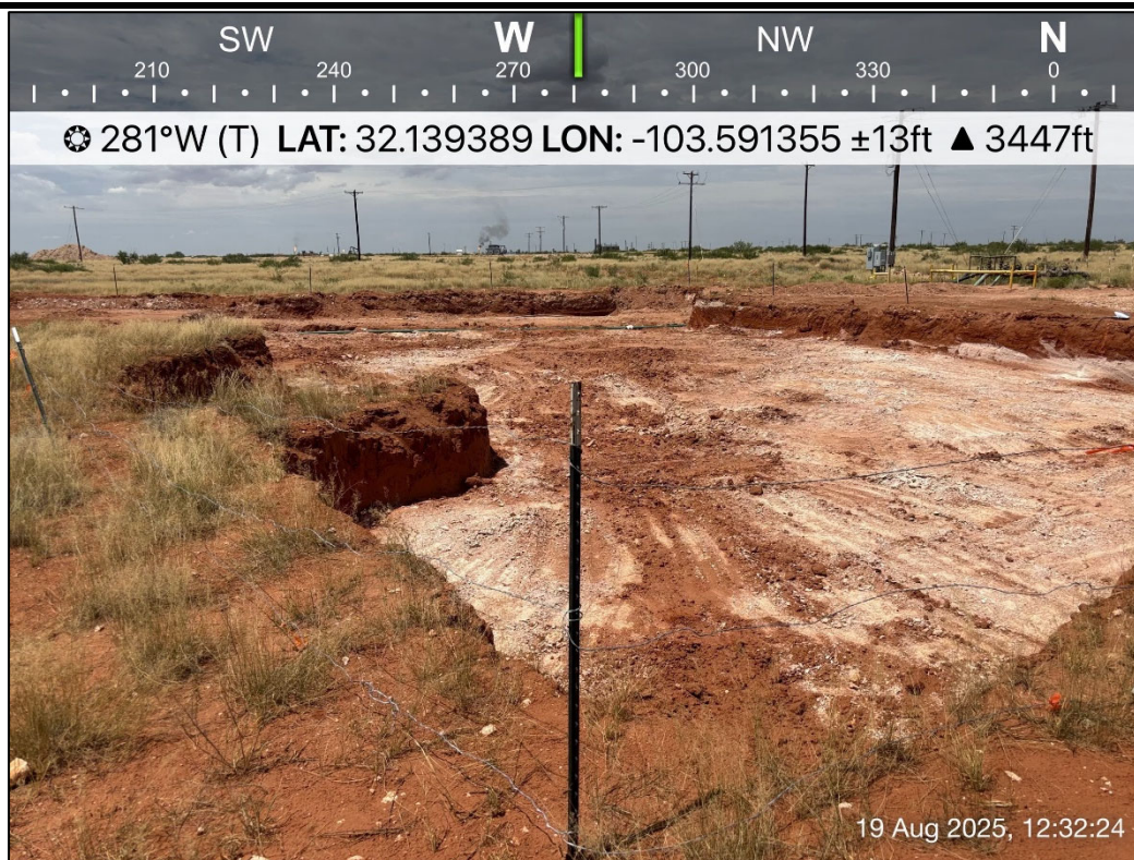
PHOTO 17: Northwestern view of excavation extent. 8/19/2025
