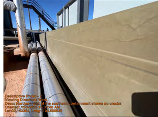
Viewing Direction: West
