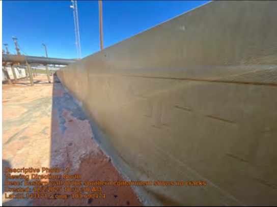
Viewing Direction: North
