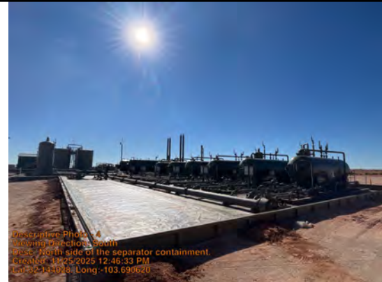
North side of the separator containment.
