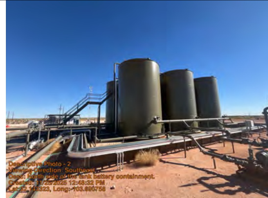
North side of the tank battery containment.
