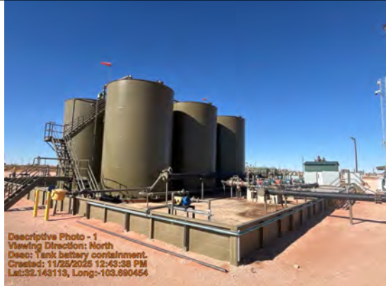
South side of the tank battery containment.
