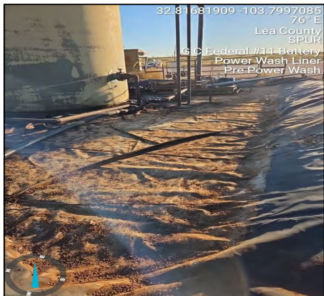
Photograph taken pre- powerwash process facing east.
