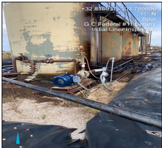
Photo of liner taken during initial liner inspection facing north.
