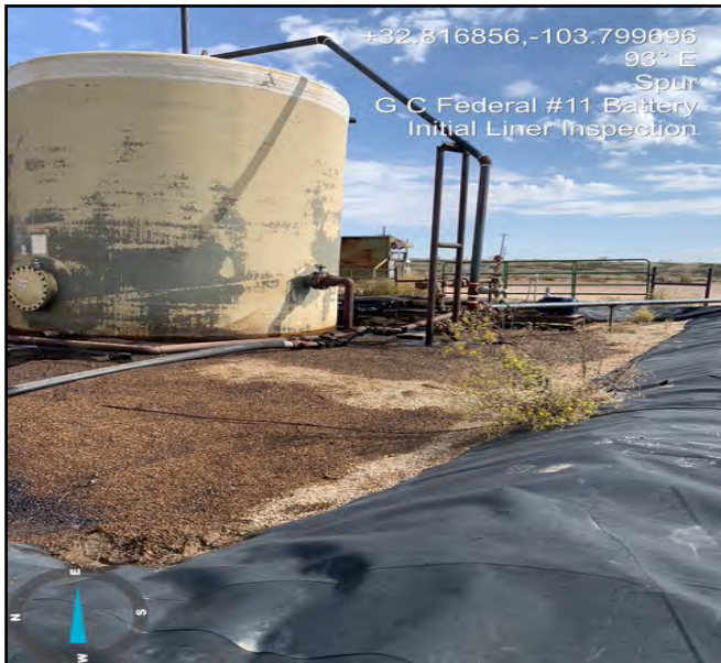
Photo of liner taken during initial liner inspection facing east.
