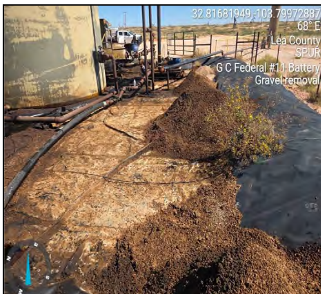
Photograph taken prior to gravel removal, facing east.
