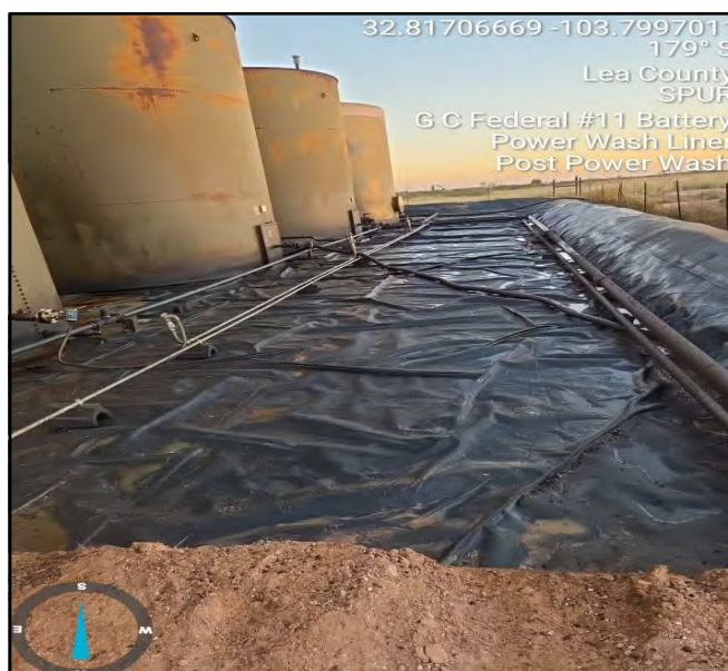
Photo of location taken post power wash facing south.
