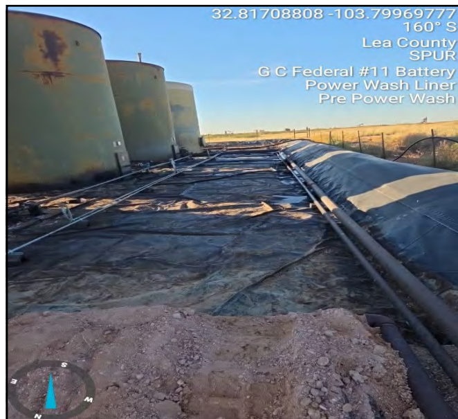
Photograph taken pre- powerwash process facing south.
