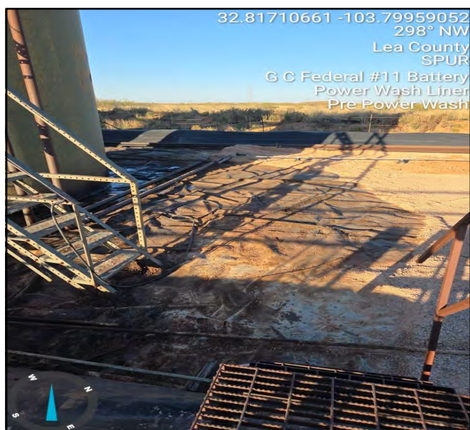
Photograph taken pre- powerwash process facing northwest.
