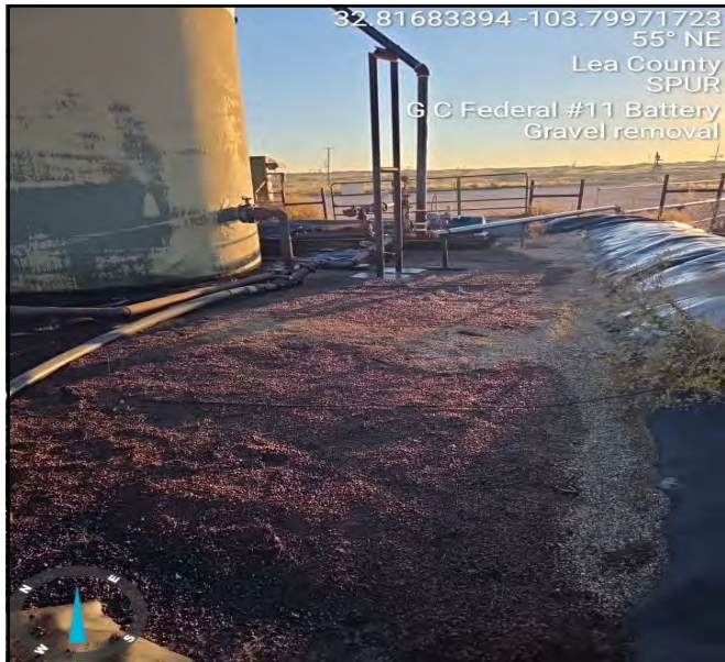
Photograph taken prior to gravel removal, facing northeast.
