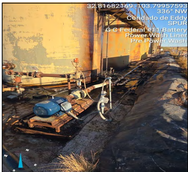
Photograph taken pre- powerwash process facing northwest.
