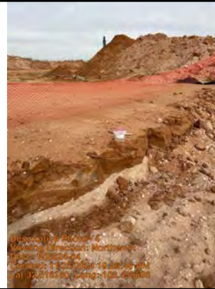
Viewing Direction: Northwest
