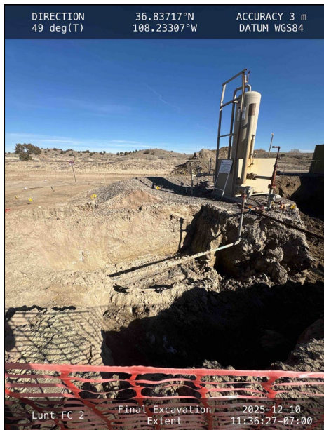
Photograph: 7 Date: 12/10/2025 Description: Final Excavation Extent View: Northeast
