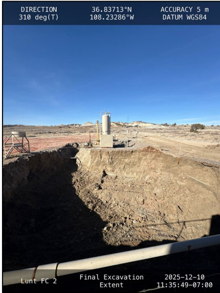
Photograph: 5 Date: 12/10/2025 Description: Final Excavation Extent View: Northwest
