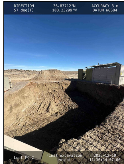
Photograph: 6 Date: 12/10/2025 Description: Final Excavation Extent View: Northeast
