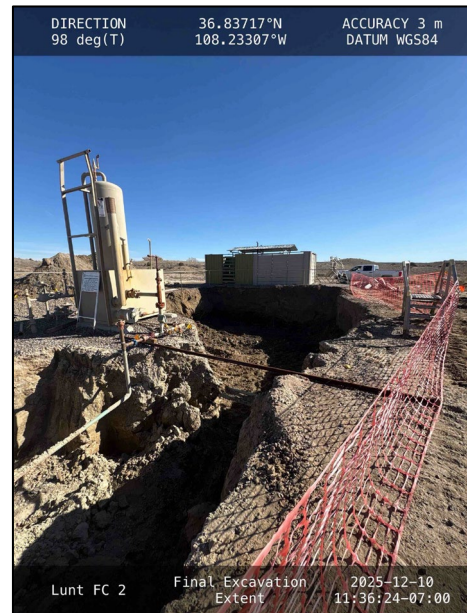
Photograph: 8 Date: 12/10/2025 Description: Final Excavation Extent View: East
