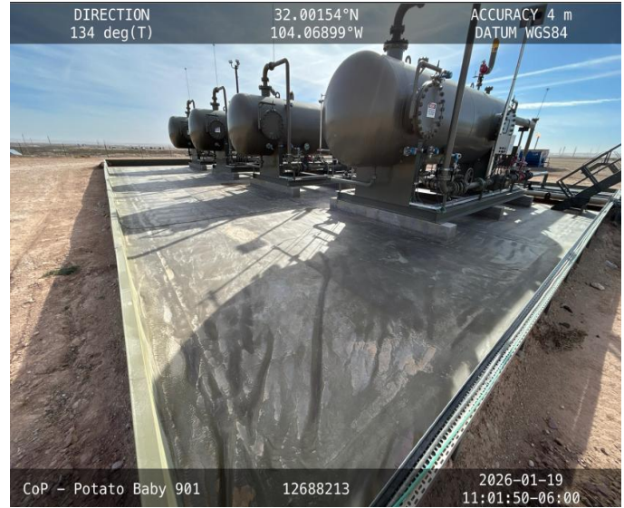
Photo 2 View of northwest corner of containment.
