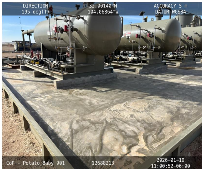
Photo 3 View of northeast corner of containment.
