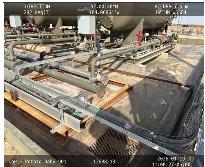
Photo 4 View of southeast corner of containment.
