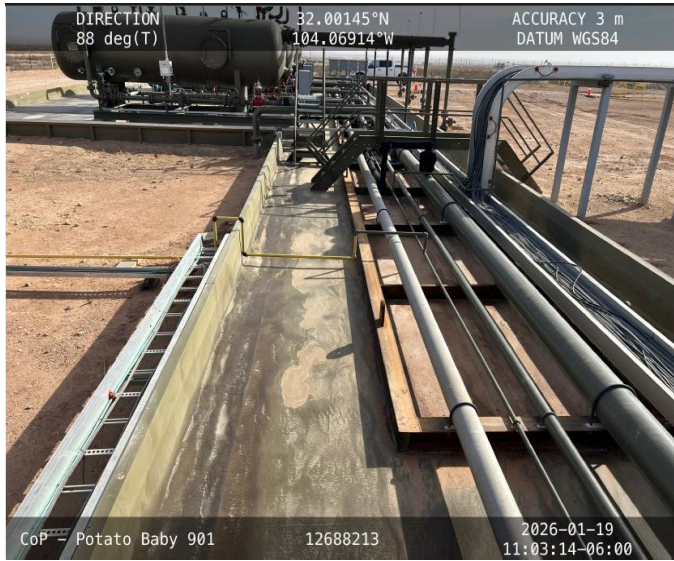
Photo 1 View of containment towards east.
